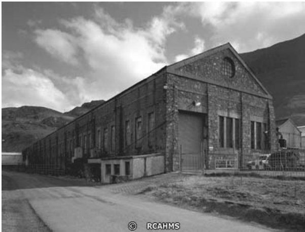
[3 and 4] Kinlochleven Aluminium Works Power House (view from the NW) [Coignet System]
