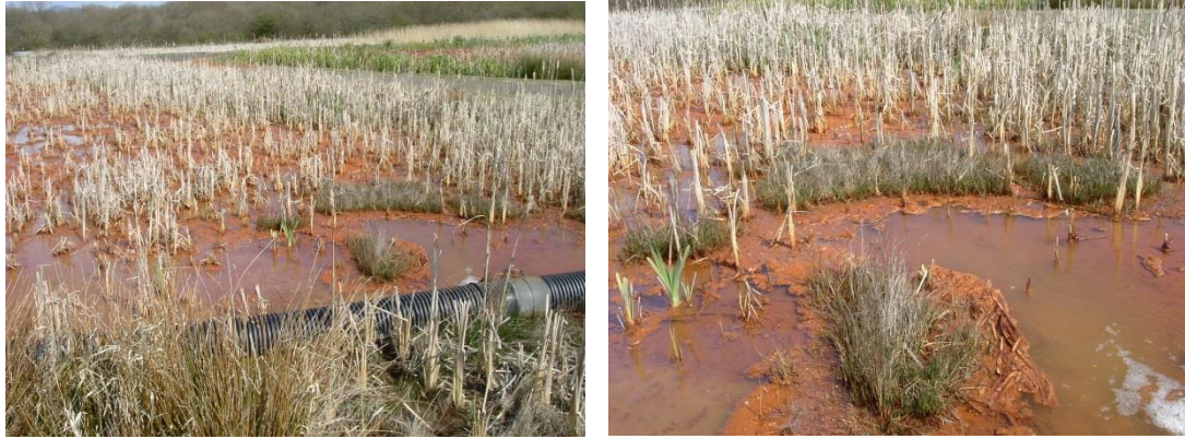
Figure 1.10 The Minto minewater treatment plant wetland in Fife, Scotland (Photographs courtesy of Professor Kate Heal)
