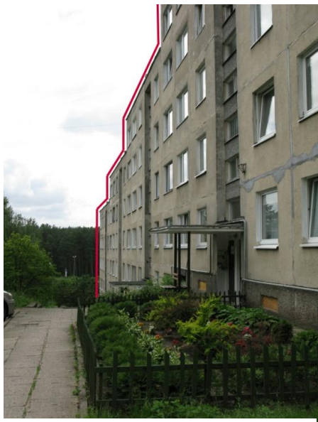
Figure 30. Terraced 5 storey blocks in Lazdynai.
