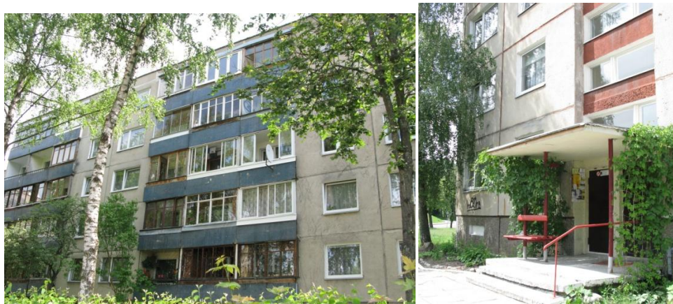
Figure 20. A five storey high block and its entrance, Karoliniškės.
