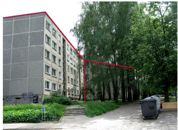
Figure 29. Broken configuration blocks in Lazdynai.
