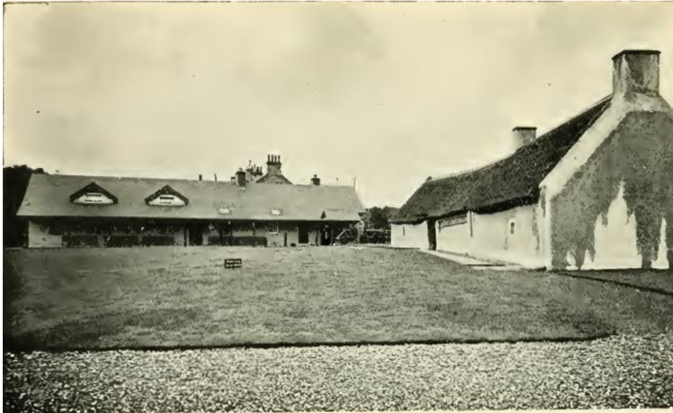
Fig 83 'Cottage, back view, showing new museum buildings' at the left hand side of the picture, photo taken from M'Bain's Burns' Cottage: The Story of the Birthplace of Robert Burns (1904), p. 121, showing the place in restored state
