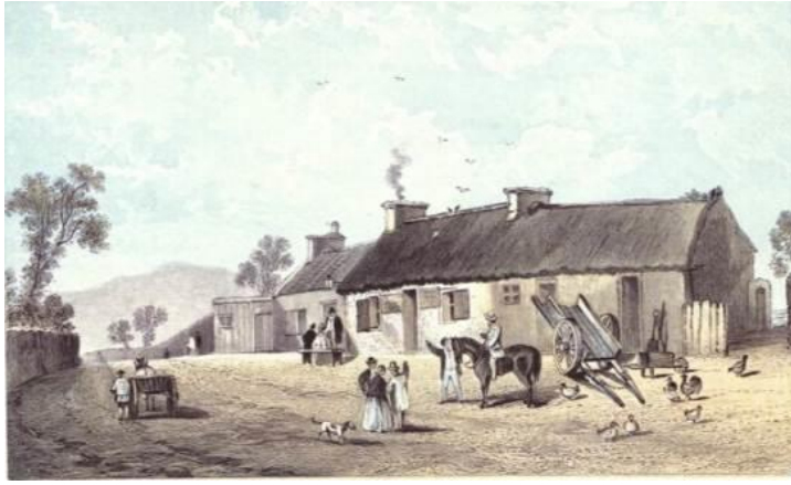
Fig 60 ‘Burns Cottage’, illustration in Nelsons’ Pictorial Guidebooks for Tourists: Ayrshire and Robert Burns , 1870, showing the slated extension to the thatched Cottage at the left hand side
