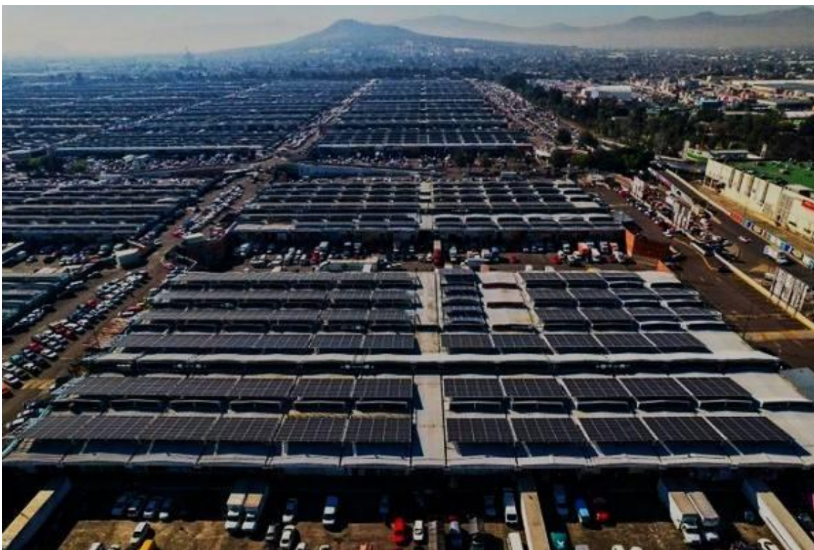
Figure 6 First inner-city (Mexico City) 18MW PV project with intentions to demonstrate Demand-side management by incorporating BESS and EV chargers to a flexible demand system (Rojas, R. 2024)
