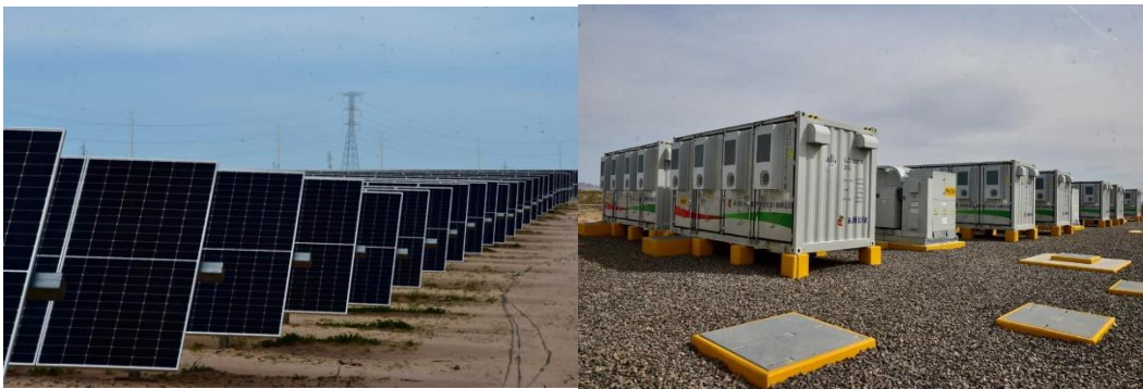
Figure 11 Example of the first phase of Puerto Peñasco PV project (120 MW PV + 24MWh BESS). (García, J., 2023)
