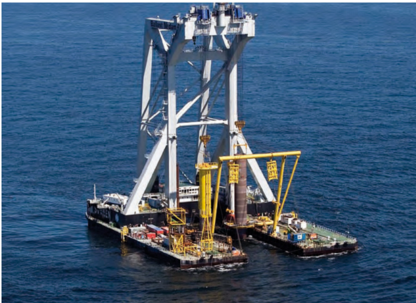
Figure 3.6: Svanen heavy lift vessel installing a monopile [115]
