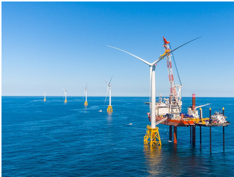
Figure 3.8: Brave Tern WTIV Installing a turbine blade on a jacket foundation[117]
