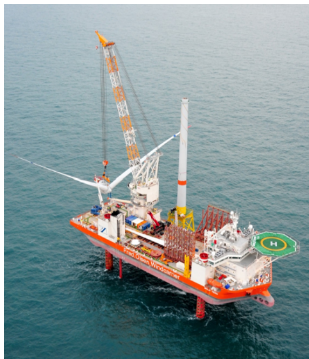
Figure 3.9: Brave Tern WTIV Installing a ‘bunny ear’ rotor assembly[118]
