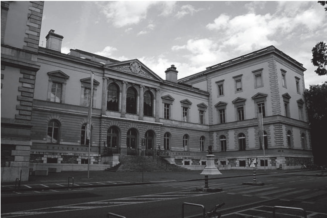
FIGURE 12: BASTIONS BUILDINGS AT THE UNIVERSITY OF GENEVA
