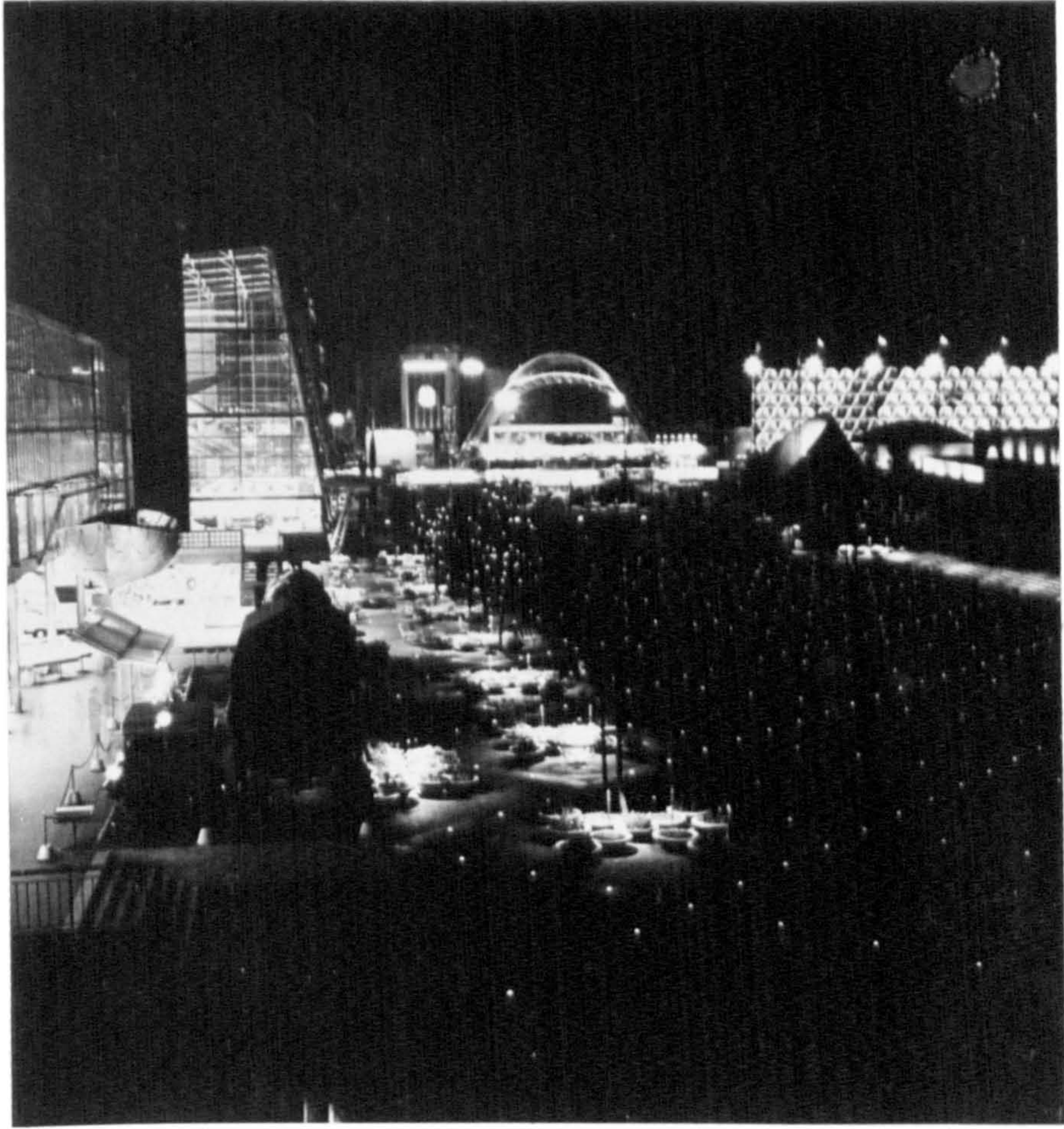
Fig 25 The open concourse of the Upstream Section
