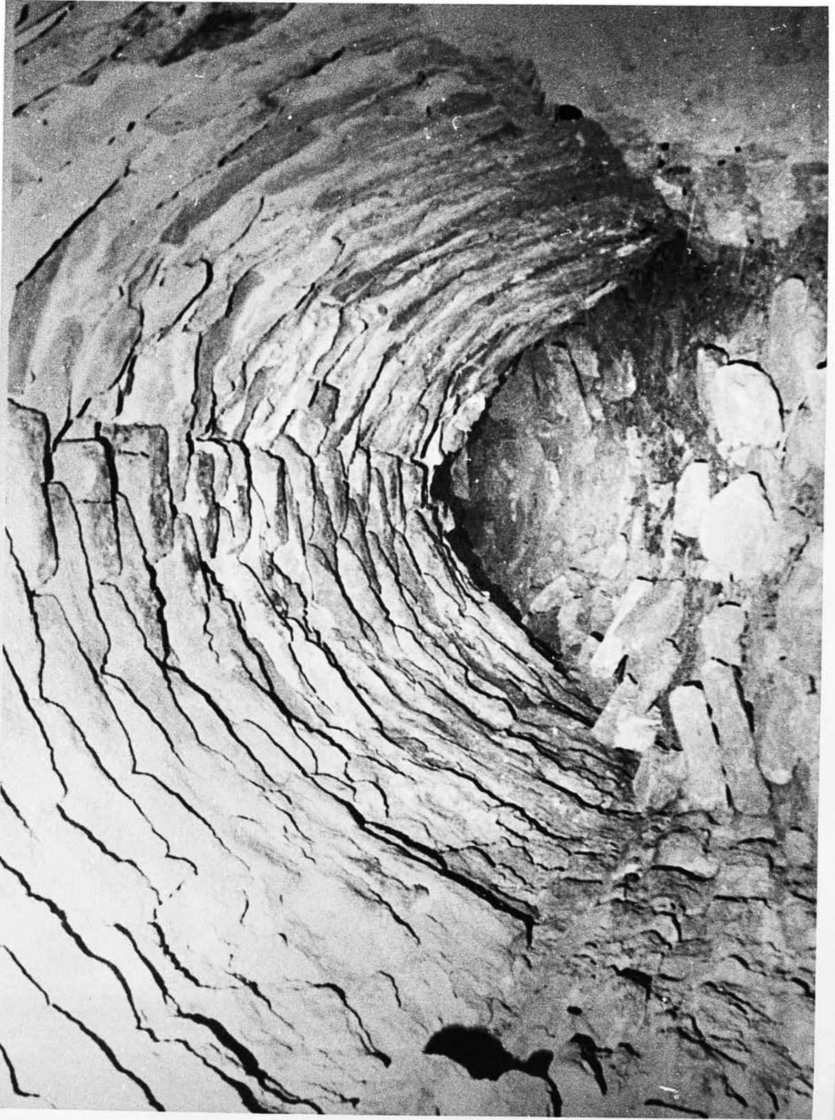
13- Deyr-e Gachin, Iran-Sasanian vault on the corridor leading to the north western tower .
