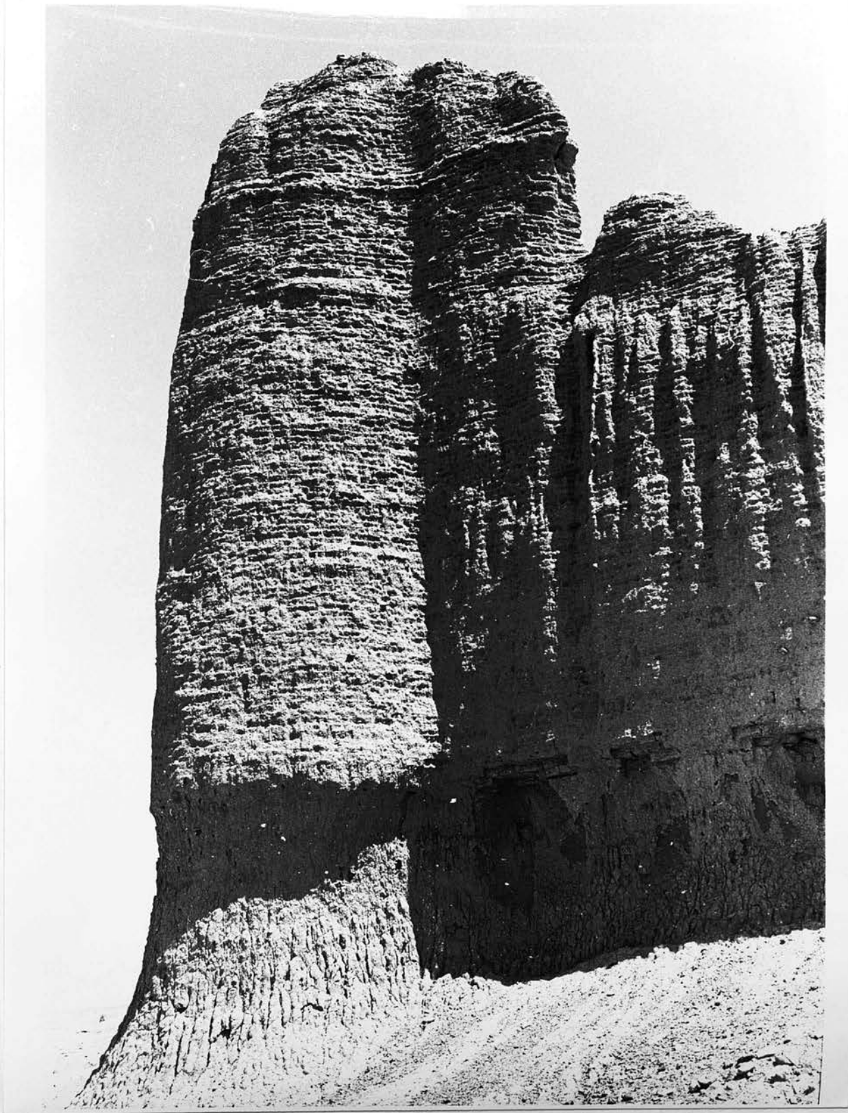
120-Dârzin, Iran-Fort two, north-west tower .
