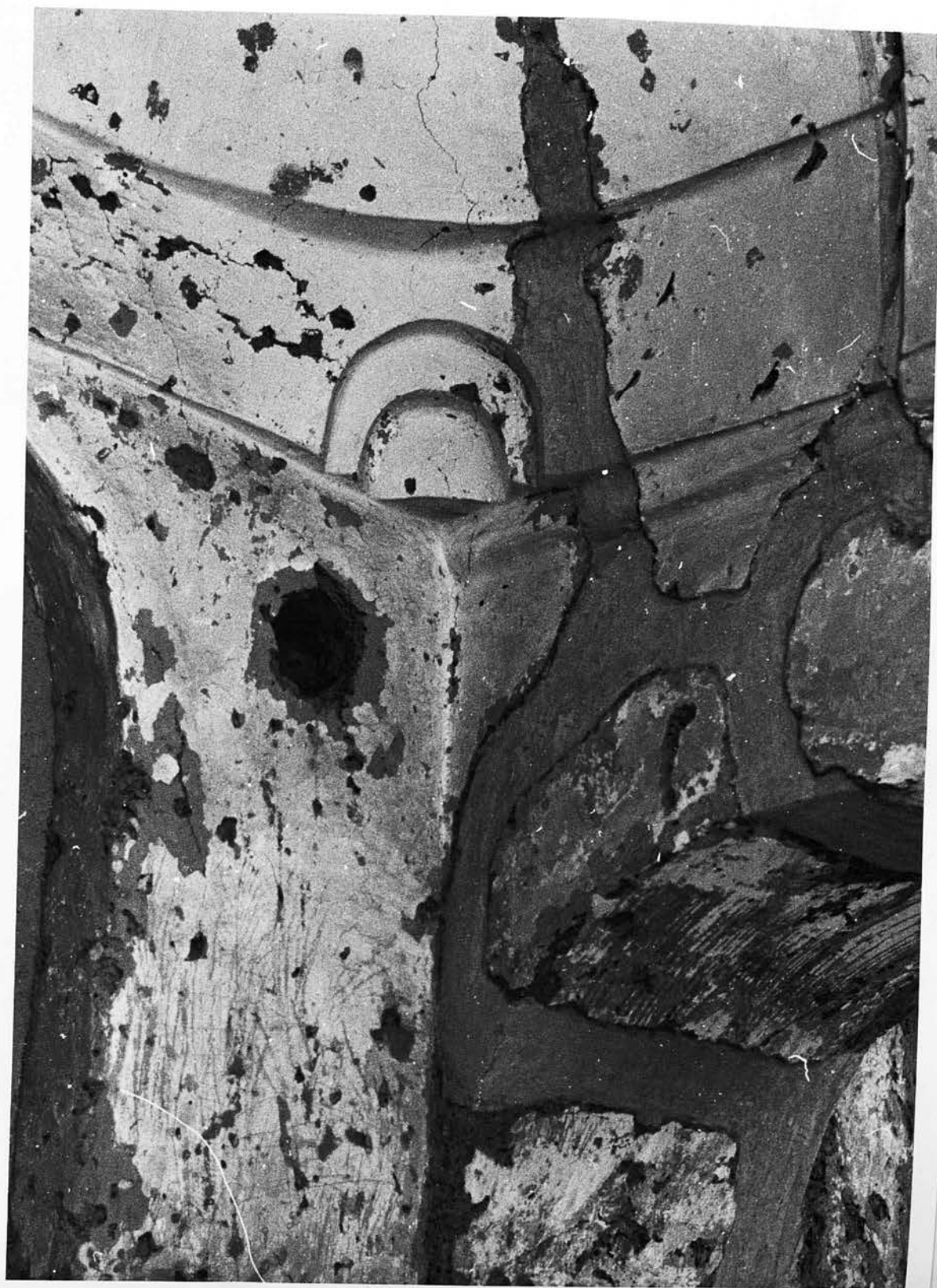
98-Fāhraj, Iran; the jāme' mosque-A sasanian type squinch at the western entrance chamber .
