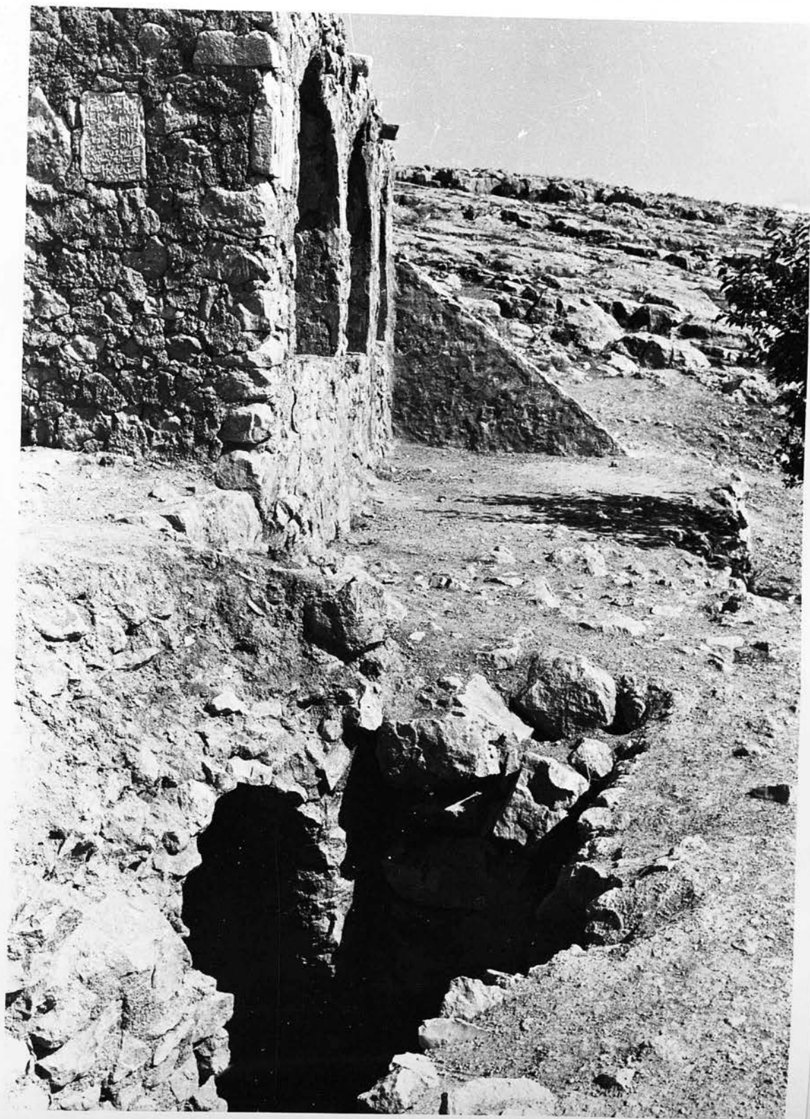
185-Shirāz, Iran-Chāh-e Morteżā 'Ali, part of under ground chambers.
