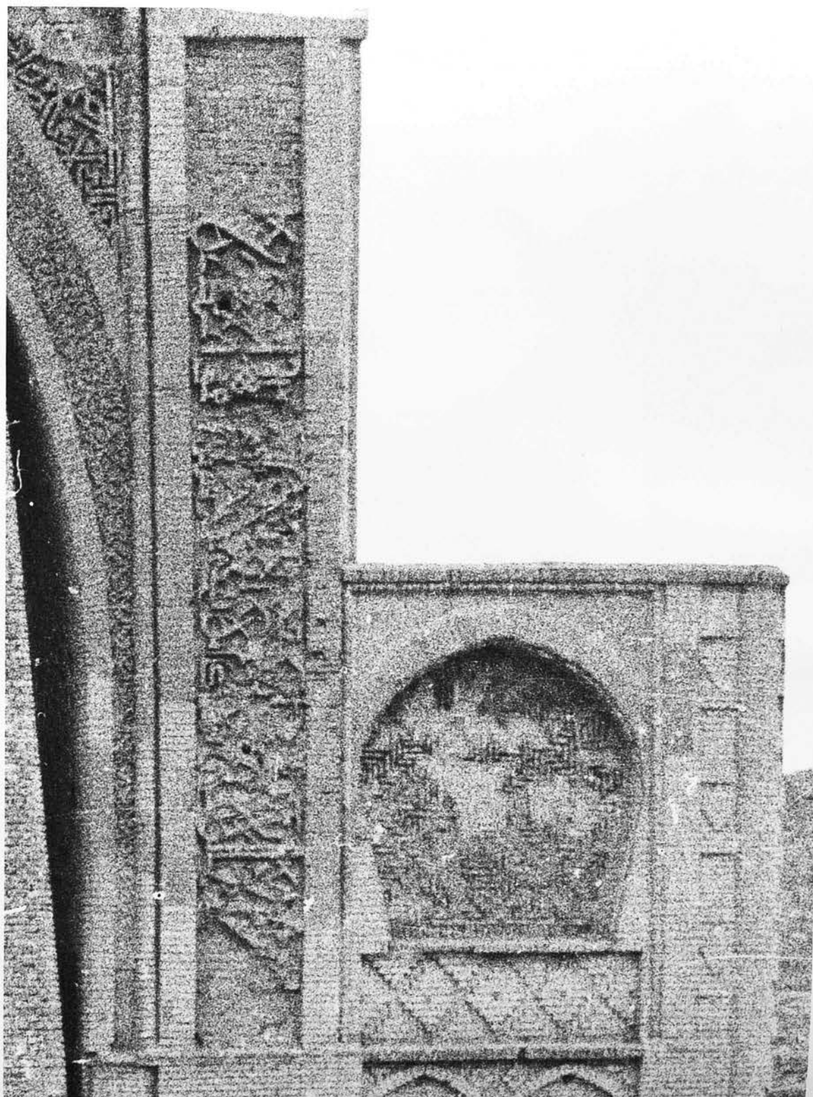
144a-Bost, Afghanistan; The Arch, eastern view (present condition), north wing .
