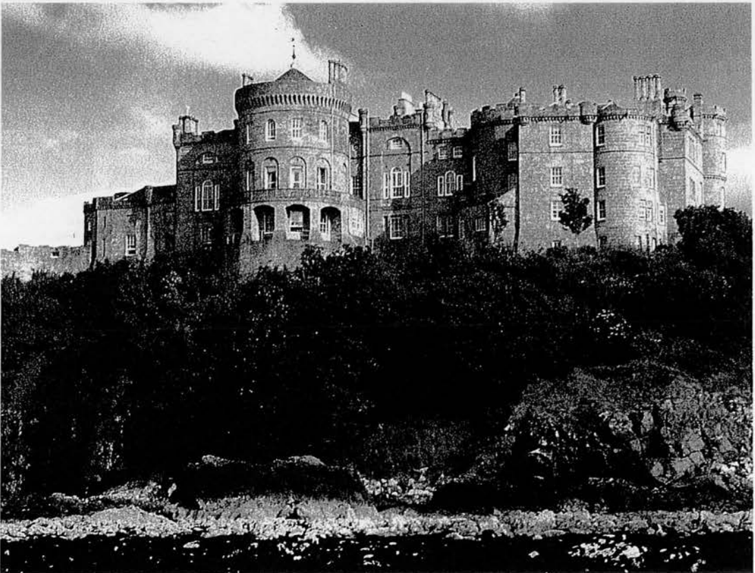
95. Culzean Castle; view of the seaside front.
