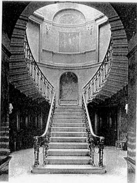
51. Home House, 20 Portman Square; interior view of the stairwell.
