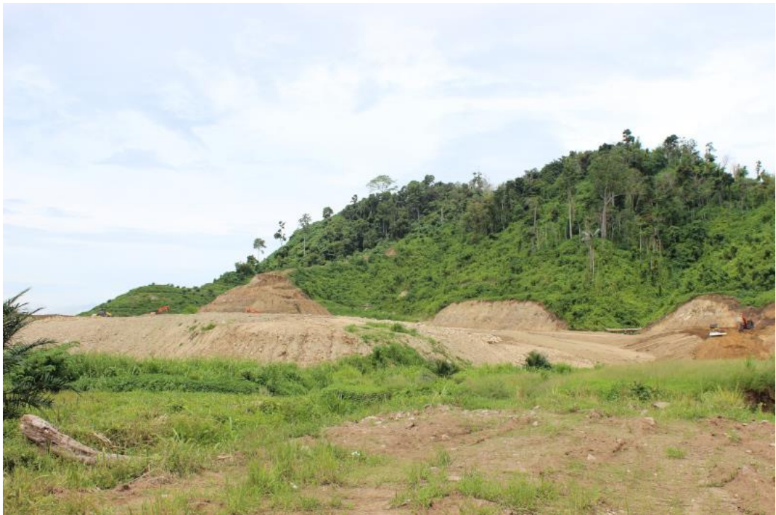
Figure 31 - Bulldozers Clearing the Bush
