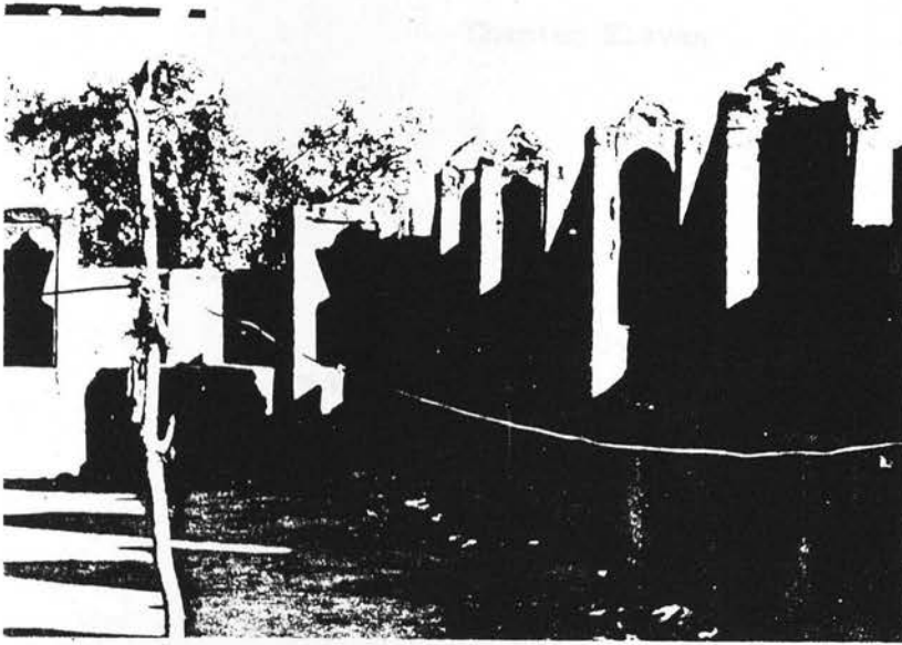
FIGURE 58 Air-catchers, house in Bagdad.
