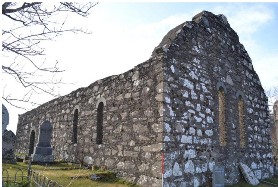
Figure 6.1 (above) – St Columba's Craignish, Argyll; Twin-lancet, unicameral, lateral nave entrance, coursed rubble, fine-dressed sandstone details, limestone-lime; probably mid- 13 th -century; Scale 500mm.
