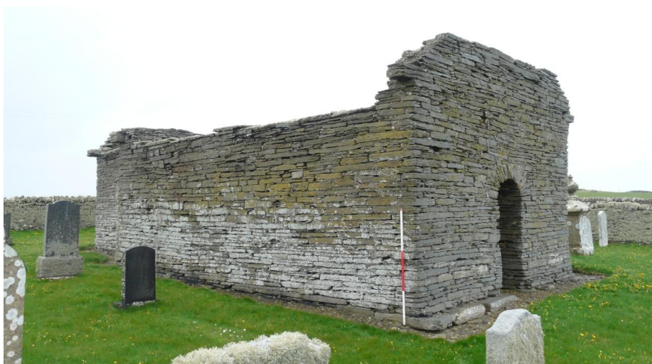
Figure 6.2 (above) – St Mary's Wyre, Orkney; no east window, bicameral, west nave entrance, no fine-dressed sandstone features, biogenic-lime; probably early 12 th -century; Scale 500mm.
