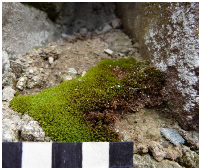
Figure 5.3 (above) – An example of ‘shelly clay’. This medieval wall was previously fully lime-bonded, but the core mortar has almost completely degraded to leave a mixture of silty temper and Type 3 C. edule shell kiln-relicts. St Duthoc’s Chapel, Tain. Scale 10mm; photograph M. Thacker.
