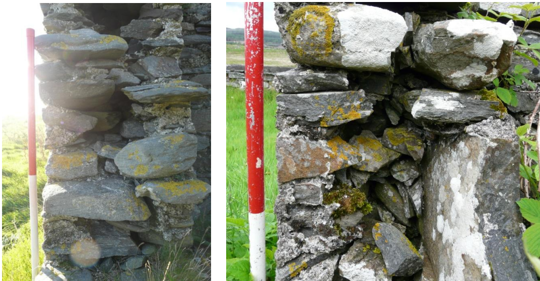
Figures 5.1 & 5.2 (above). Formerly fully lime-bonded, the core mortar in these structures has degraded much faster than the bedding and coating leaving a very voided core which can look like pointed or coated dry-stone. Kilvickeon, Mull and St Ninian's Point, Bute. Scale 500mm; photographs M. Thacker.
