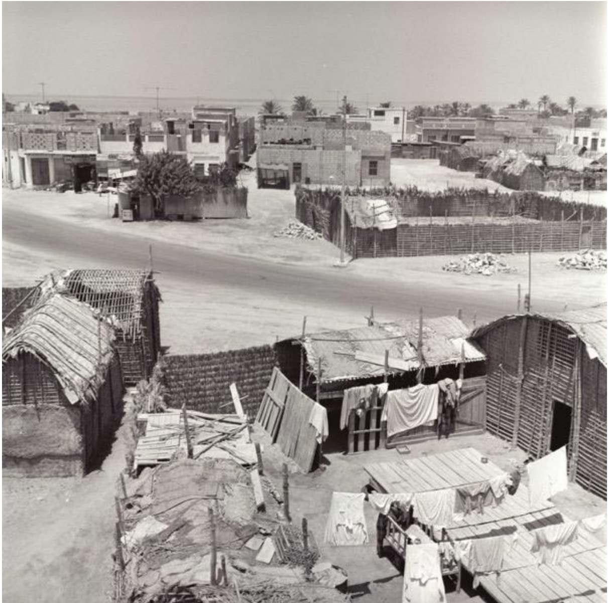
Image 4.1. Before the new town: barasti houses made of palm reeds in Um Al Hasam, circa 1960s. Source: Abdulla Mohammed Al Khan.
