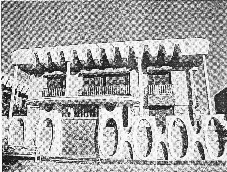
Fig. (7.4) An example of a modern villa in Jeddah during the middle post-oil period. The confused and irrational facade treatment adds yet another cosmetic design approach to Jeddah's eclectic architectural scene.
