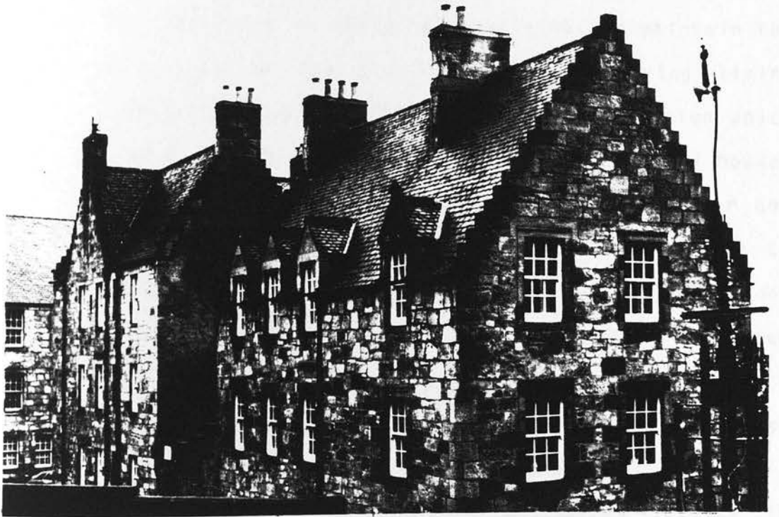
Fig. 6.22. Two views of the three-storey tenement and adjoining two-storey building on Church Wynd, Stirling. Stone from the vernacular buildings which had originally stood on the site was used in their construction. F.C. Mears, 1937.
