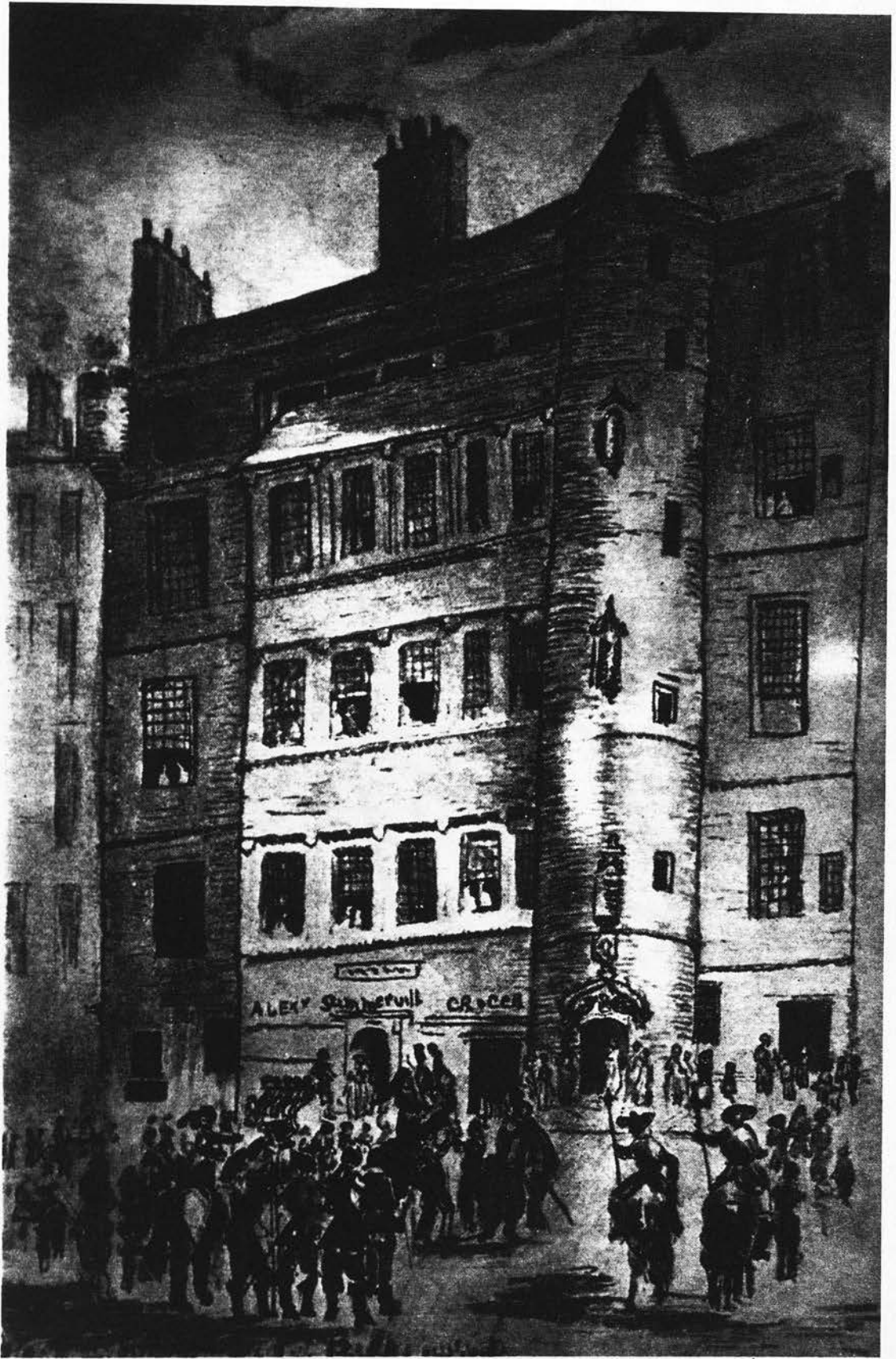
Fig. 5.6. The Black Turnpike. An early Edinburgh tenement. Source: MEARS, F.C. (1929), "The Growth of Edinburgh", in "Edinburgh: 1329-1929", Edinburgh Corporation, Oliver & Boyd, Edinburgh.
