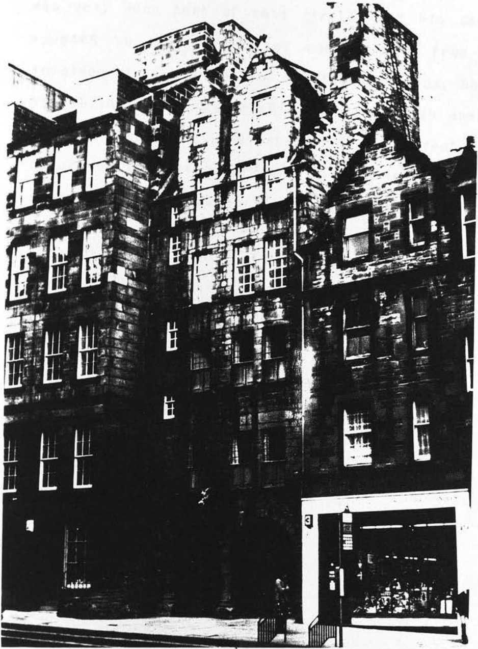
Fig. 6.28. Gladstone's Land, Edinburgh. Restored by Mears for the National Trust for Scotland between 1936 and 1938.
