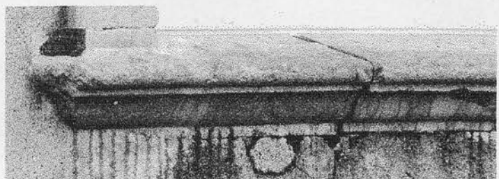
Plate 129 v Beechwood Park, Co. Tipperary
