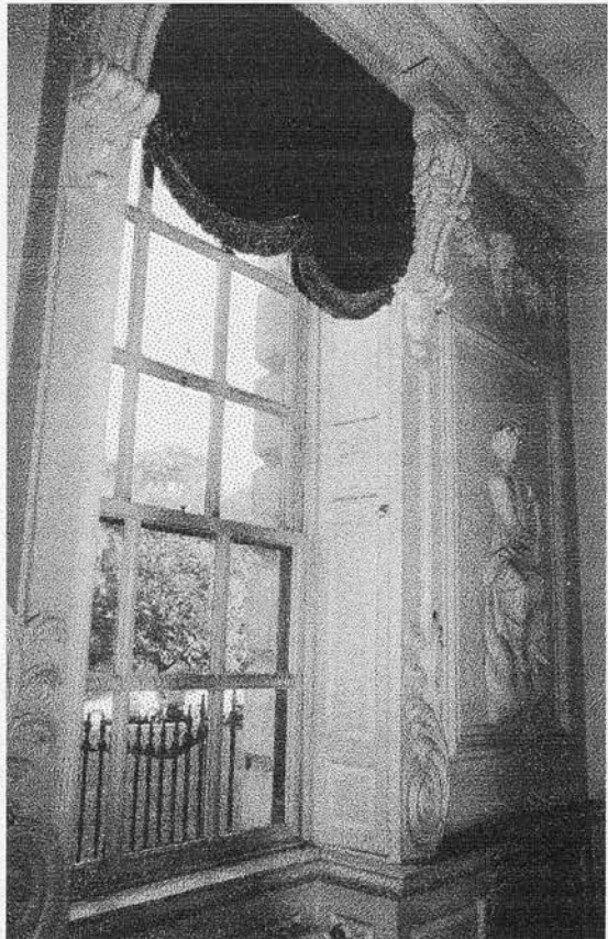
Plate 141 No. 85 St. Stephen's Green, ground floor reception room
