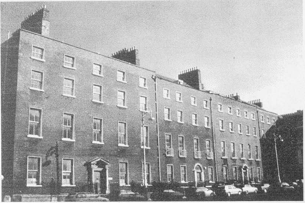
Plate 74 i Nos. 21-4 Upper Merrion Street, Dublin (24 in foreground)
