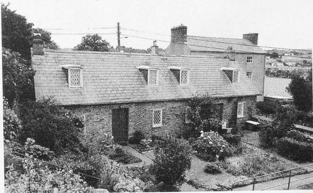
Plate 24 ii Southwell Gifhouses, west range
