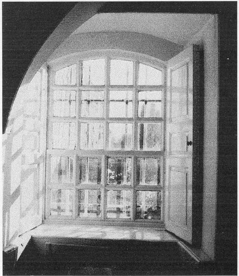
Plate 40 ii Castletown, basement window
