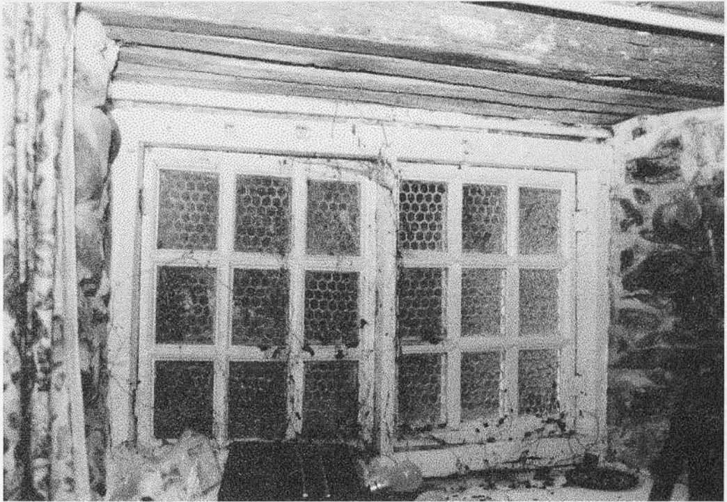
Plate 27 Waringstown, window to south side elevation
