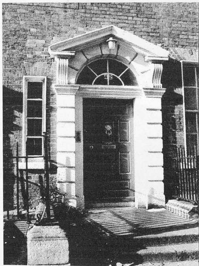
Plate 88 Doorcase with single side-light, Dominic Street, Dublin
