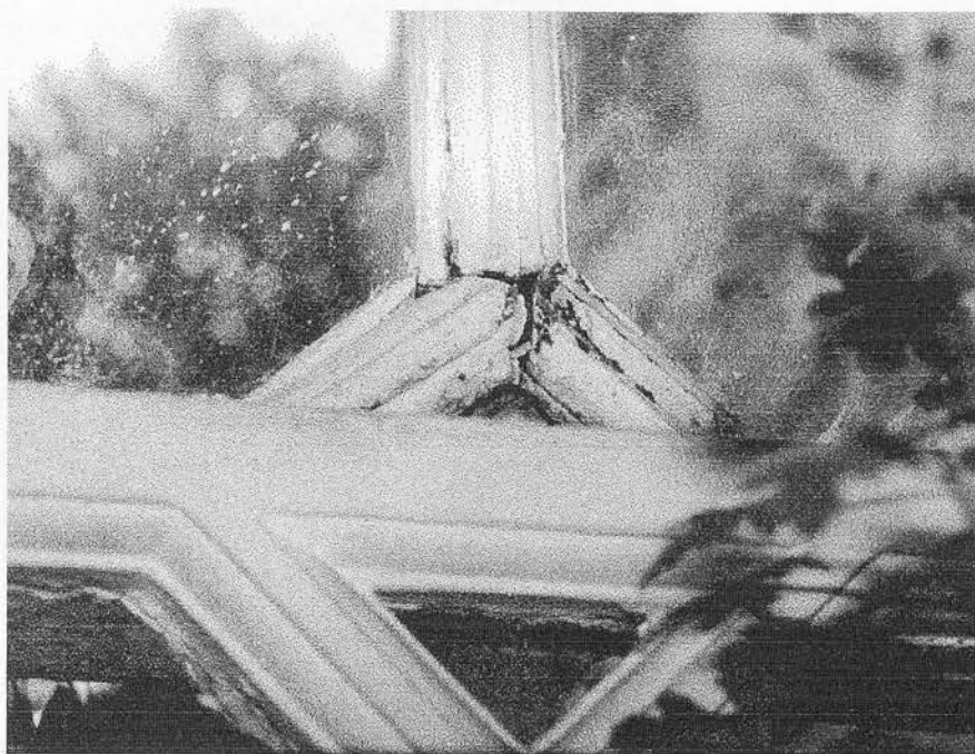
Plate 160 Leixlip Castle, two-part glazing bar
