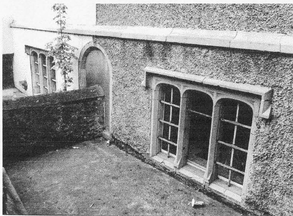
Plate 70 ii Nos. 2-3 Patrick Street, basement windows
