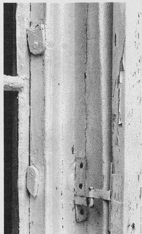
Plate 147 i-iii Quadrant stops: Waringstown and no. 1 Vicar's Hill, Armagh
