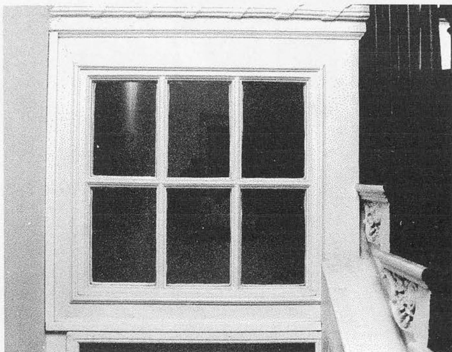
Plate 73 ii Casino, original over-door light at doorway to basement
