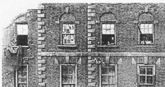
Plate 128 Wards Hill, Dublin, detail of window heads
