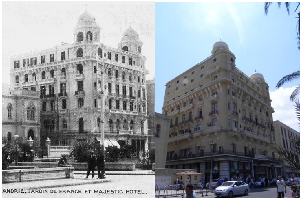
Figure 55. Majestic hotel (privately owned) after demolishing the characteristic domes, adding 2 floors and reconstructing the domes. Source: (left) www.egyptianroyalty.net
