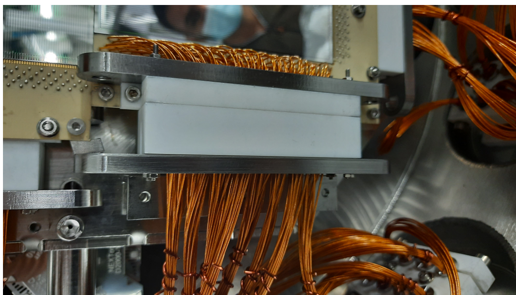
Figure 3.7: Close up view of the cable harness connecting point to the detector carrier. D-connectors are brought together by tightening silver plated screw into the jacking plate of the detector carrier.
