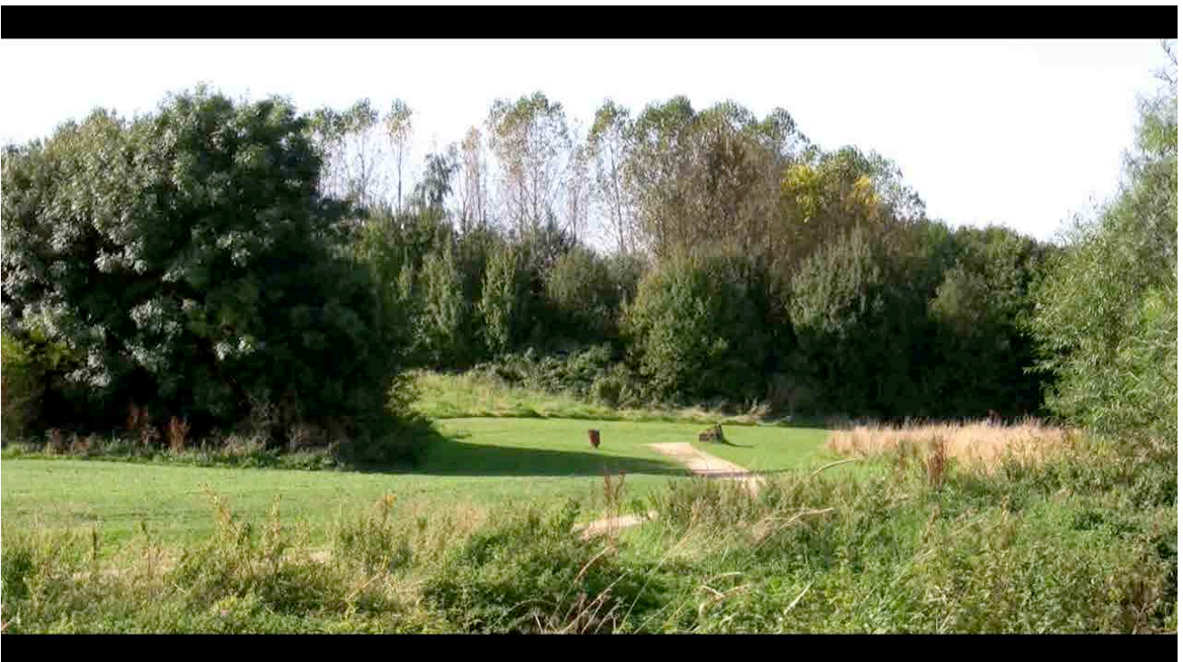
Figure 9.34 The 'Keepsafe' post-restoration from the north bank looking south. Trees have been planted to screen industrial buildings (September, 2009).
