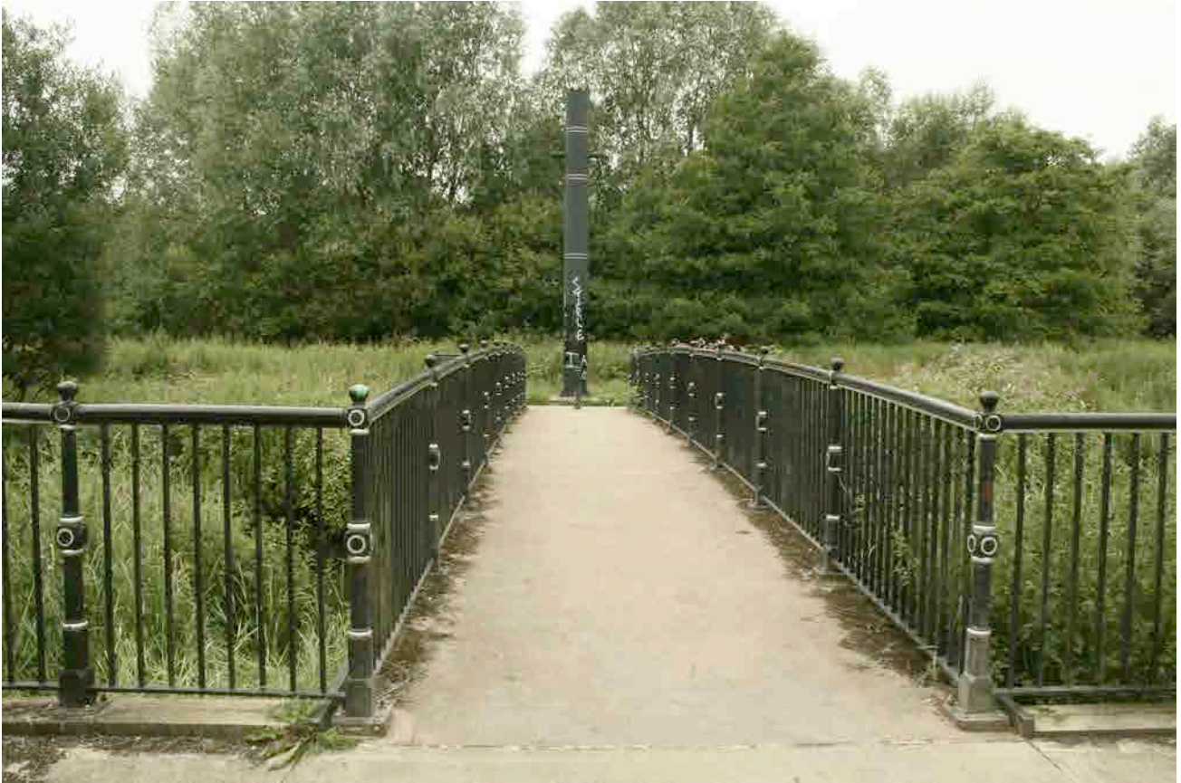
Figure 9.29 The Locomotive Footbridge, with a steam train funnel on the north bank of the Skerne (July, 2009).
