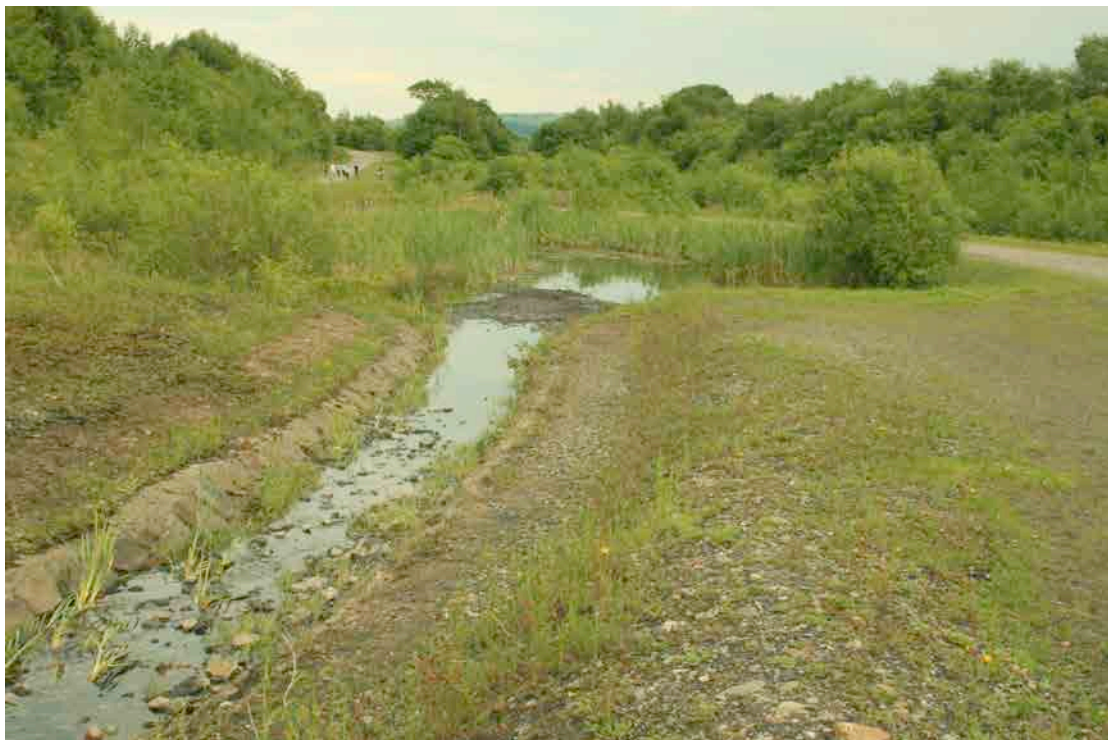
Figure 15.4 A drainage channel terminating at a settling pond. Note the accumulated coal where the channel terminates (June 2010).
