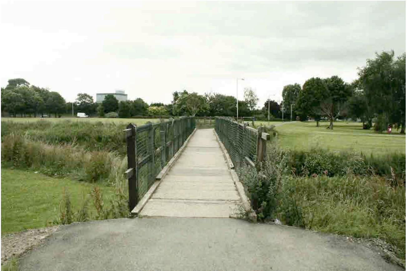
Figure 9.35 Hutton Avenue Footbridge (July, 2009).
