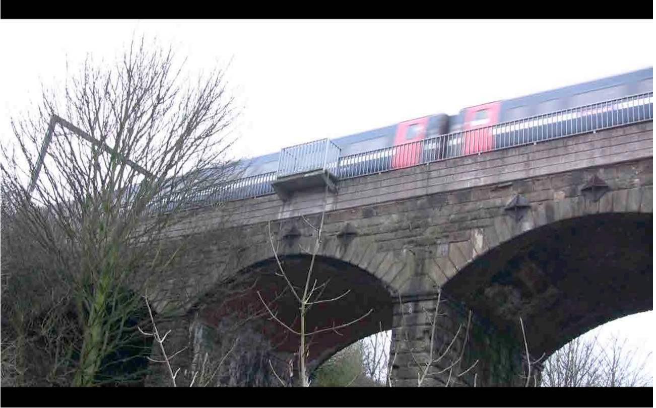
Figure 9.24 Train crossing the Five Arches Bridge (February, 2010).
