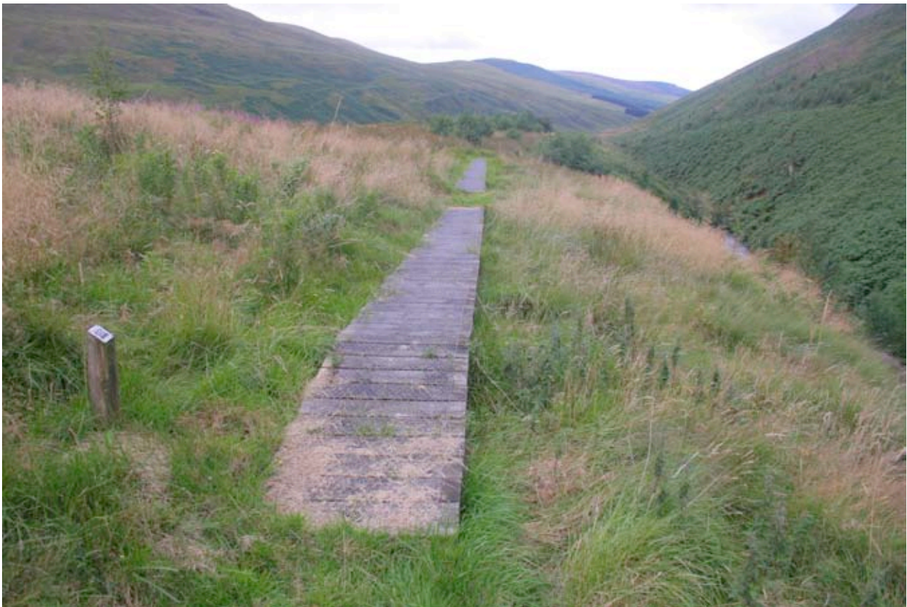
Figure 11.8 Section of boardwalk (August, 2009).
