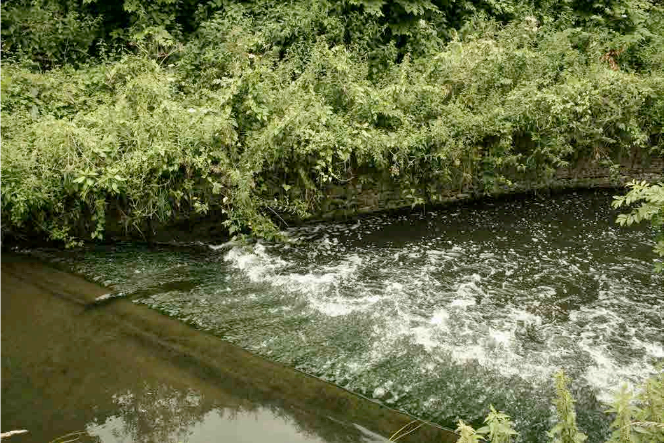
Figure 9.23 Installed 'fish-friendly' weir (July, 2009).
