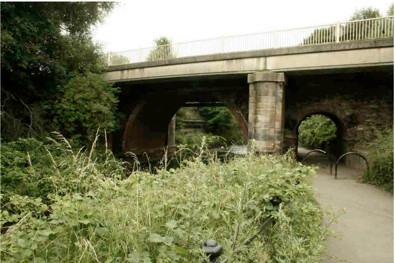
Figure 9.26 Approaching Albert Road Bridge (July, 2009).
