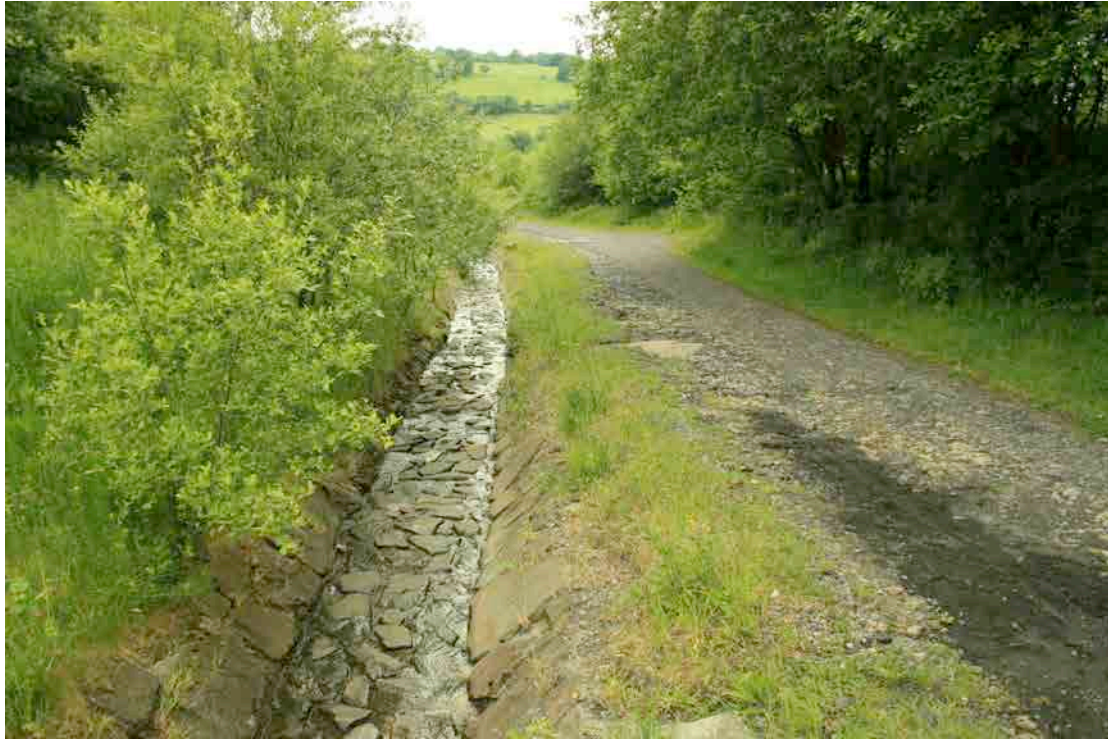
Figure 15.3 Drainage channel running adjacent to footpath (June 2010).
