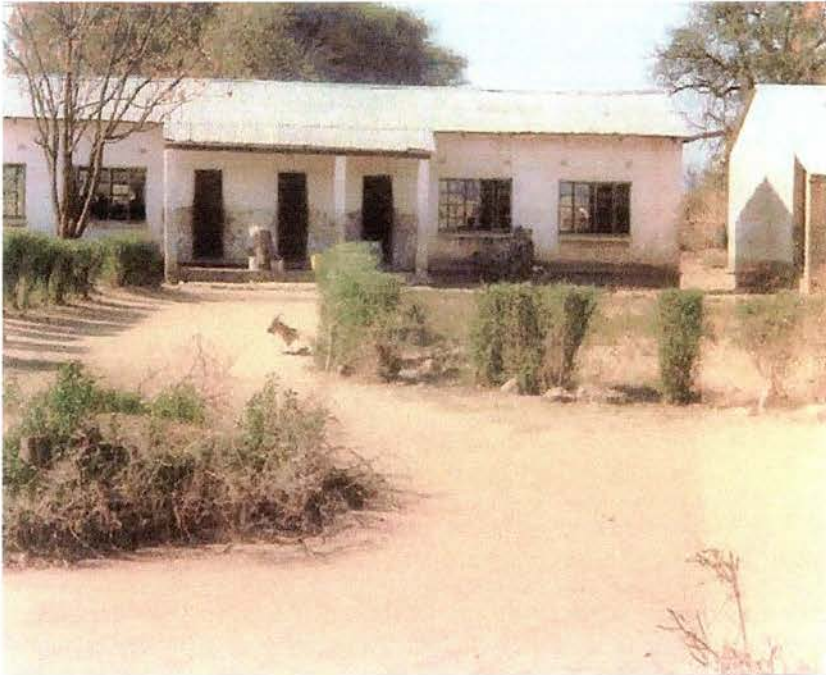
Figure 6.5: An old classroom block
