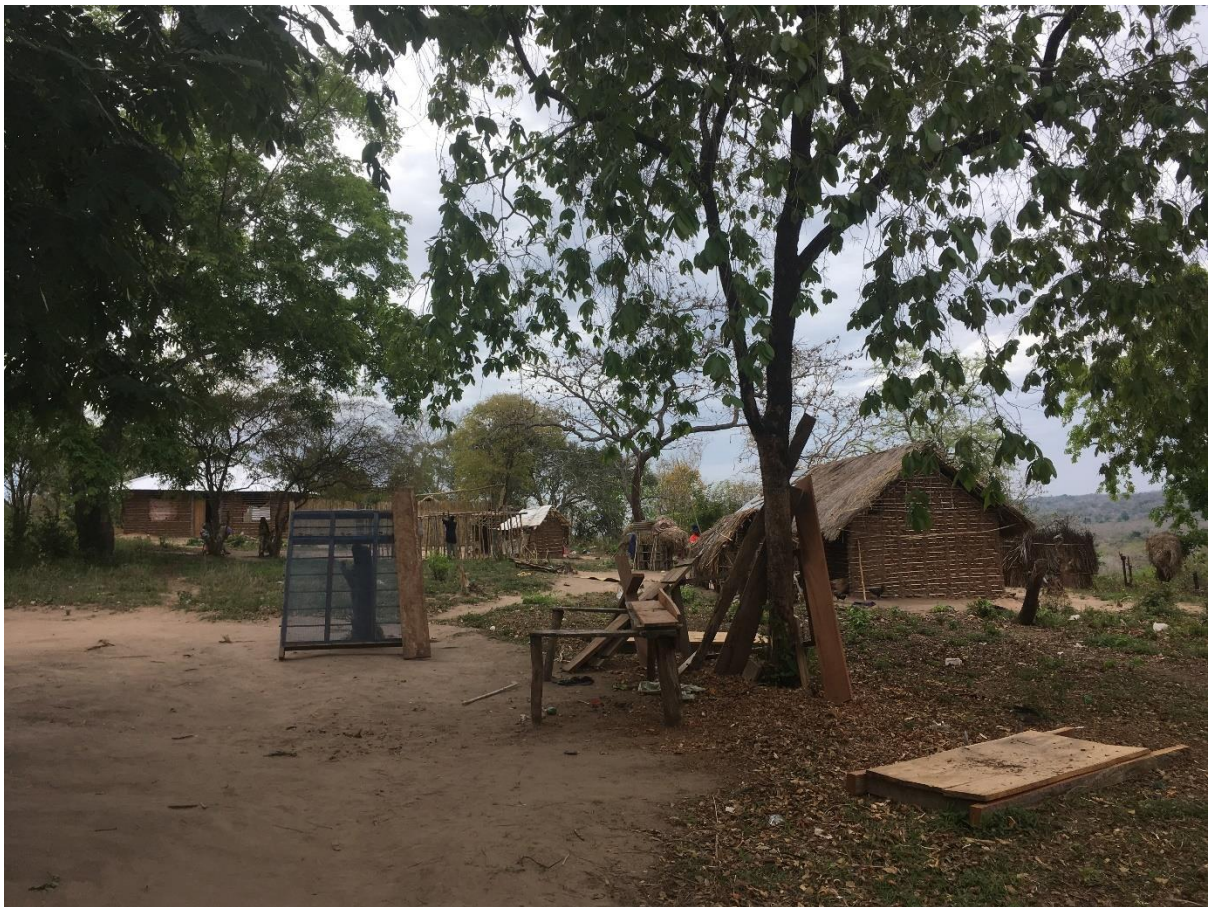
Home being built in Kikole village, Kilwa District, Tanzania (Ellie Wood, 2018).
