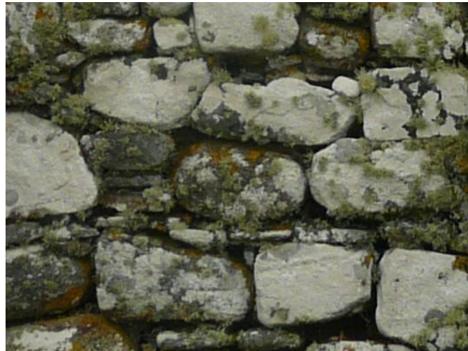
Figure 21 (above) – Caibéal Dhiarmaid , Howmore. Internal east wall.
