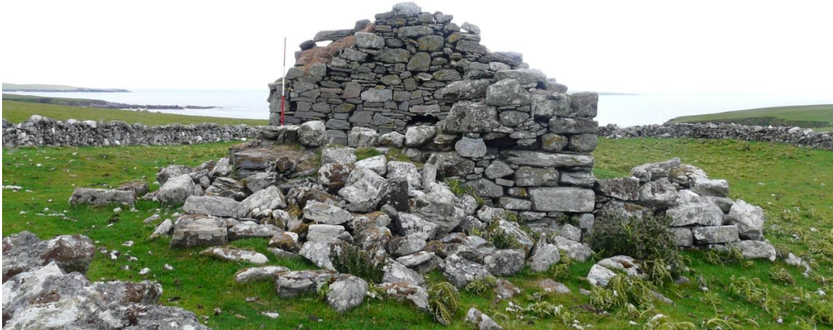
Figure 8 (above) – Uyea chapel and western burial aisle from the west. Scale 500mm; photograph Mark Thacker.
