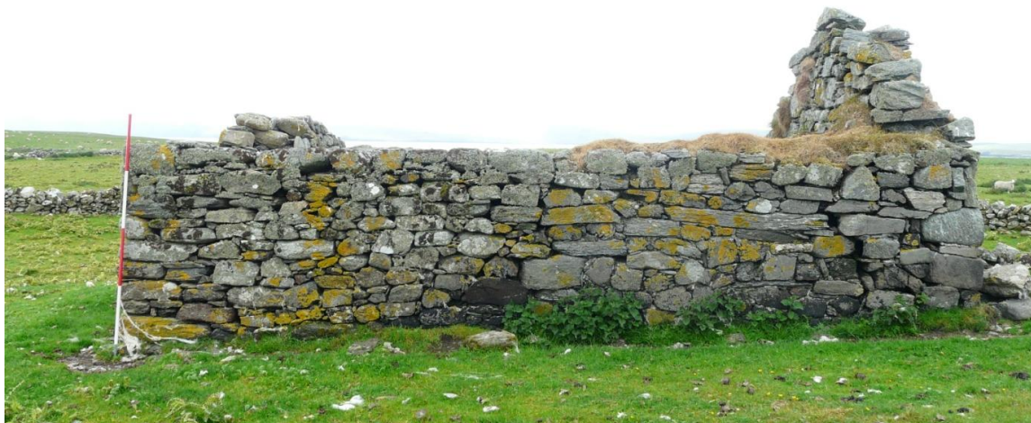
Figure 7 (above) – External face of North wall of Uyea chapel nave. N.B. clear phase change half way along the wall. Scale 500mm; photograph Mark Thacker.
