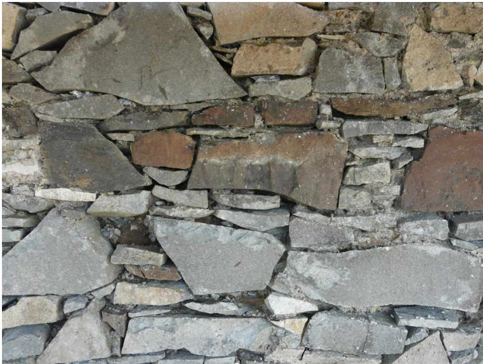
Figure 9 (above) – Dolerite masonry of the external west face of the primary curtain wall. No scale; photograph Mark Thacker.
