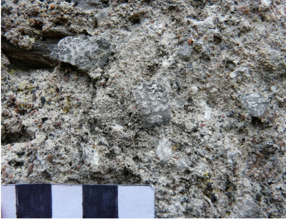
Figure 14 (above) – External face of nunnery west cloister wall; Mortar 1a. Note Type 3-4 heated C. Edule shell relicts. Scale 10mm; photograph Mark Thacker.
