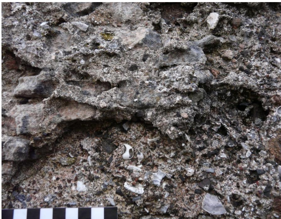
Figure 24 (above) – Mortar phasing and re-coating of the south tower. Scale 10mm; photograph Mark Thacker.
