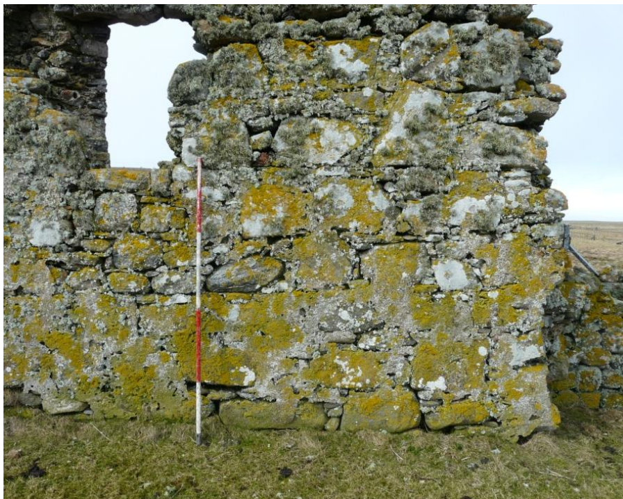
Figure 7 (above) – External face of east wall of Teampull Mòr Howmore. Note formal course lines. Scale 500mm; photograph Mark Thacker.
