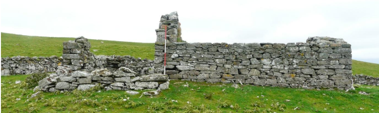
Figure 9 (above) – Uyea chapel and western burial aisle from the south. Scale 500mm; photograph Mark Thacker.
