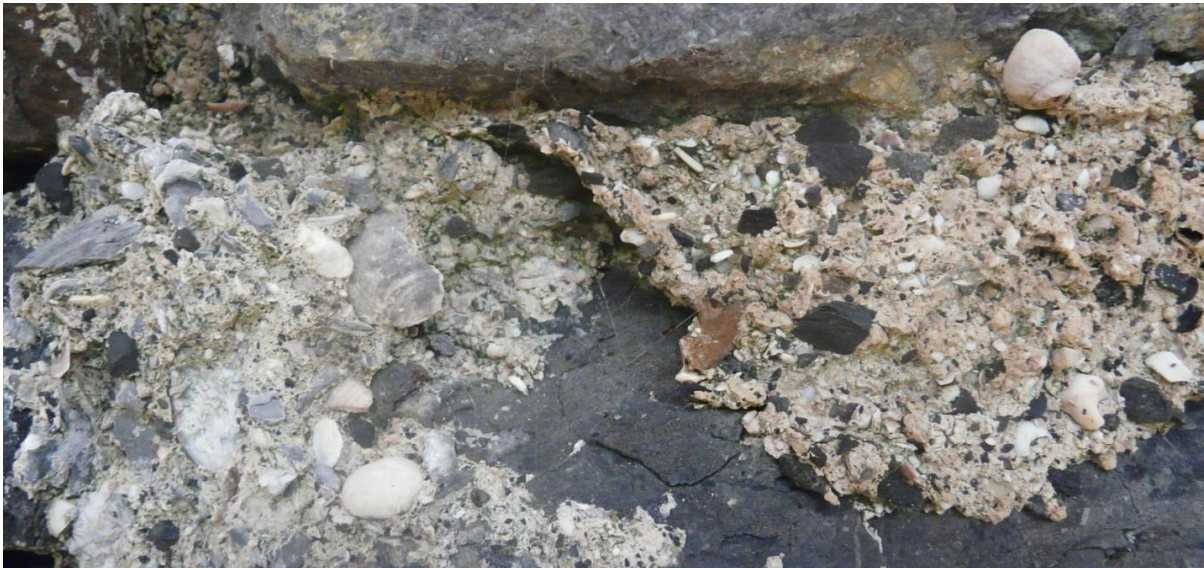
Figure 15 (above) - Mortar 6 (to the right) overlying Mortar 2 (to the left); North range, external face of south wall. Field of view 200mm; photograph Mark Thacker.
