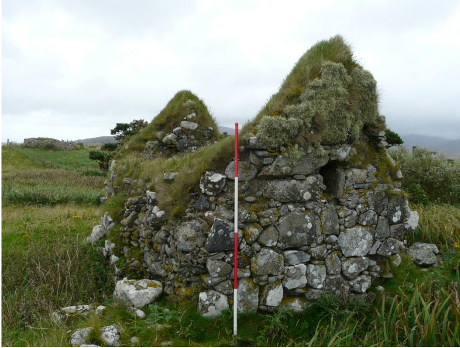
Figure 18 (above) – Caibéal Dubhgail from the north-west. Scale 500mm; photograph Mark Thacker.
