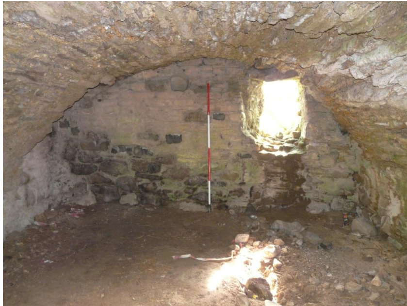
Figure 12 (above) – South tower ground-floor vault looking south-east. Scale 500mm; photograph Mark Thacker.
