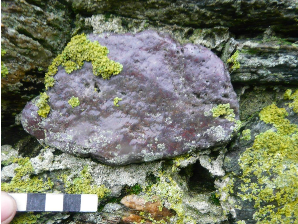
Figure 18 (above) – Uyea chapel nave, internal face of west wall. Vitrified possible kiln lining stone reused in phase 1 masonry. Scale 10mm; photograph Mark Thacker
