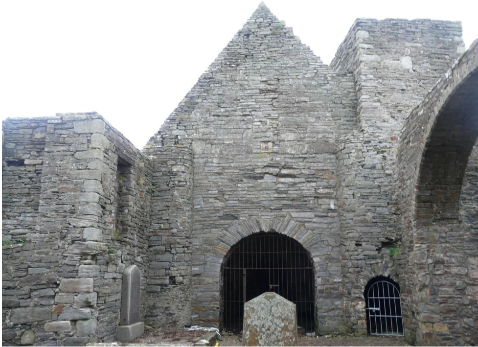
Figure 10 (above) – East nave wall showing primary chancel arch, primary upper chancel doorway (with keyhole stone in blocking), secondary side altar blocking in lower drum to the left of chancel arch, primary tower entrance to the right, and surviving late medieval upper tower. No scale; photograph Mark Thacker.
