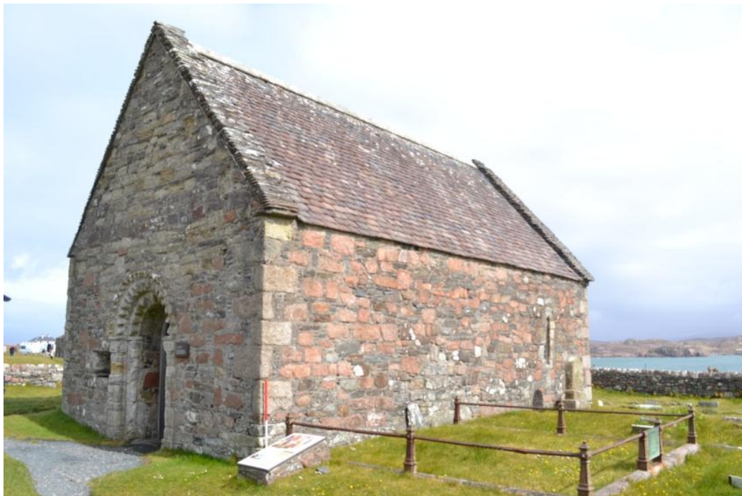
Figure 7 (above) – St Orans chapel from the south-west. Scale 500mm; photograph Mark Thacker
