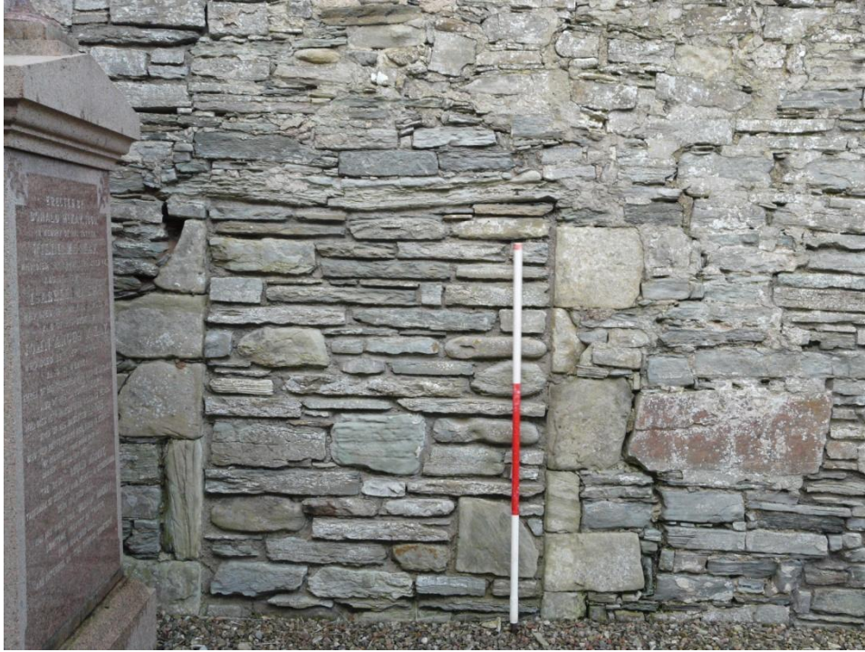
Figure 24 (above) – Internal face of north-west nave doorway. Scale 500mm; photograph Mark Thacker.
