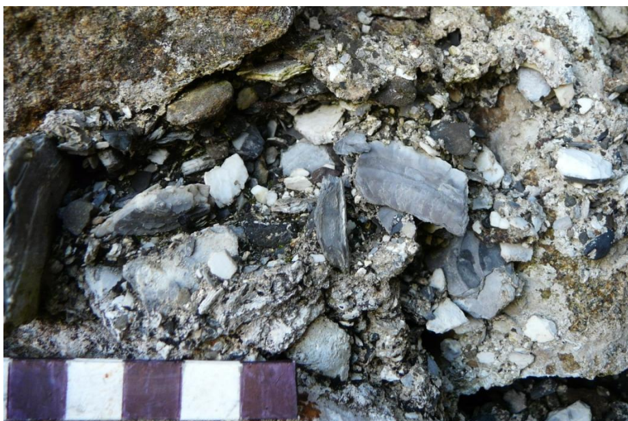
Figure 25 (above) - Mortar 1a in the core of the south-west enclosure wall. Scale 10mm; photograph Mark Thacker.
