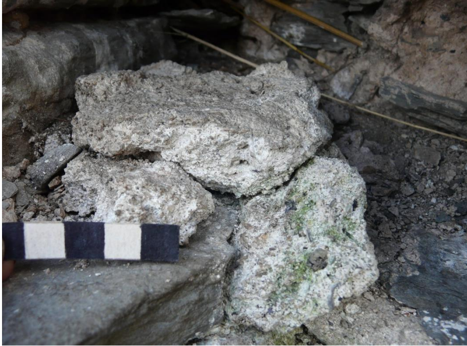
Figure 22 (above) – Mortar 2; deep bed and core context; External face of east chancel secondary window. Scale 10mm; photograph Mark Thacker.
