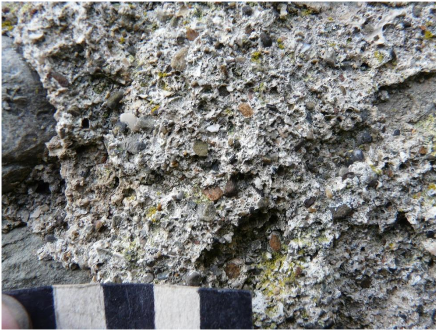
Figure 36 (above) - South aisle; external face of east wall; Mortar 4 slaister. Scale 10mm; photograph Mark Thacker.
