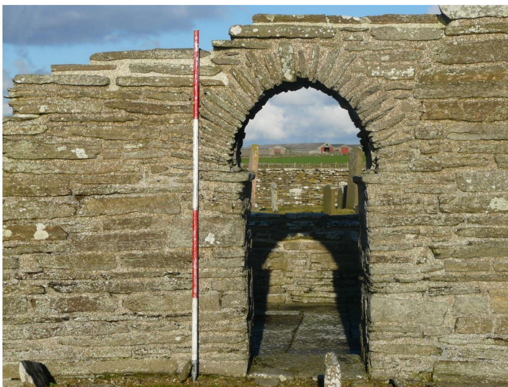
Figure 7 (above) – Crosskirk Tuquoy, south nave doorway. Scale 500mm; photograph Mark Thacker.
