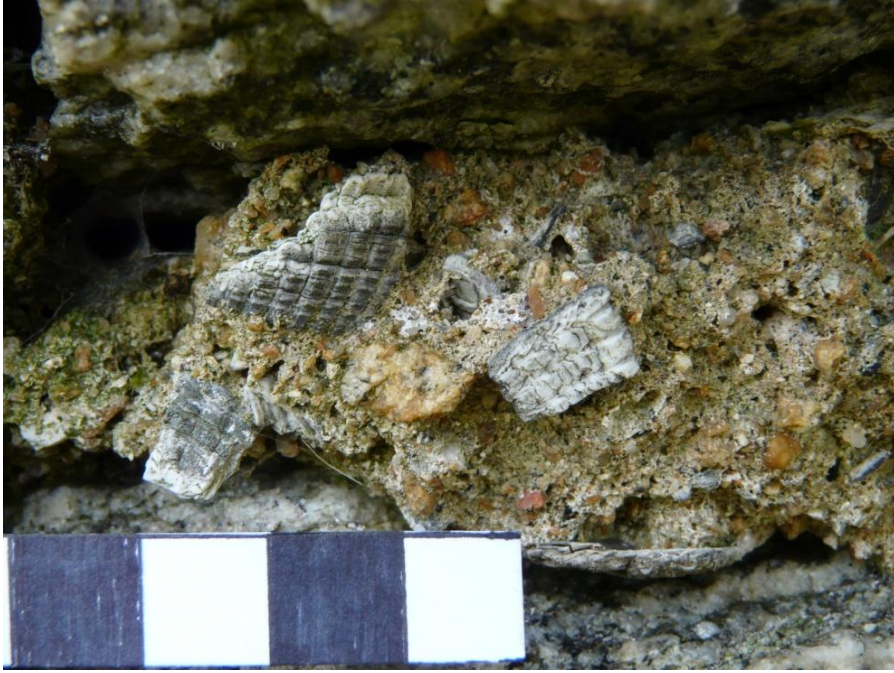
Figure 8 (above) - Primary mortar evidence in surviving east wall of Teampull Mòr, Howmore. Note Type 3 C.edule relicts and quartz-rich sand aggregate. Scale 10mm; photograph Mark Thacker.
