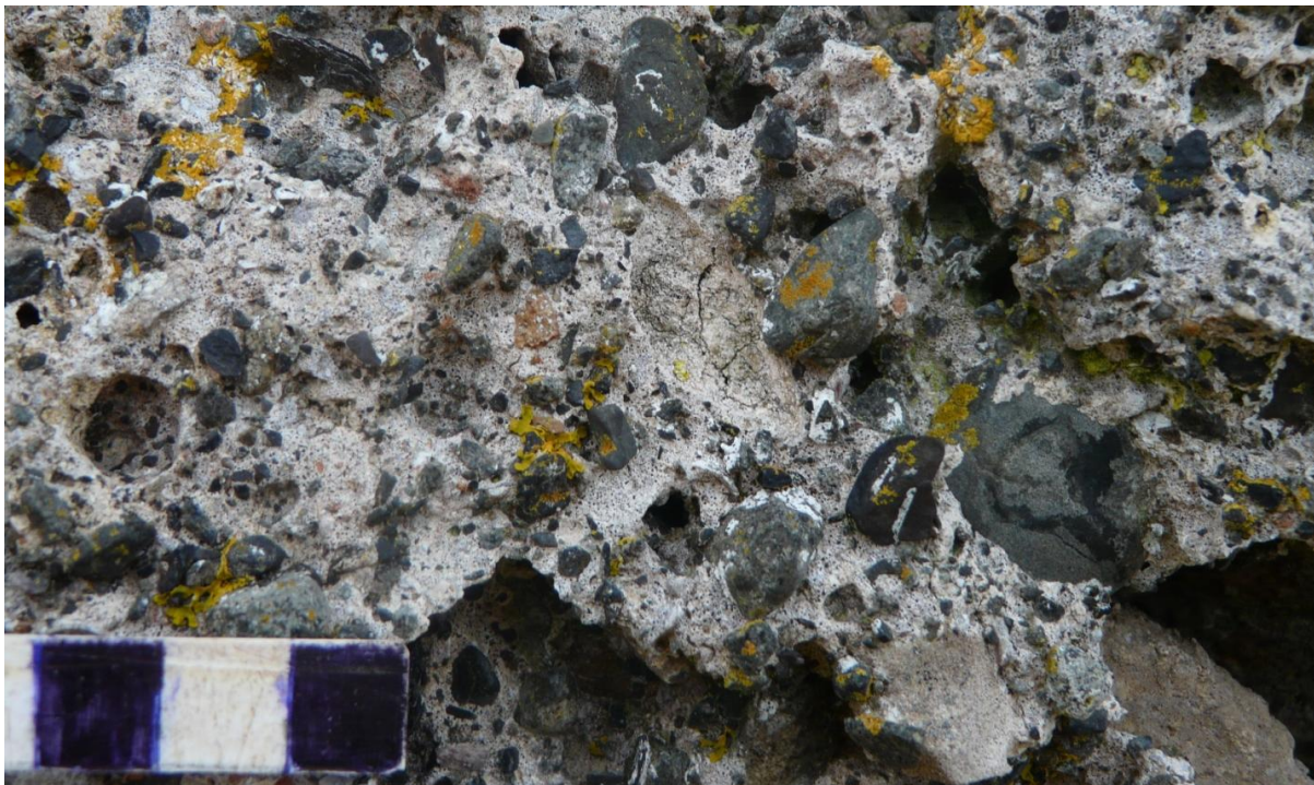
Figure 19 (above) - Mortar 10; External elevation of the north-west curtain parapet. 10mm scale; photograph M. Thacker.
