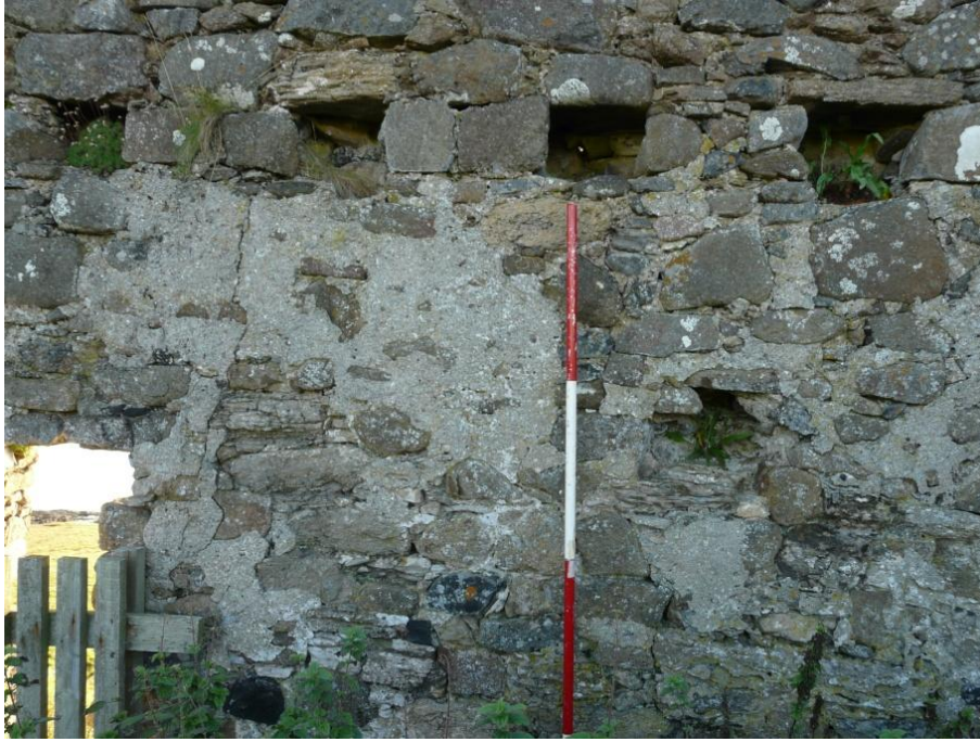
Figure 18 (above) - Internal south-west wall of west hall. Note informal use of very small gabbro stones. Scale 500mm; photograph Mark Thacker.
