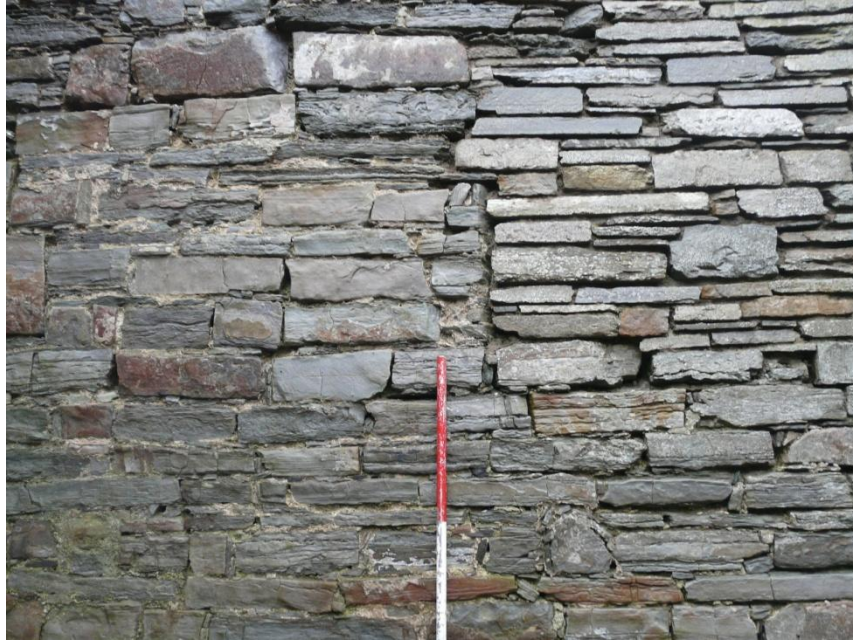
Figure 18 (above) – Nave; internal face of west wall; surviving remains of south jamb and splaying reveal of west window. Note the tighter jointing and sharp blocky primary masonry to left of the jamb. Scale 500mm; photograph Mark Thacker.
