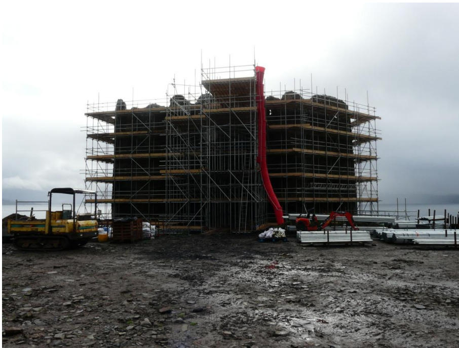
Figure 7 (above) – Mingary Castle from the north before main mortar survey in October 2013 when almost complete scaffold access was available. No scale; photograph Mark Thacker.
