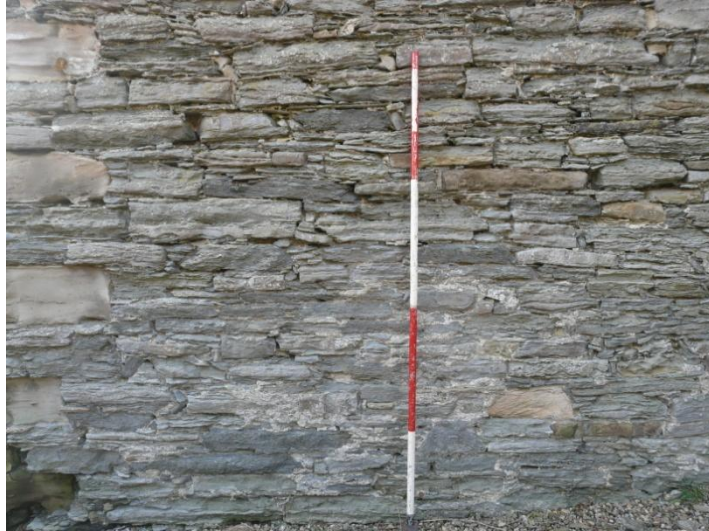
Figure 31 (above) – South Aisle; east face. Thin flagstone masonry with occasional fine sandstone. Highly eroded fine-grained sandstone quoins laid in strict alternate pattern. Scale 500mm; photograph Mark Thacker.
