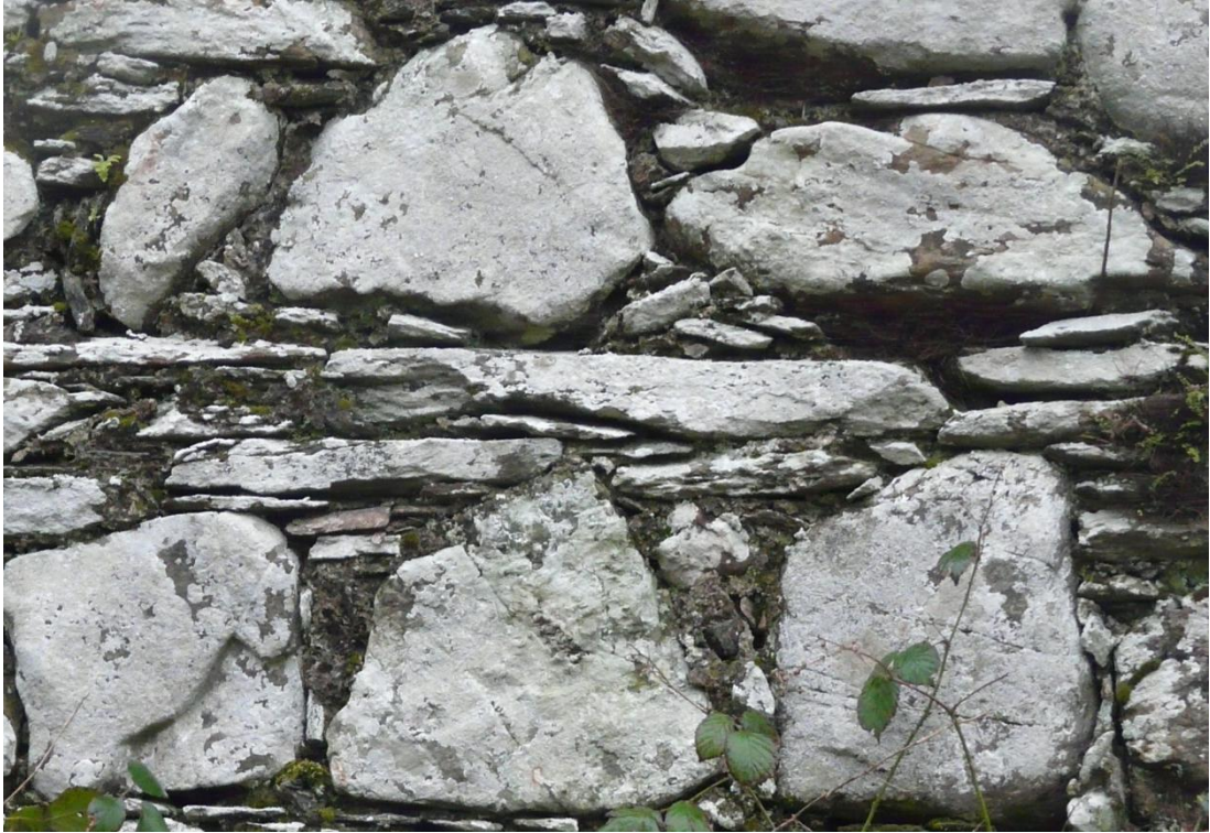
Figure 18 (above) External face of east wall of Killenuar Church, showing masonry style
