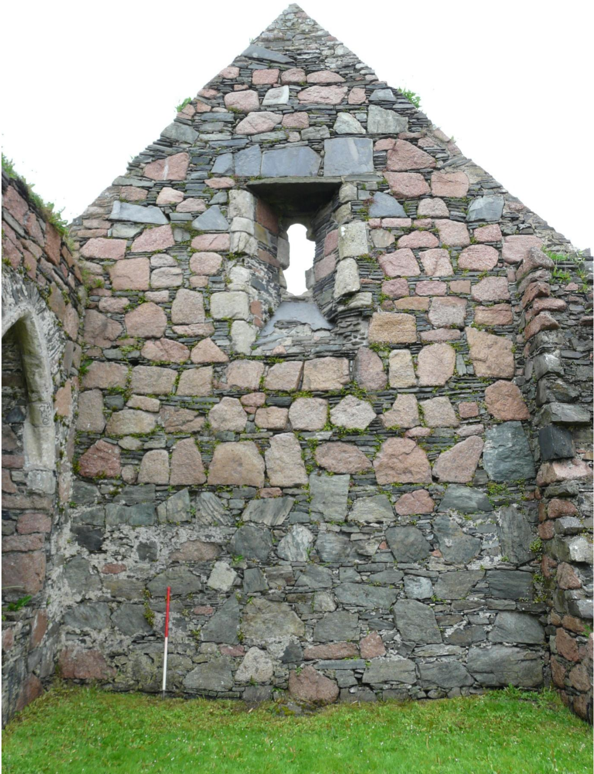
Figure 16 (above) - Internal face of Refectory west wall. Scale 500mm; photograph Mark Thacker.
