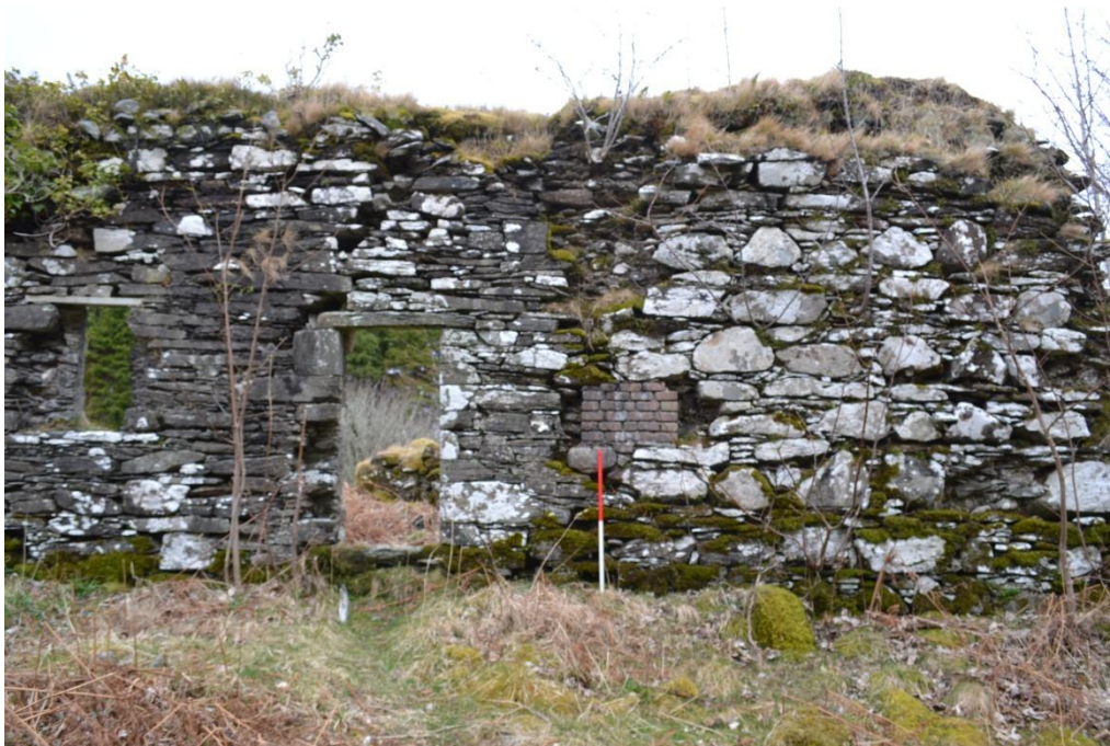
Figure 17 (above) – Detail of Kilneuir Church from the south showing contrasting masonry styles. The more formal primary medieval masonry is to the east, on the right of this image. Scale 500mm; photograph M. Thacker.
