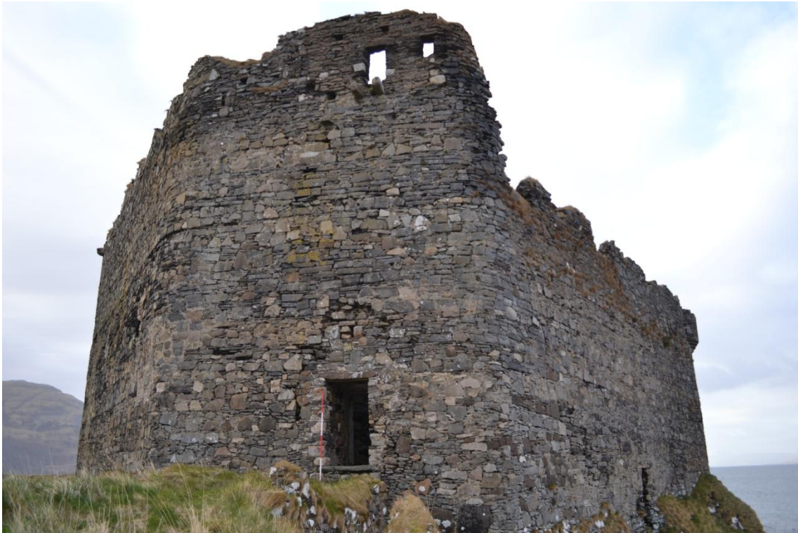
Figure 8 (above) North-west curtain wall. Scale 500mm; photograph Mark Thacker.
