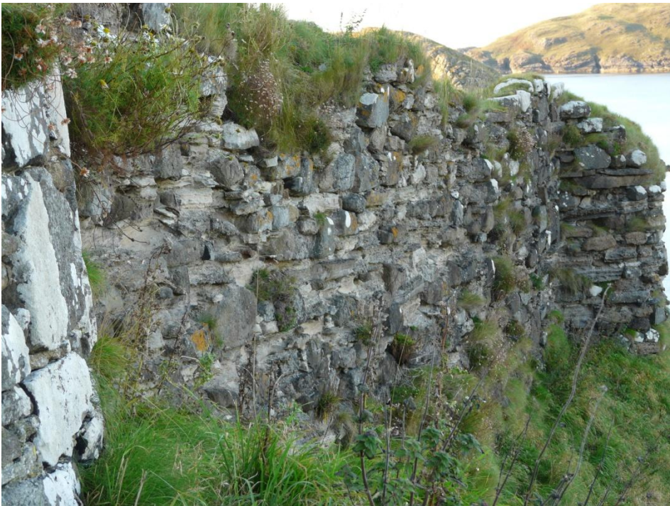
Figure 11 (above) – The north-east section of the east enclosure wall from the south-east. The masonry of the enclosure wall and drum tower appears consistent and provides great contrast with the small south-east section just visible on the left of his image. No Scale; photograph Mark Thacker.
