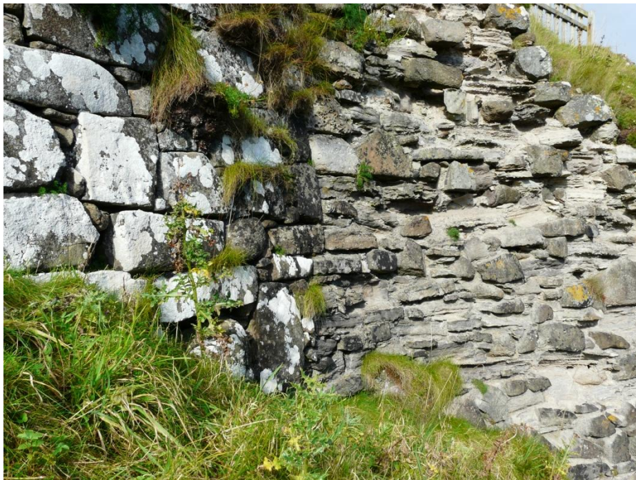
Figure 21 (above) - Phasing and contrasting masonry styles at south-east section of east enclosure wall. No scale; photograph Mark Thacker.
