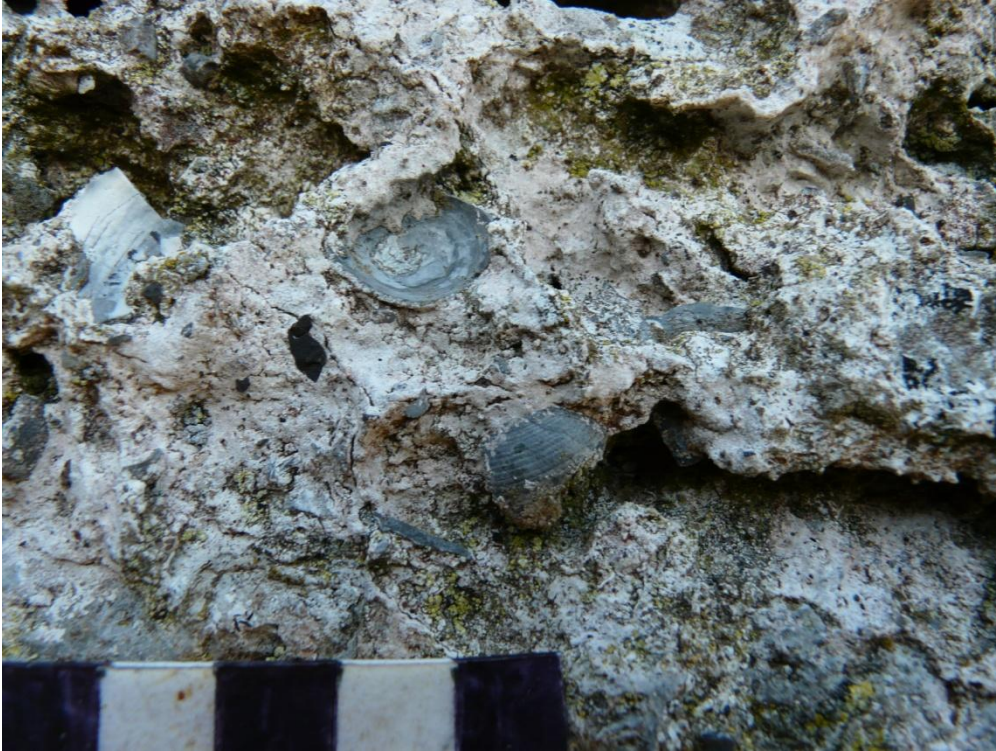
Figure 32 (above) - Shell-lime coating on internal face of south-east wall in west hall. Scale 10mm; photograph Mark Thacker.
