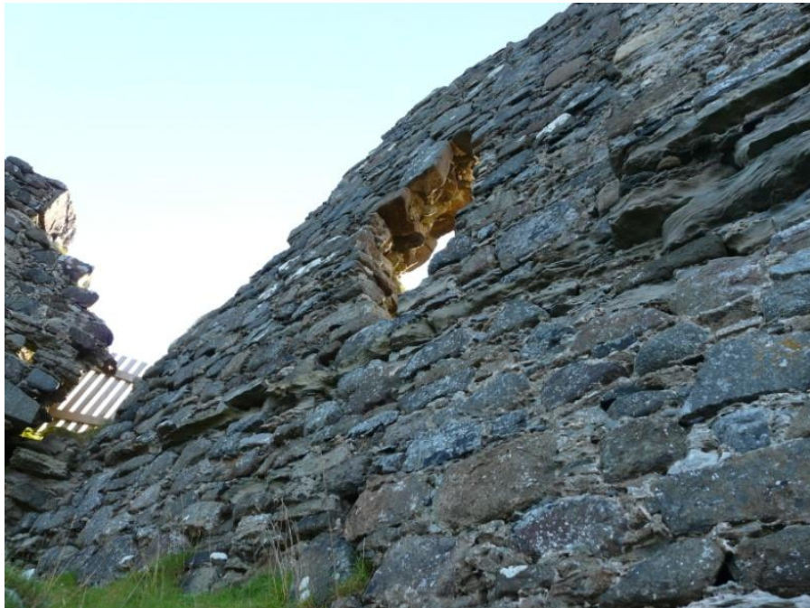
Figure 9 (above) – North-west external faces of north-west enclosure wall (lower) and west hall (higher). No scale; photograph Mark Thacker.
