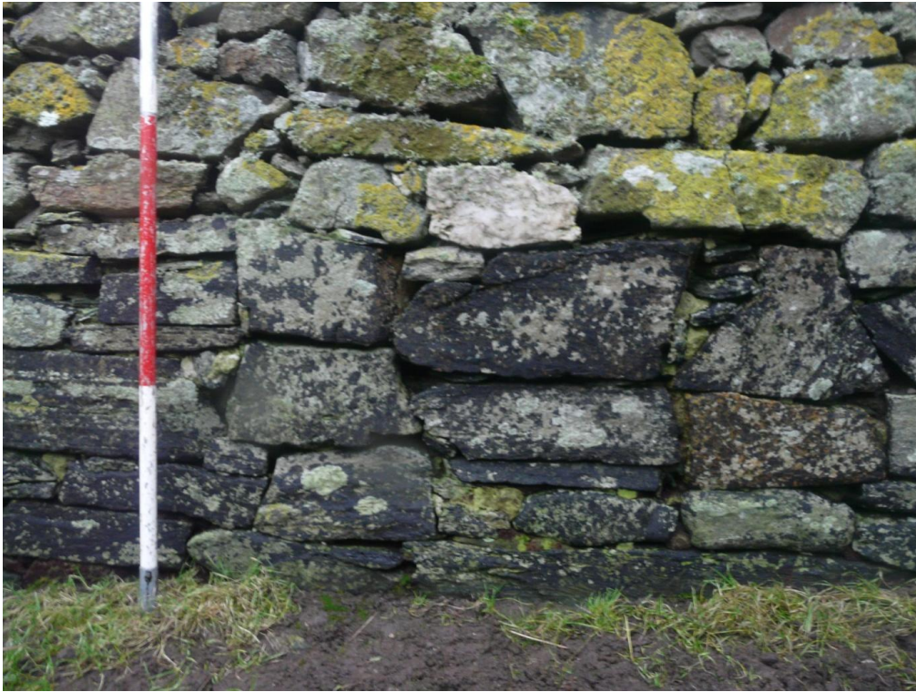
Figure 16 (above) – Uyea chapel nave, internal face of south wall. Phase 1 lime-bonded masonry below, overbuilt by Phase 3 dry-stone masonry. Note remarkably poor bonding of primary masonry, and resultant risbond joints. Scale 500mm; photograph Mark Thacker
