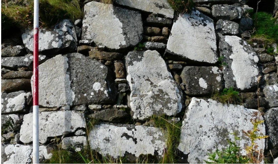
Figure 20 (above) – Masonry style of the south-east section of east enclosure wall. Scale 500mm; photograph Mark Thacker.
