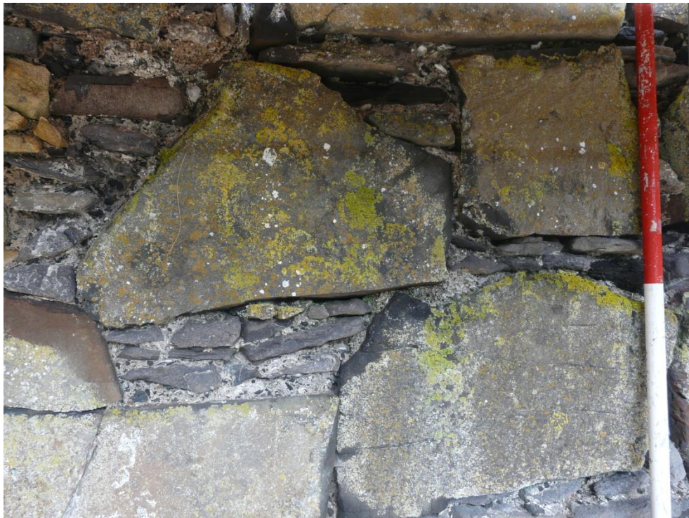
Figure 13 (above) – External face of north range displays very consistent bimodal distribution of stone sizes, dominated by very large dolerite blocks, laid level with stone-to-stone contact, and levelled-up with much smaller stone. Scale 500mm; photograph Mark Thacker.
