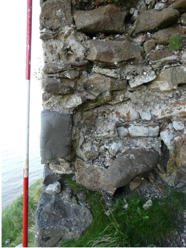
Figure 22 (above) – Multiphase masonry at the re-facing of primary west curtain. Scale 500mm; photograph Mark Thacker
