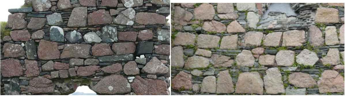
Figure 19 (above) – Masonry Styles; The bishop’s House on the left and Nunnery Refectory on the right. No Scale; photographs Mark Thacker.
