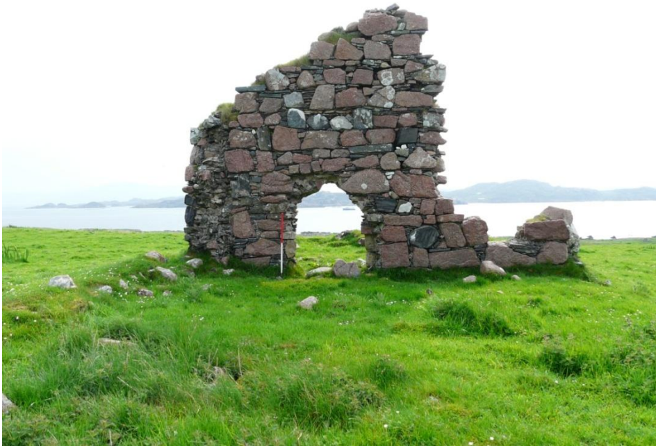
Figure 17 (above) – The Bishop’s House, Iona, from the west. The ruin is mostly comprised of the remains of the cross-wall and some of the external south wall. Scale 500mm; photograph Mark Thacker.
