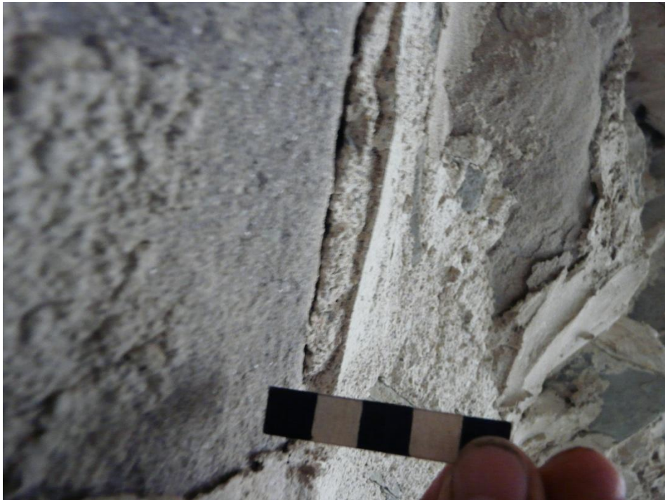
Figures 21 (above) – Coating 2; Lower chancel, above east window. Note two-coat system of fine lime-rich finishing coat overlaying coarser keyed scratch coat. Scale 10mm; photograph Mark Thacker.
