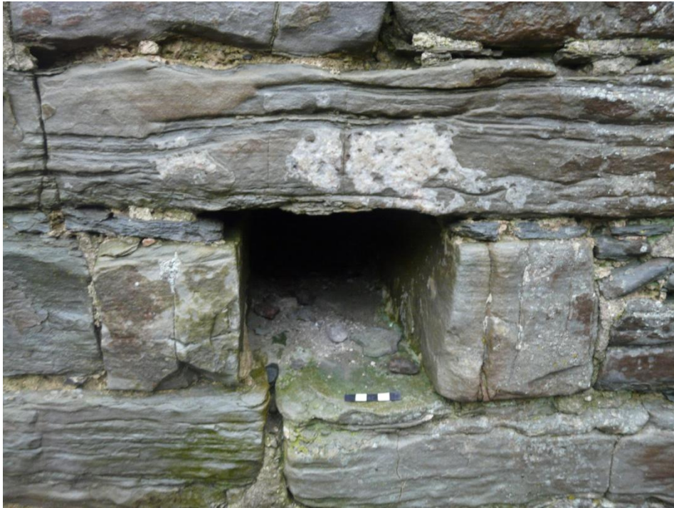
Figure 16 (above) – Primary fabric; putlog socket; internal south wall of nave. Note blocky hard blue sandstone typical of phase 1 and remains of quartz veining on the face of the lintel. Scale 10mm; photograph Mark Thacker.
