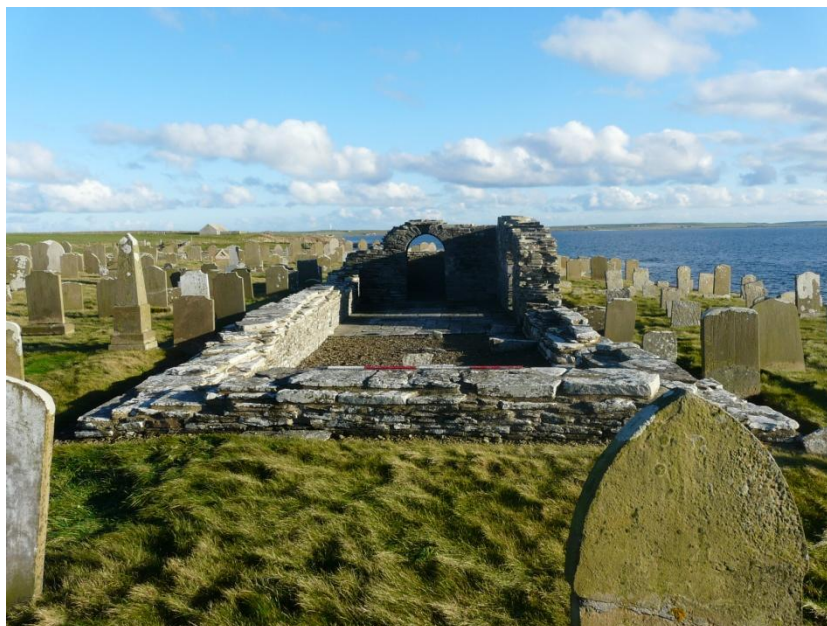
Figure 6 (above) – Crosskirk Tuquoy from the west with the secondary western extension in the foreground. Scale 500mm; photograph Mark Thacker.
