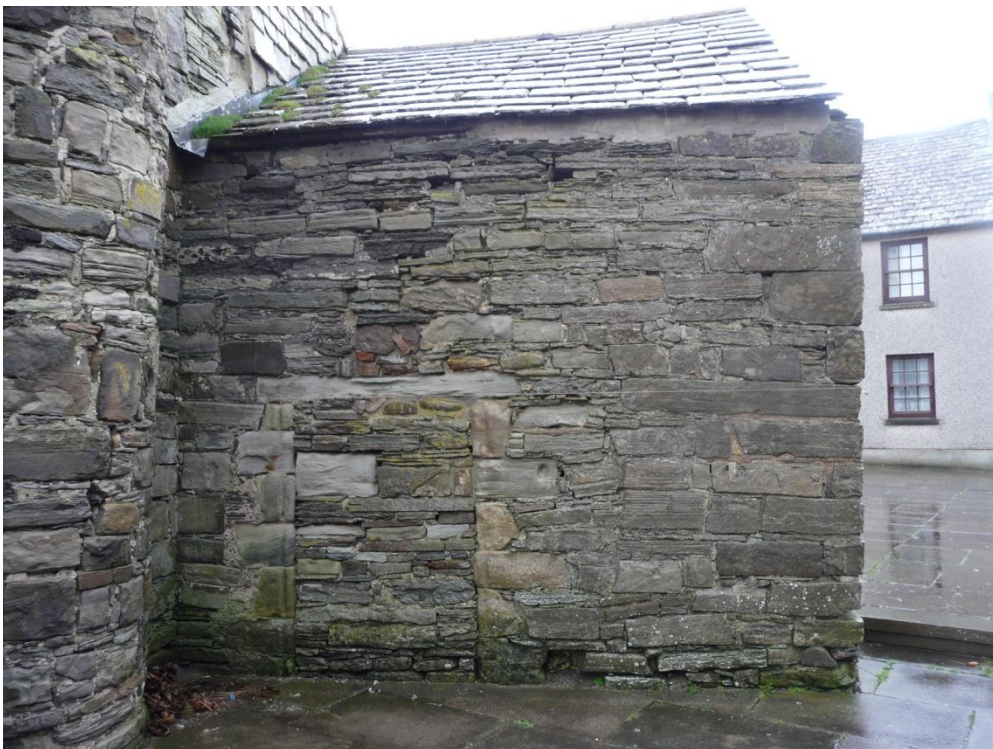
Figure 7 (above) – External face of south chancel wall. Note regular blocky primary masonry at south-east corner and disturbed masonry around secondary doorway and above. No Scale; photograph; Mark Thacker.
