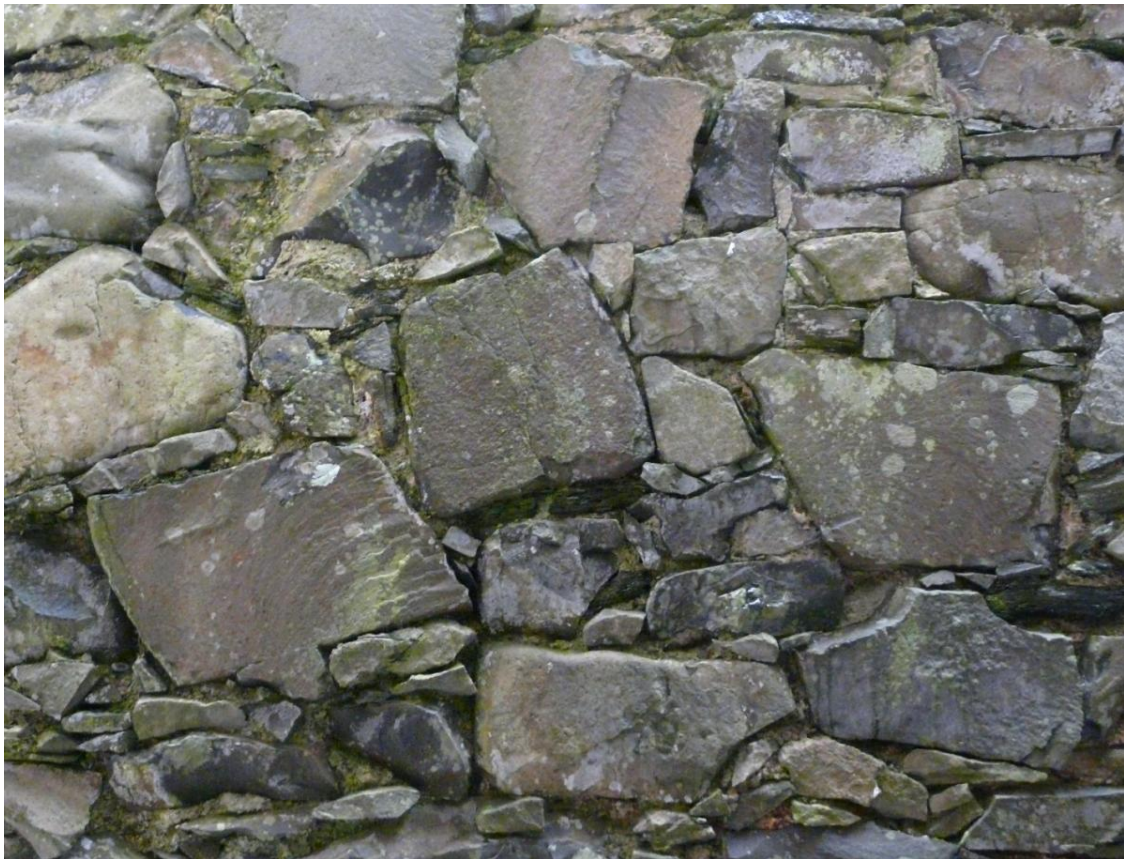
Figure 21 (above) - West range, north-west wall. No Scale; photograph M. Thacker.
