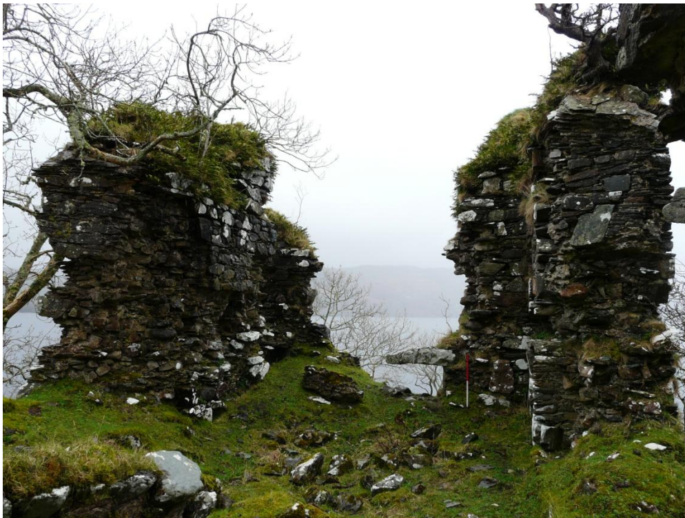
Figure 13 (above) –Inside Castle Fincham looking north. Large volumes of single phase core mortar exposed in multiple locations. Scale 500mm; photograph M. Thacker.
