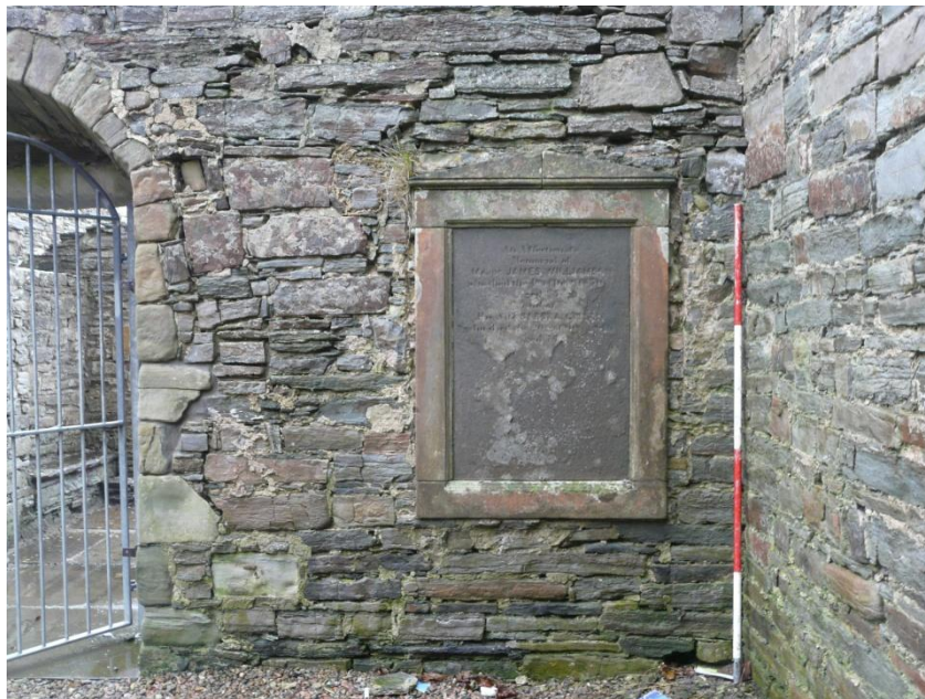
Figure 17 (above) – Primary south-west nave window with inserted memorial. Scale 500mm; photograph Mark Thacker.
