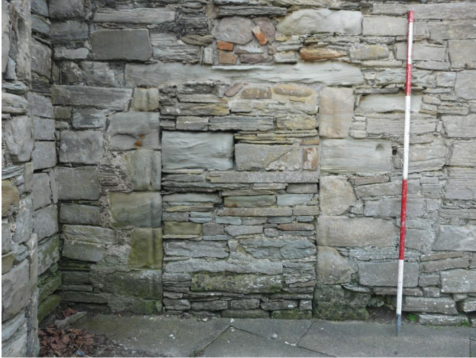
Figure 37 (above) – Blocked south chancel doorway; dressings display strict alternate bonding pattern; roll-moulded jambs; stooled lintel; blocked date plaque; eroded sandstone with iron-rich inclusions. Scale 500mm; photograph Mark Thacker.
