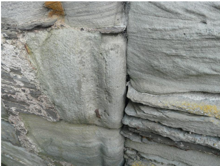
Figure 38 (above) – Roll-moulded jambs of south chancel door external dressings. No scale; photograph Mark Thacker.
