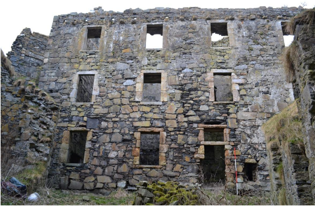
Figure 12 (above) – External face of south wall of north range. Note consistent lack of lateral bonding between very large dolerite face stones, very rough or no coursing, and dolerite quoins of south-west corner. Scale 500mm; photograph Mark Thacker.
