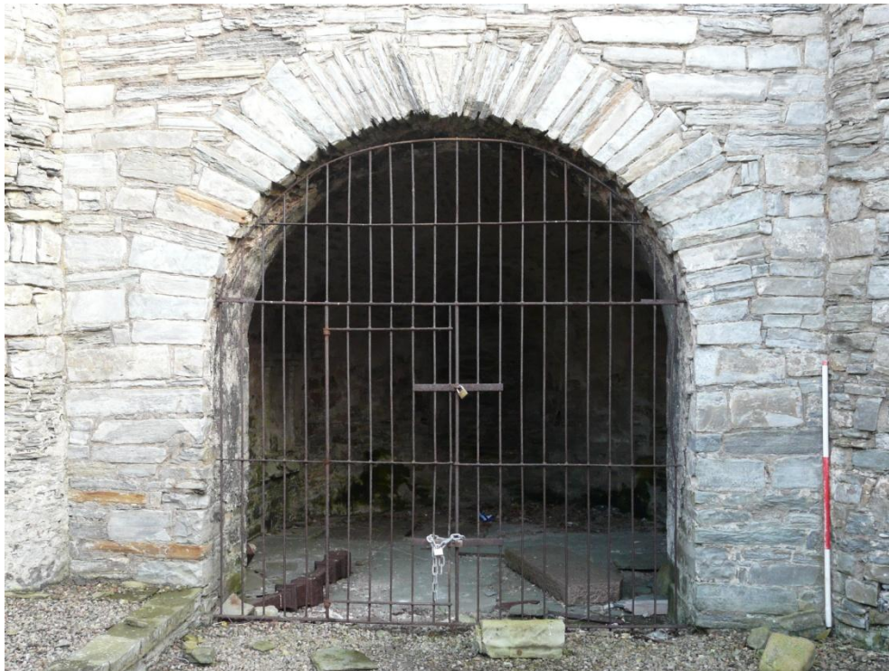
Figure 19 (above) – Chancel arch from the nave. Scale 500mm; photograph Mark Thacker.
