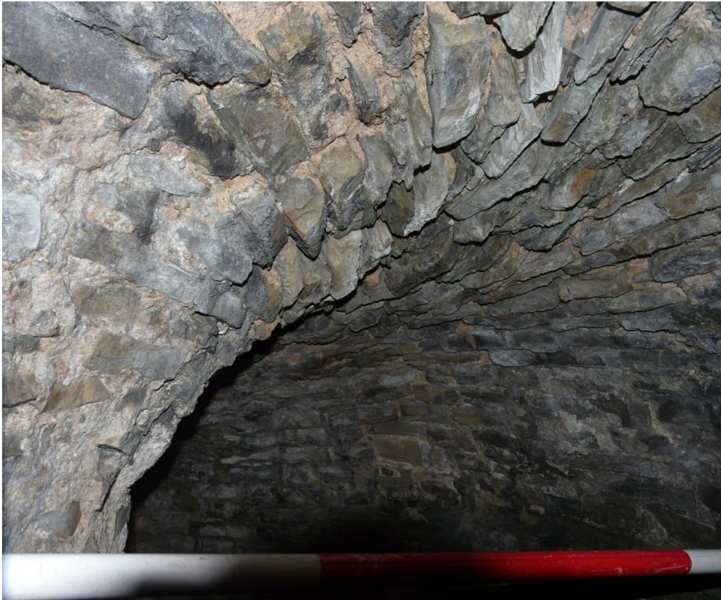
Figure 12 (above) - Lower tower spiral vaulting above stair. Scale 500mm; photograph Mark Thacker.
