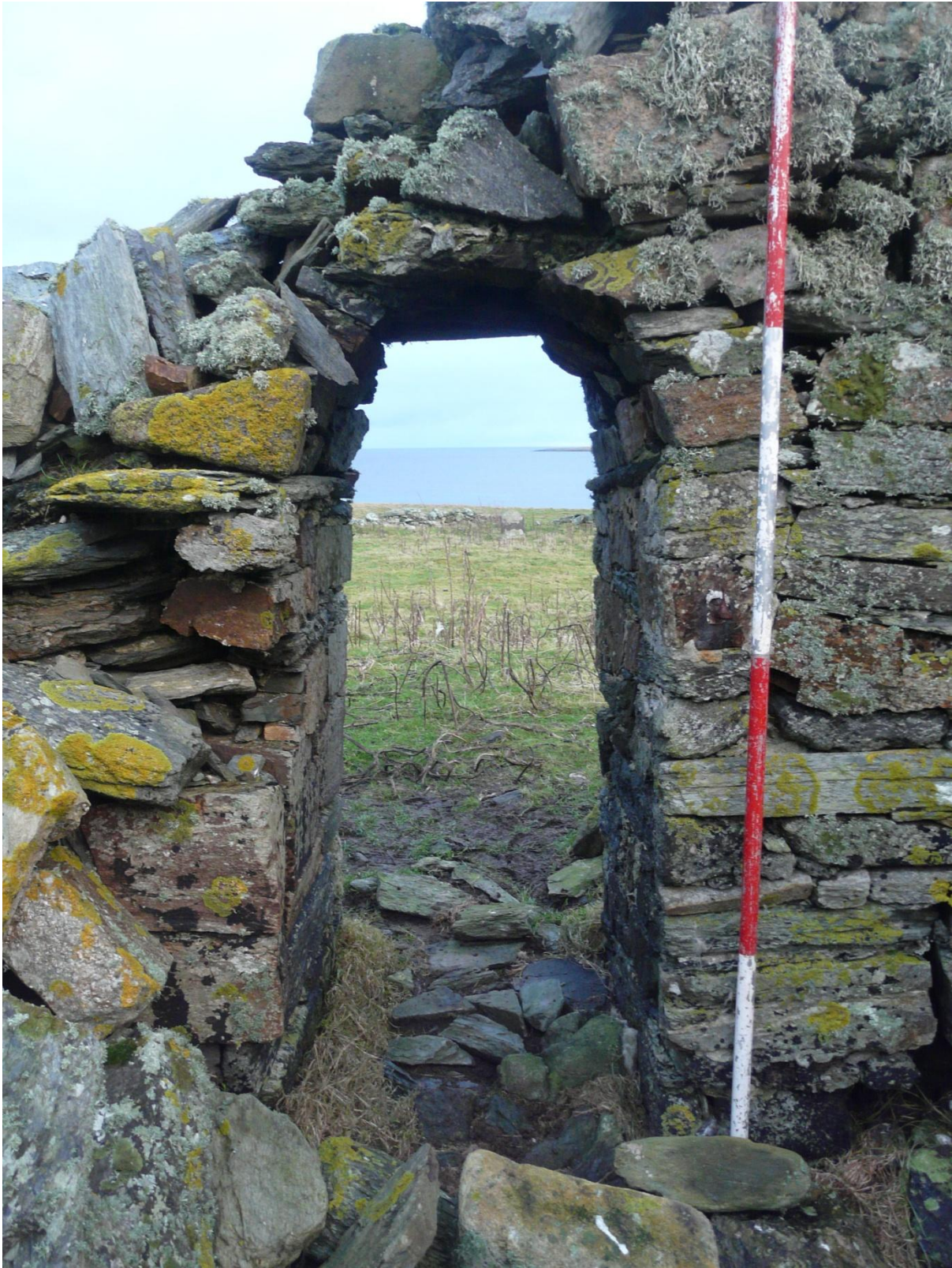
Figure 15 (above) – Uyea Chapel, west face of mid-wall chancel arch. Scale 500mm; photograph Mark Thacker
