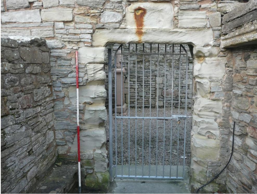
Figure 27 (above) – South-west nave doorway. Scale 500mm; photograph Mark Thacker.
