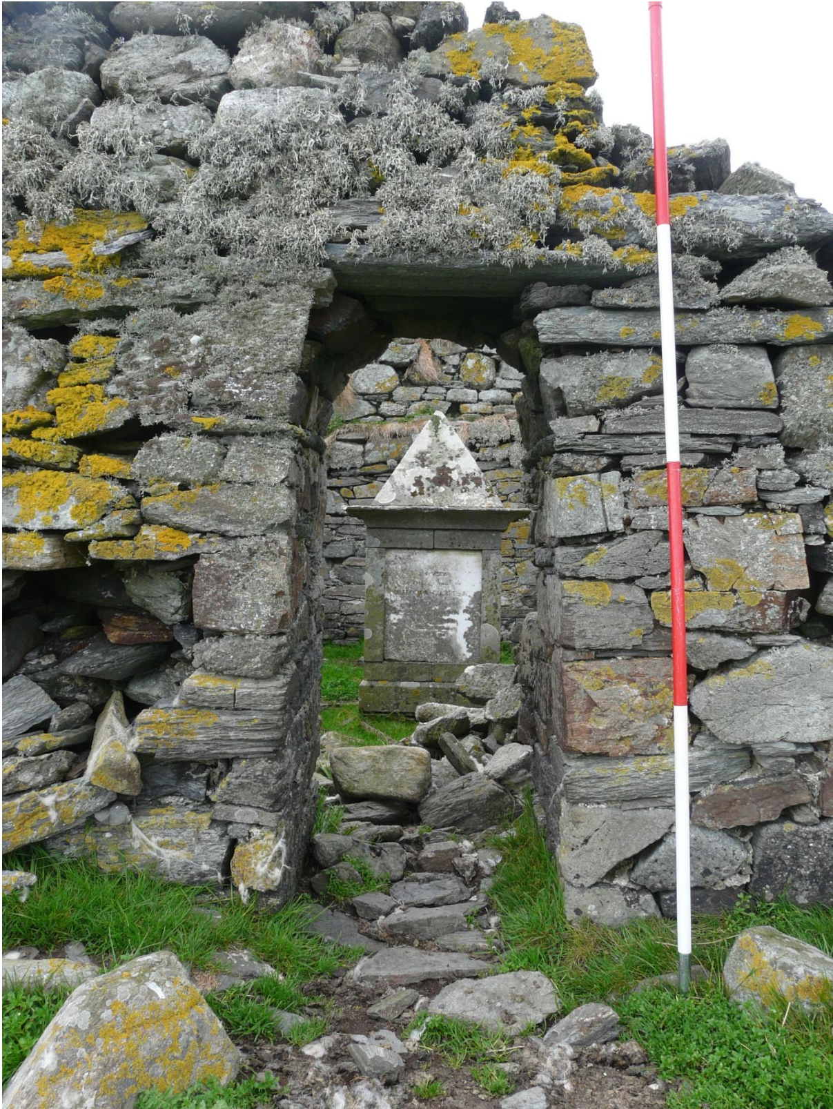
Figure 14 (above) – Uyea Chapel, east face of mid-wall chancel arch. Scale 500mm; photograph Mark Thacker.
