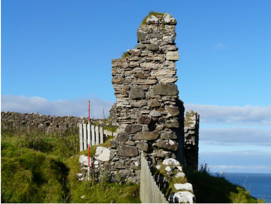
Figure 10 (above) – east wall of sea gate. Note contrast between lower (mafic, dipping) and higher (sedimentary, level) sections of masonry. Scale 500mm; photograph Mark Thacker.
