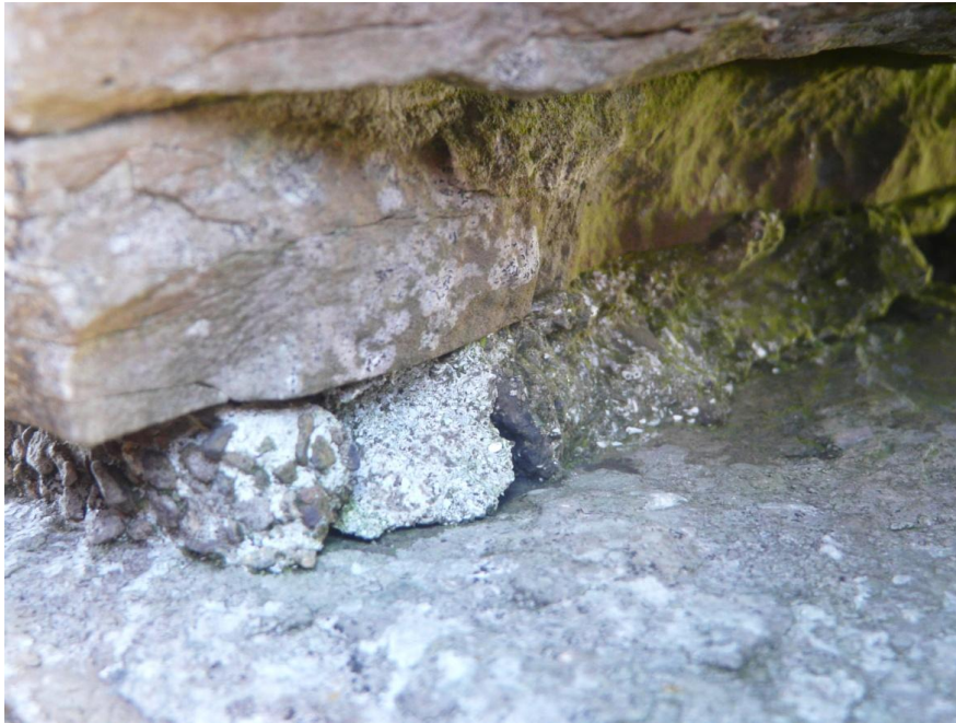
Figure 10 (above) - Crosskirk Tuquoy, external face of west jamb of south nave putlog. Note three phases of contrasting mortar. No scale; photograph Mark Thacker.
