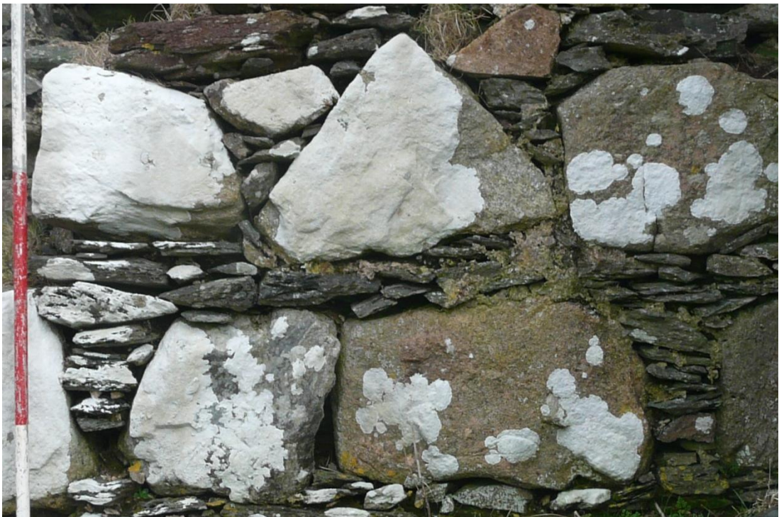
Figure 19 (above) Internal face of east wall of Castle Fincham, showing masonry style. Scale 500mm; photograph M. Thacker.
