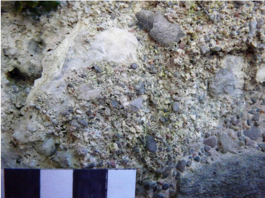
Figure 6 (above) – St Ronan’s shell-lime mortar internal coating and bedding context. Scale 10mm; photograph Mark Thacker.
