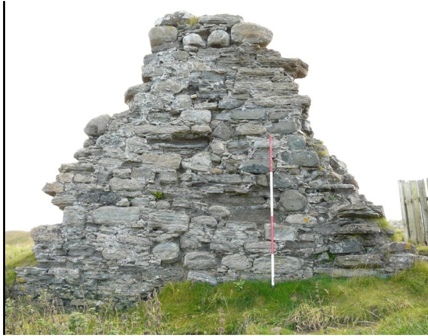
Figure 14 (above) Surviving fragment of external north face of south-east range. Scale 500mm; photograph Mark Thacker.
