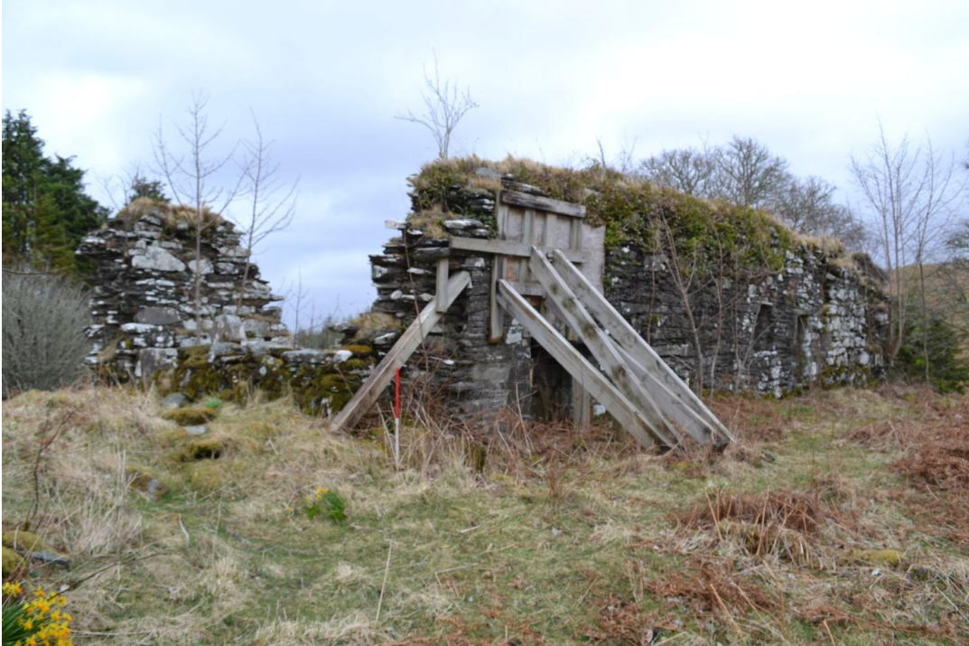
Figure 16 (above) – Kilneuir Church from the south-west. Scale 500mm; photograph M. Thacker.
