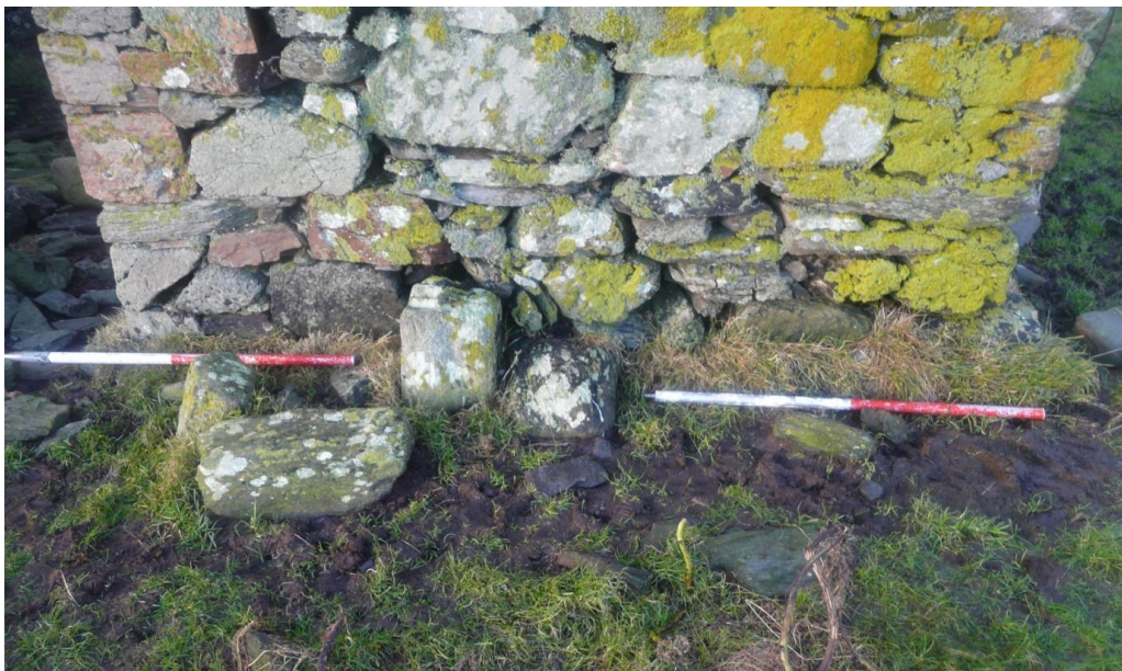
Figure 12 (above) – Uyea chapel, probable remains of north wall of chancel, protruding from the east face of the mid-wall of the chapel. Scale 500mm; photograph Mark Thacker
