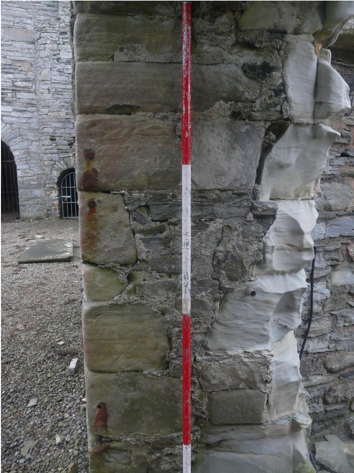
Figure 26 (above) – East reveal of south-west nave doorway into the church. Note the contrasting colouration, extent of erosion, and course heights between the inner and outer jambs. These also display contrasting lime mortars. The contrast in erosion levels is particularly striking where the two phases abut. It is suggested above that the left (north, inner) jamb is secondary late medieval phase 2, and the right (south, outer) is post medieval phase 4. Scale 500mm; photograph Mark Thacker.
