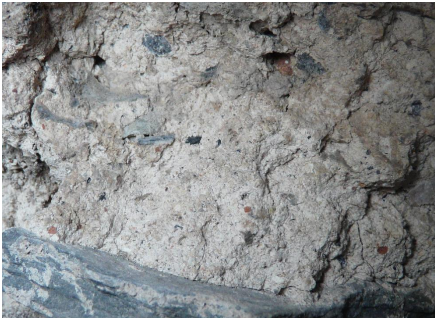
Figure 4 (above) – Mortar 1; External face of east chancel wall; deep core. Field of view approx. 50mm; photograph Mark Thacker.
