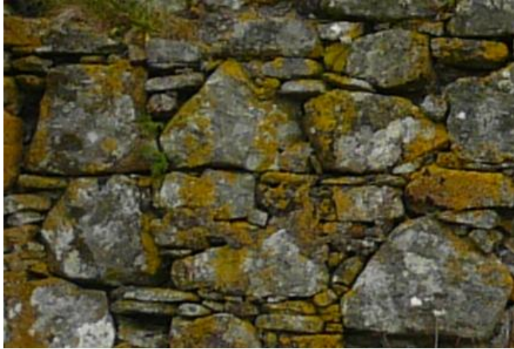
Figure 20 (above) - Teampull Mòr , Howmore, Internal east wall.
