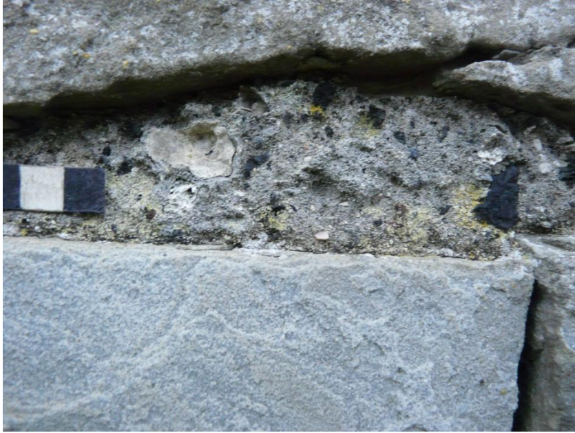
Figure 39 (above) – Chancel; external face of north wall; high courses; Mortar in bed context. Scale 10mm; photograph Mark Thacker.
