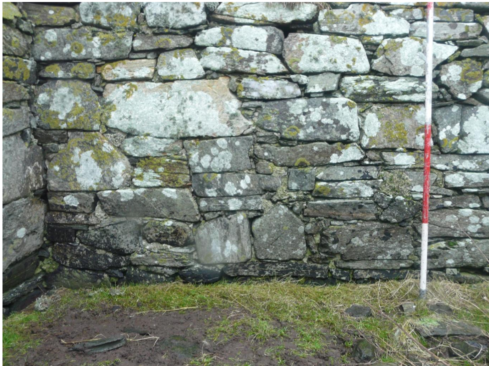
Figure 17 (above) – Uyea chapel nave, internal face of north wall. Tightly jointed poorly-bonded masonry. Scale 500mm; photograph Mark Thacker
