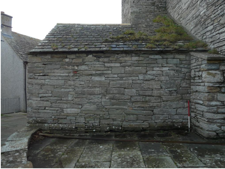
Figure 6 (above) – North chancel wall; external face. Note blocked primary chance window. Scale 500mm; photograph Mark Thacker.
