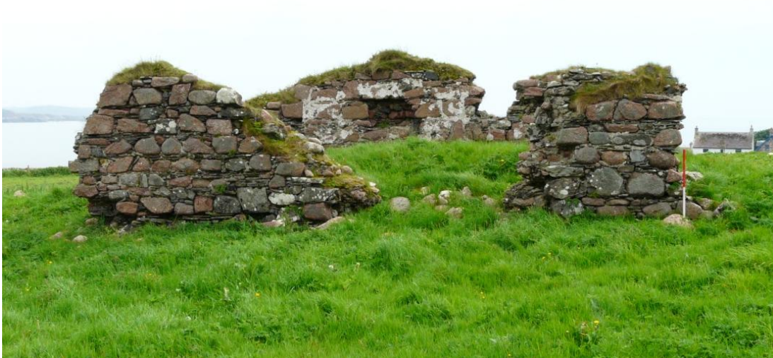
Figure 11 (above) – St Mary's chapel Iona from the north. The upstanding ruin is mostly comprised of the remains of the north and south walls. Note formal coursing and remain of bright internal mortar coating. Scale 500mm; photograph Mark Thacker.
