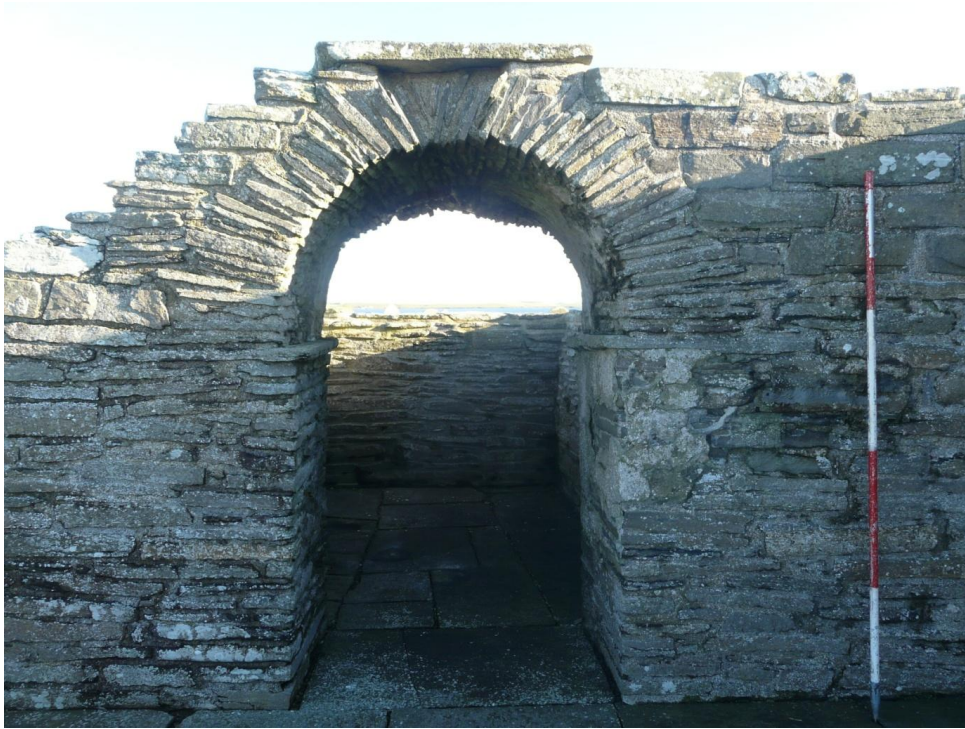
Figure 8 (above) - Crosskirk Tuquoy chancel arch from the west. Scale 500mm; photograph Mark Thacker.
