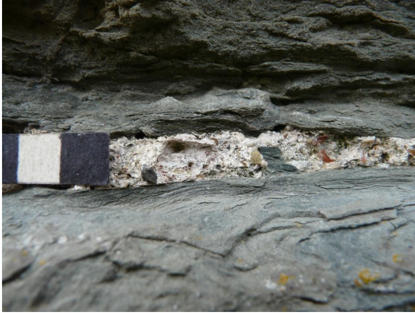
Figure 35 (above) – South Aisle; external east face; bedding mortar in-situ ; Mortar 4 . Scale 10mm; photograph Mark Thacker.
