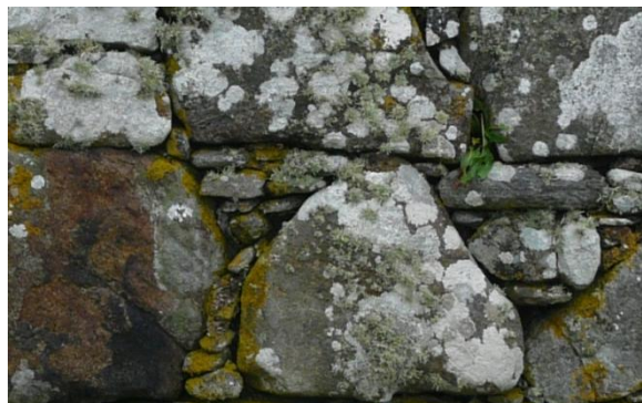
Figure 22 (above) - Cabeal Clann ic Ailean , Howmore, External west wall.
