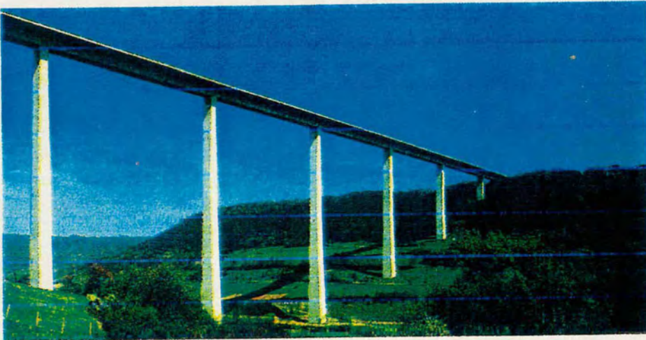
b) Kocher Viaduct, Germany
