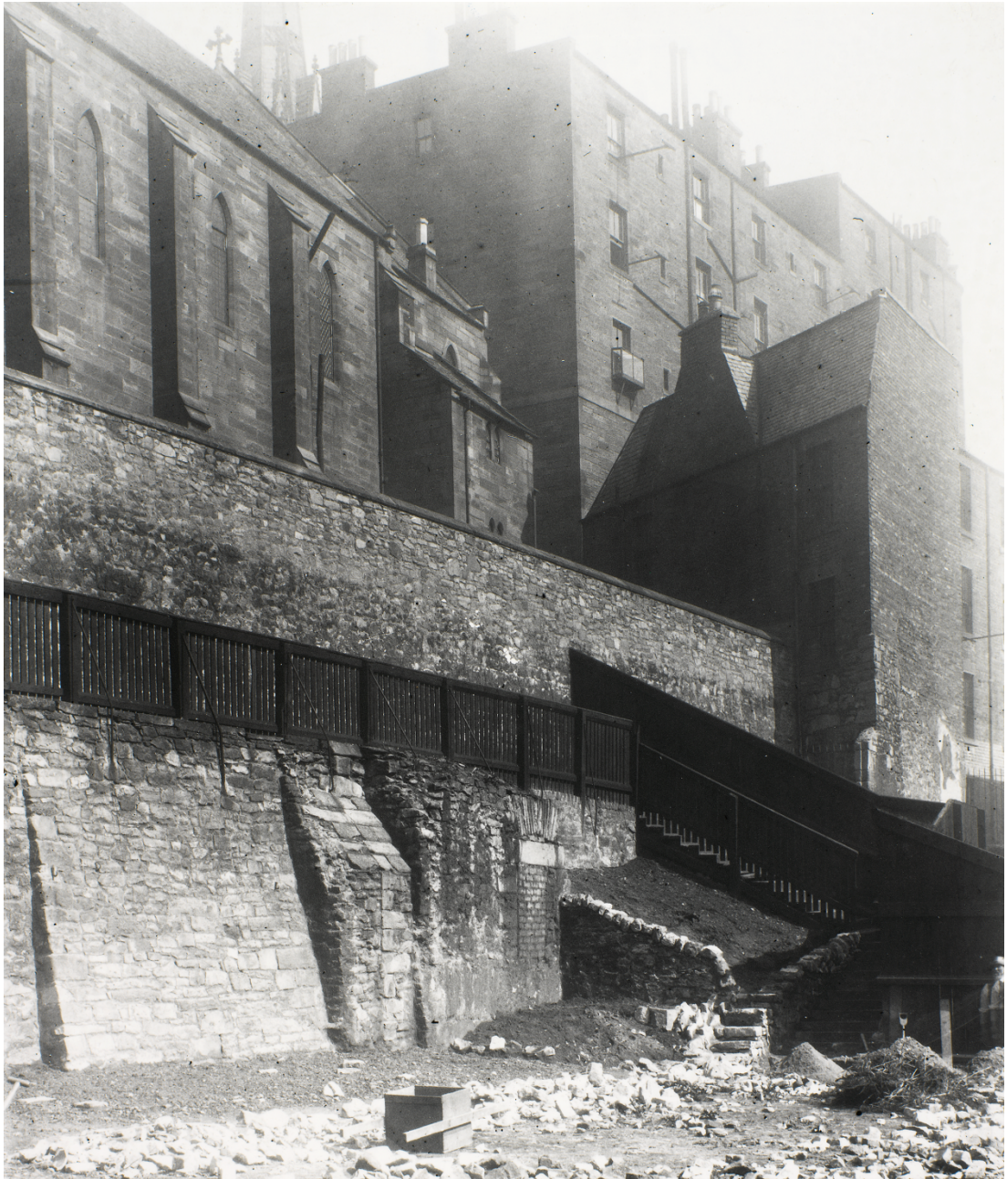
Figure 6.39 The proposed steps in the King's Wall Garden under construction c.1909-10. Sourced and reproduced with permission of the CRC, Geddes Photographs, J9.
