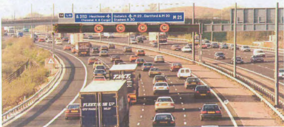
Figure 6.14 M25 Controlled Motorway
