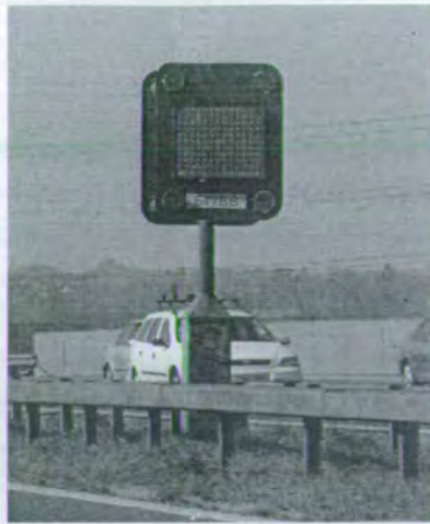
Figure 3 Example of central reservation post mounted matrix signal.
