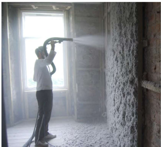
Figure 29: Cellulose sprayed over the existing brick wall existing dry lining.
