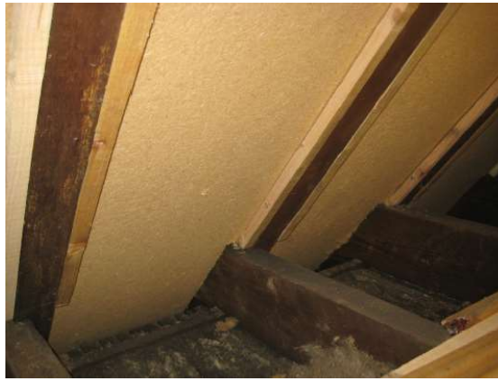
Figure 33: Wood fibreboards between rafters. [50].
