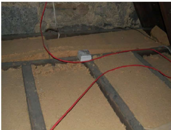
Figure 31: Wood fibre insulation between ceiling joists Figure 32: Wood fibre insulation between floor joists
