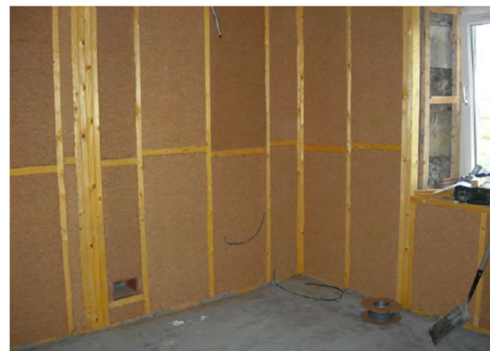
Figure 36: MDB or rigid wood fibre insulation in a frame.
