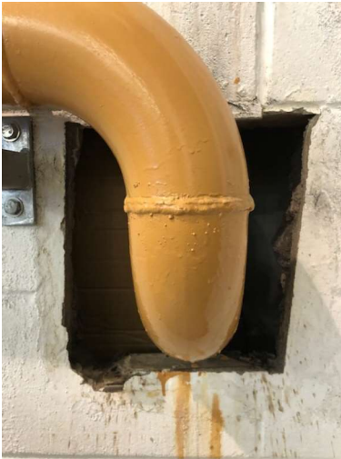
Figure 41: Undefined hole in the building envelope. Figure 42: Manual 3D scanning of hole
