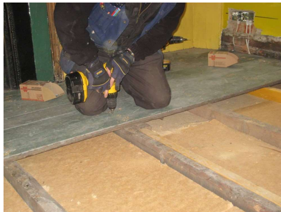
Figure 31: Wood fibre insulation between ceiling joists Figure 32: Wood fibre insulation between floor joists
