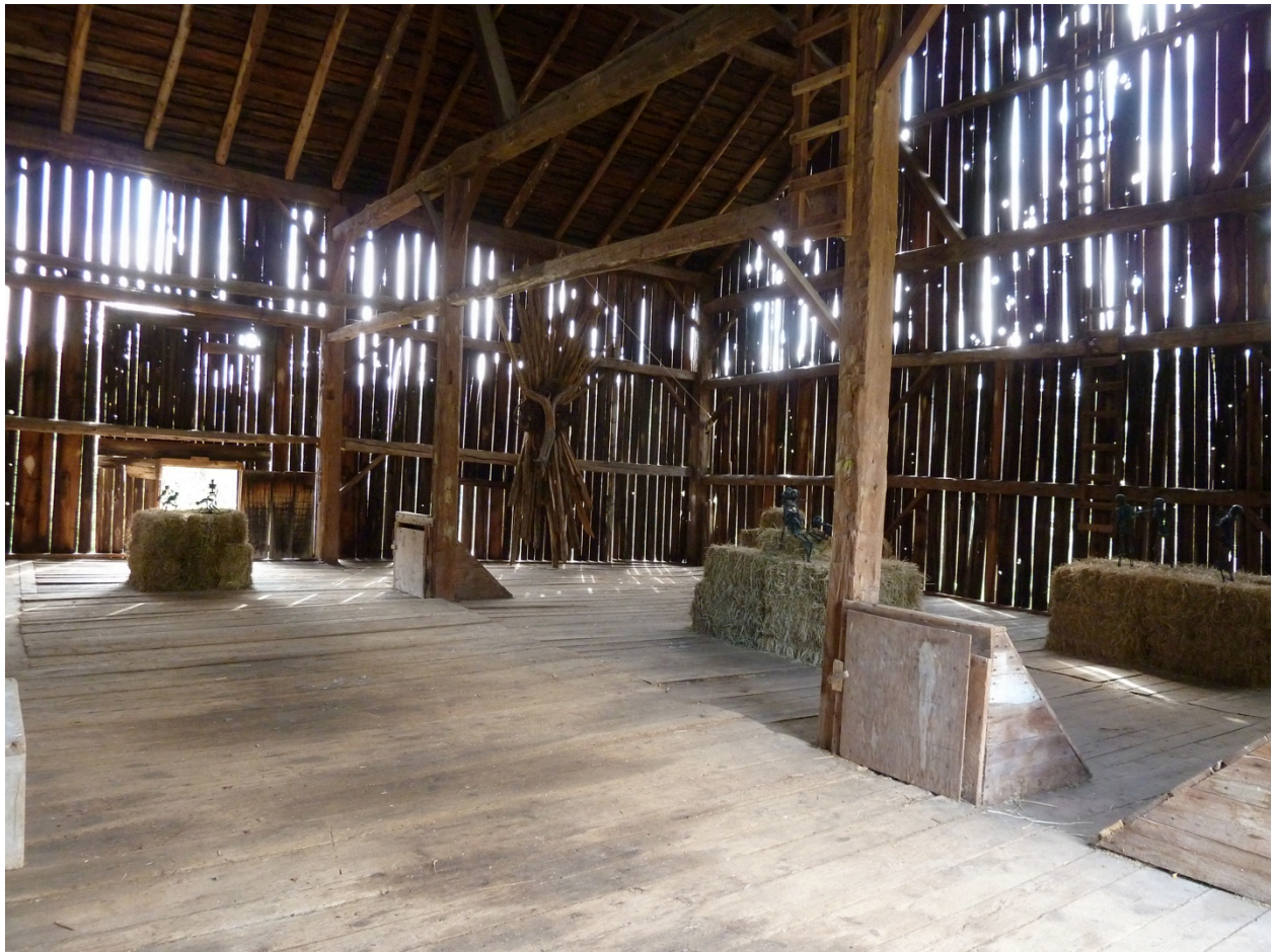
Fig. 97 View from the entrance of barn.
