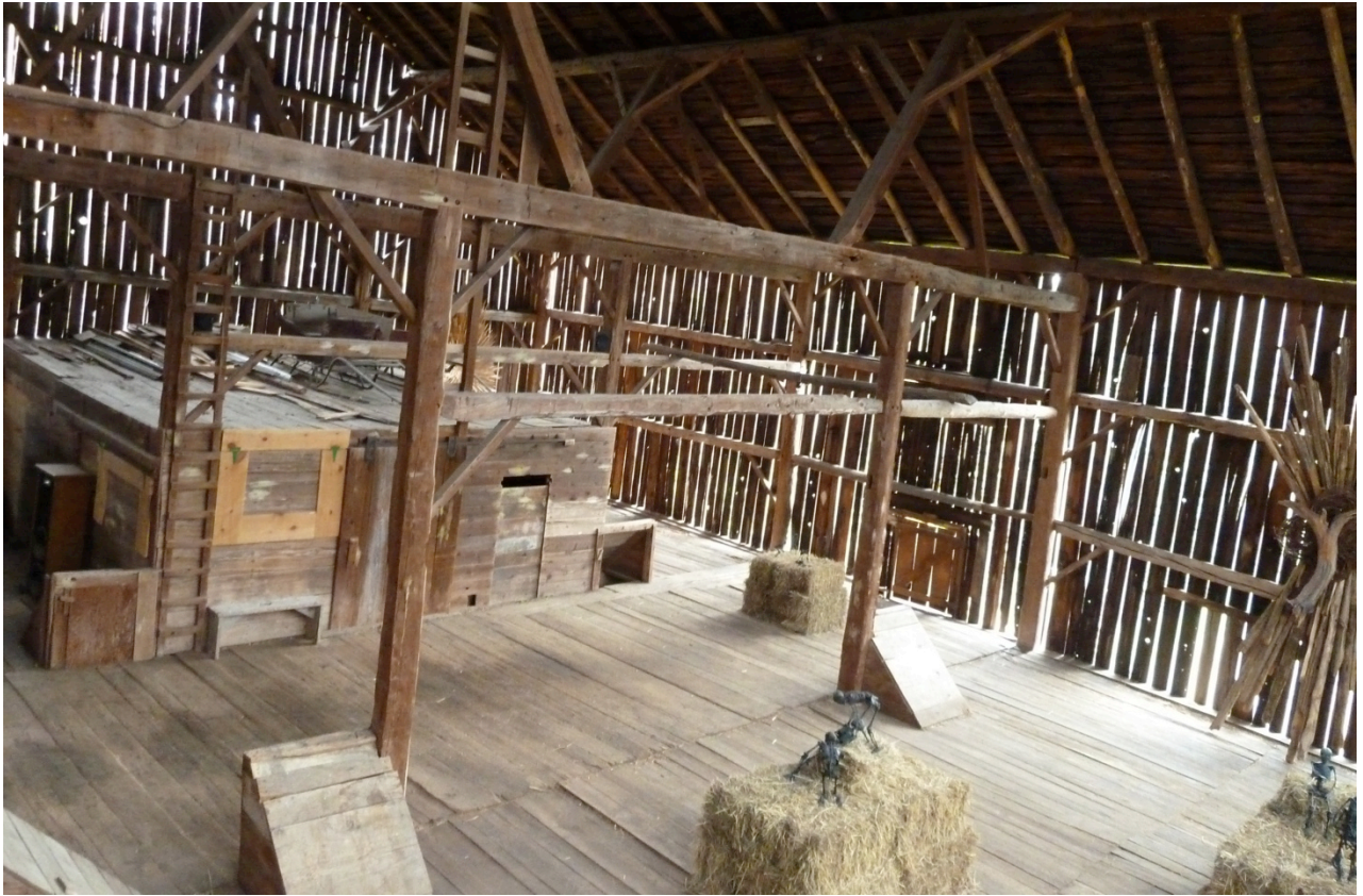
Fig. 148 Interior of barn/studio showing the compartmentalised grain room.
