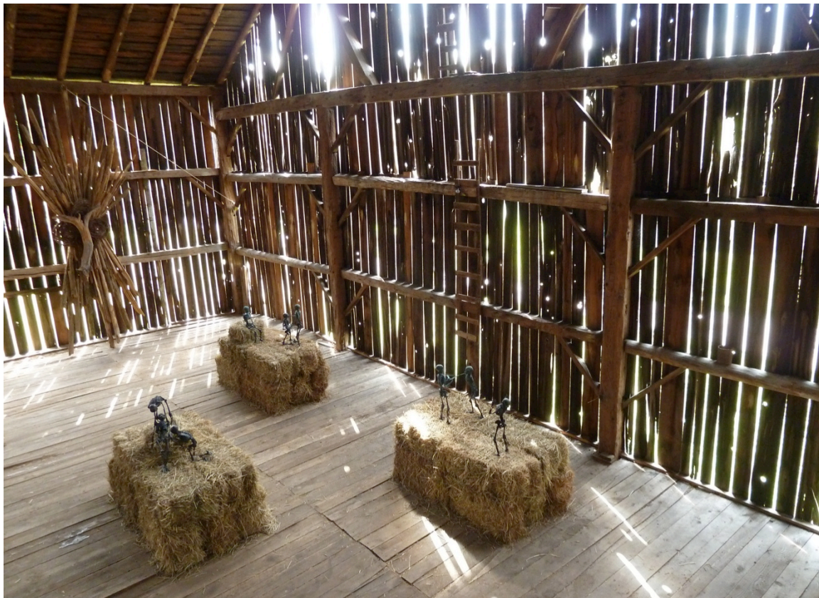
Fig. 107 Interior of Barn/studio. 2011
