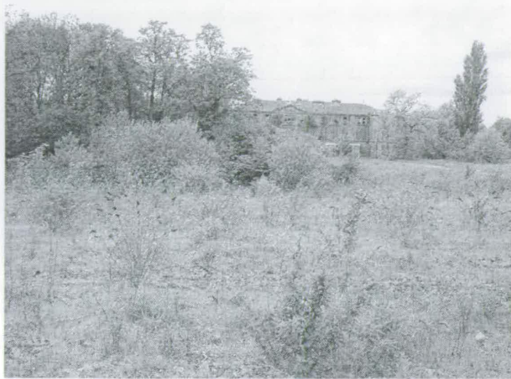
Fig 9. Belvidere Hospital area: site photograph taken on 14 May 2004 (Scholz, et al. , 2006).
