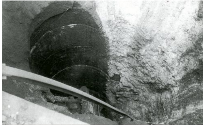
Figure 2.6. Photograph of collapse mineshaft with the front of the locomotive visible ( Shryhane, 2007 )
