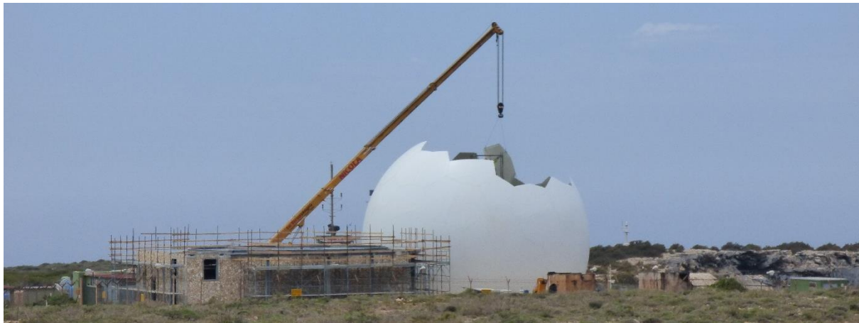
Figure 19 - Completion of the radome of RAT-31DL in May 2018
