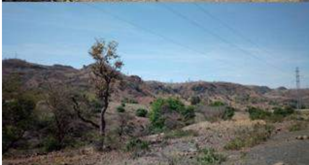
Figure 5.10 Pylons connecting the Beles power station to the national grid.
