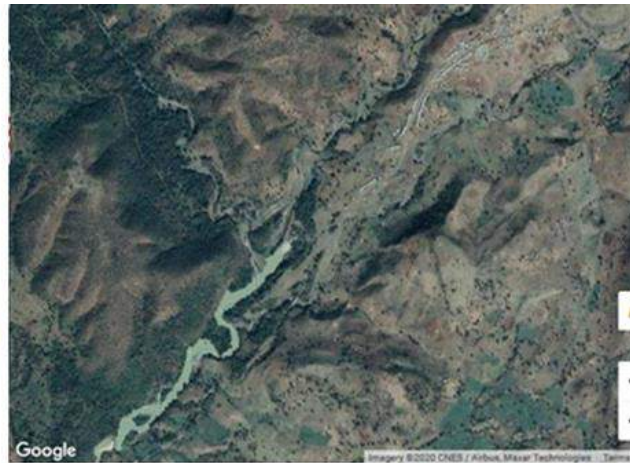
Figure 5.5 The outlet of the 20 km tunnel and some settlements along the road constructed for the Beles MPP (Google, 20 th July 2020)
