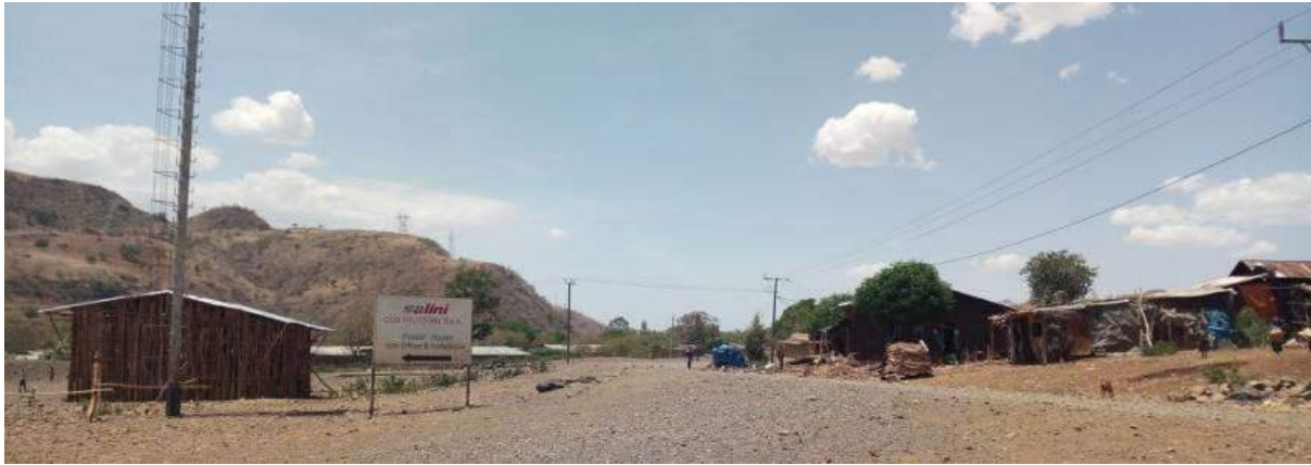
Figure 5.11 A Salini sign indicating the entrance of the underground power station. This village has been provided with electric power since 2018.
