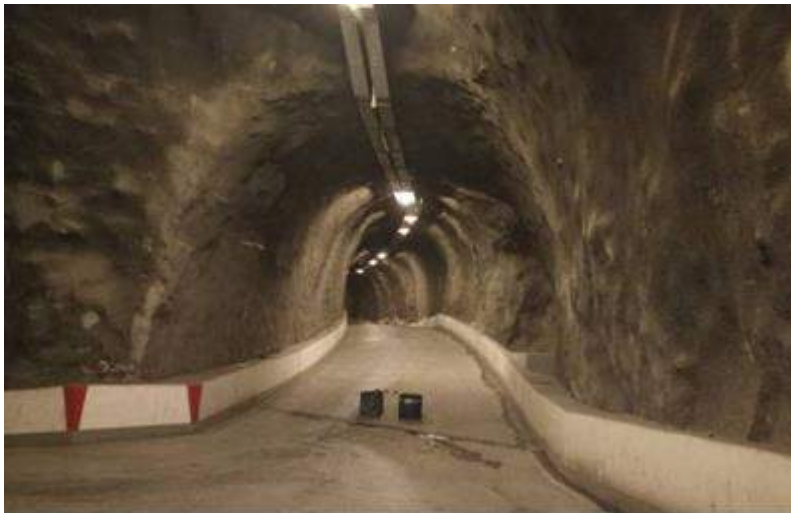
Figure 5.12 A sophisticated underground road system leads to the command centre and the actual power station.
