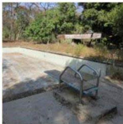
Figures 4.22 and 4.23 One of the former TBP dining halls is still in use by the Tana-Beles Girls' Boarding School that has moved into the compound; the Italian swimming pool has remained dry for almost three decades.
