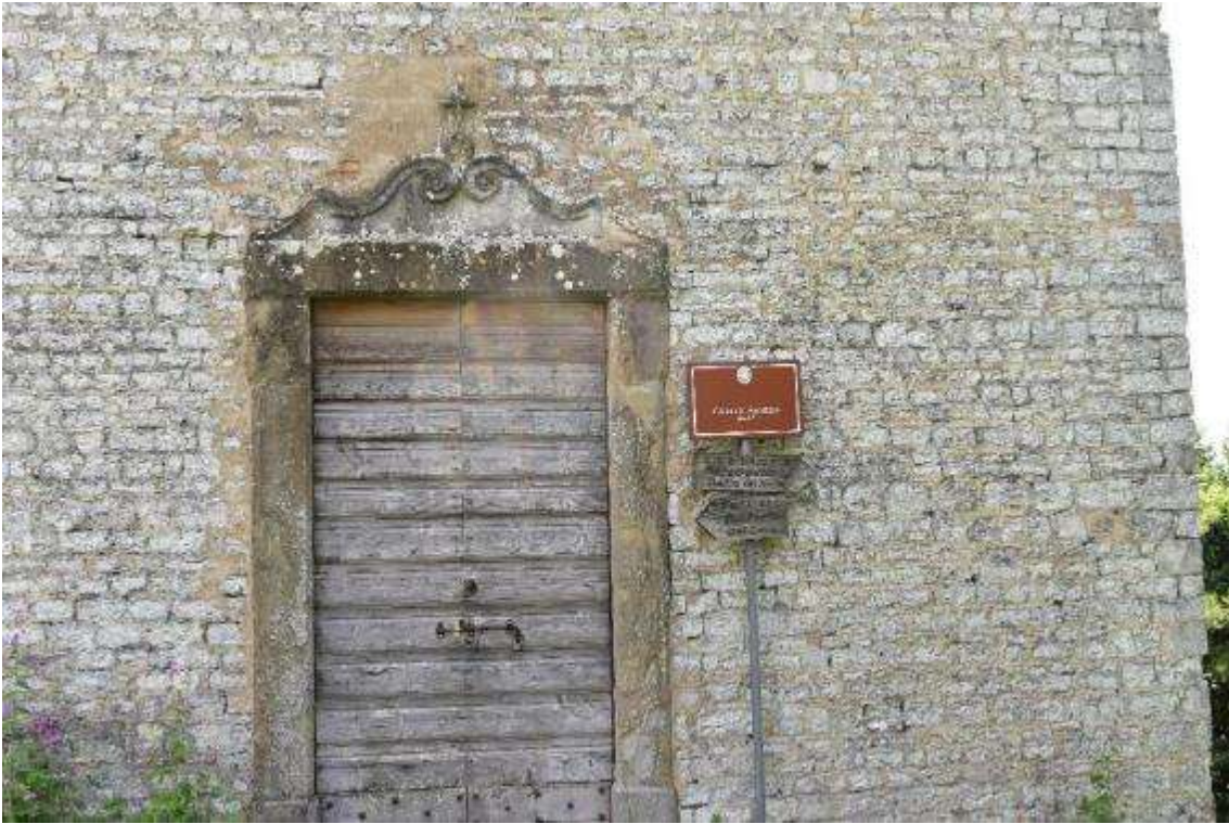
Fig. 7. 15 Church of St Augustine with two road signs, May 2022, Arcevia.
