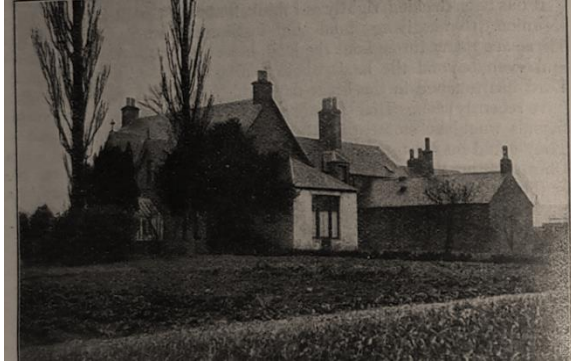
Figure 3.4 Buildings at Cornton Farm ( Life and Work , January 1930, 24).
