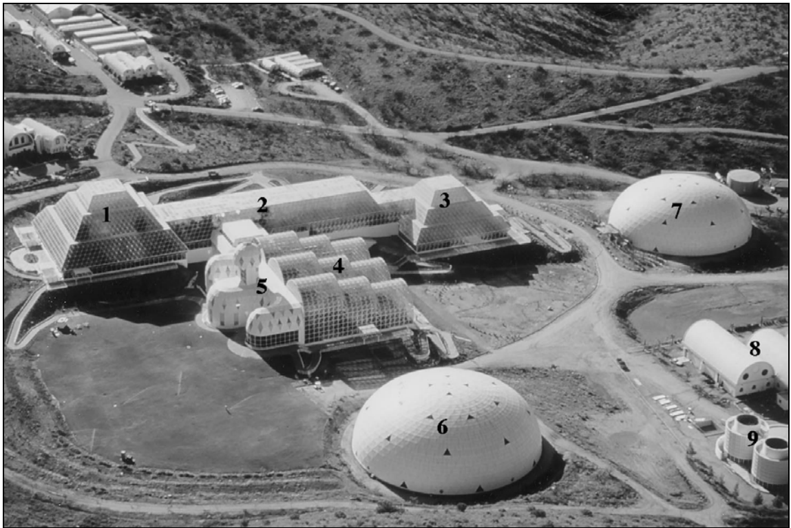
Figure 1.6. Aerial view of the Biosphere 2 Laboratory facility facing South-East showing the mesocosms: 1, tropical rainforest; 2, savannah-ocean-marsh; 3, desert; 4, intensive forestry mesocosm; 5, human habitat.
