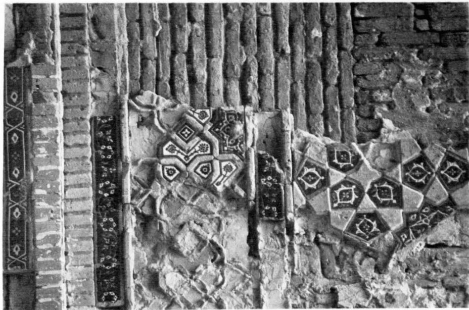
Pl. VIIb. Detail of revetment of west aivān.
