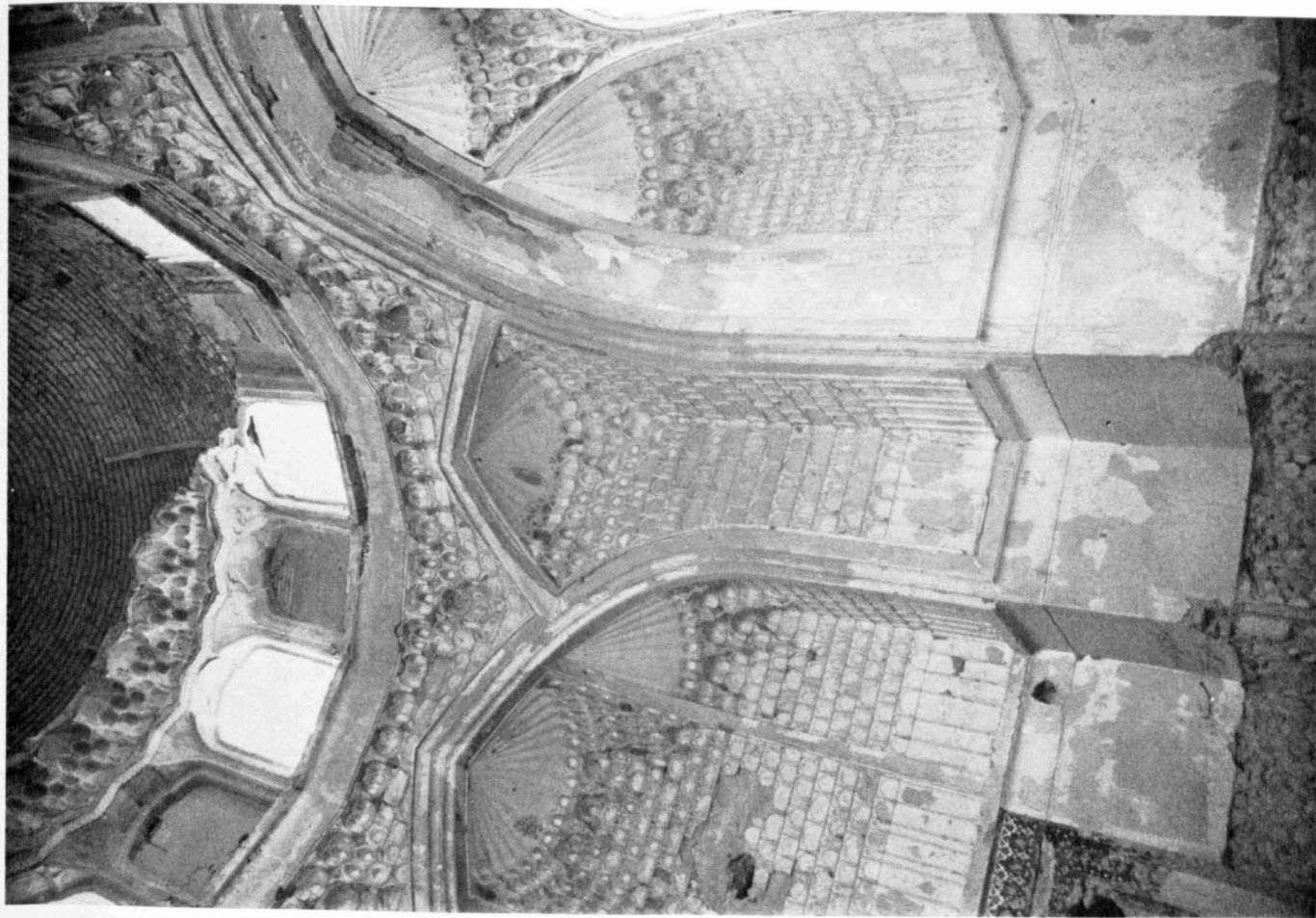
Pl. IIIb. Mosque, north-west corner.
