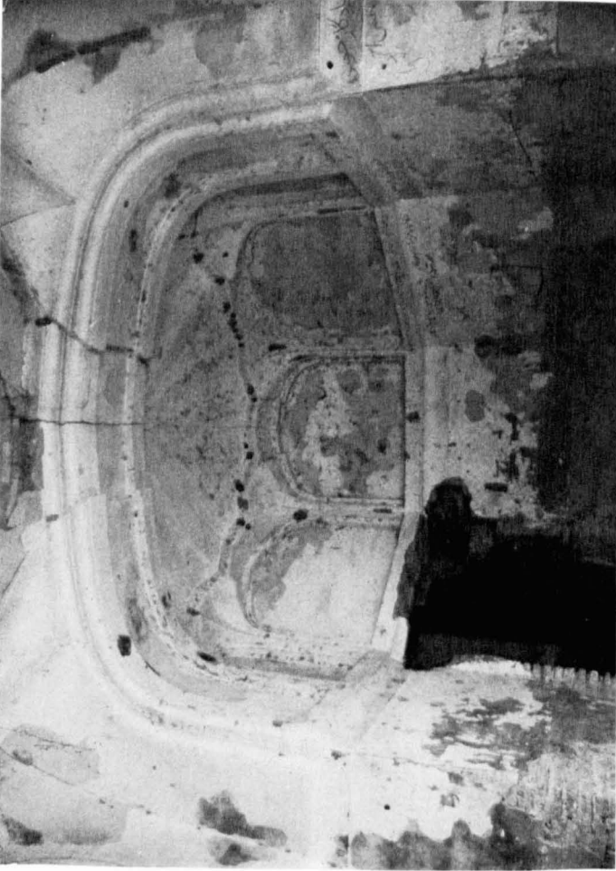
Pl. VIa. North-east lower domed room, east recess.
