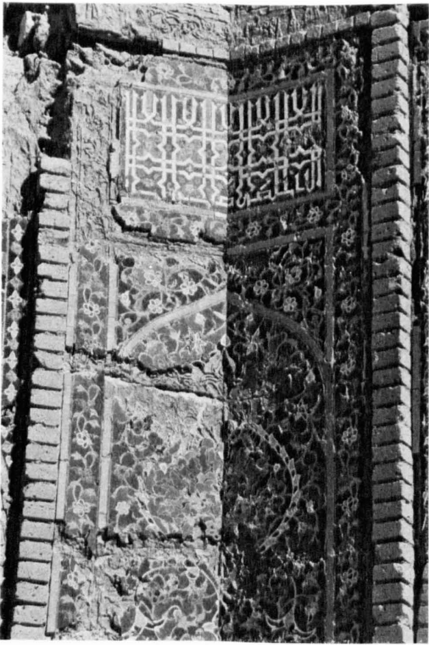
Pl. VIIIa. Panel of mosaic-faience on bevelled corner of courtyard.
