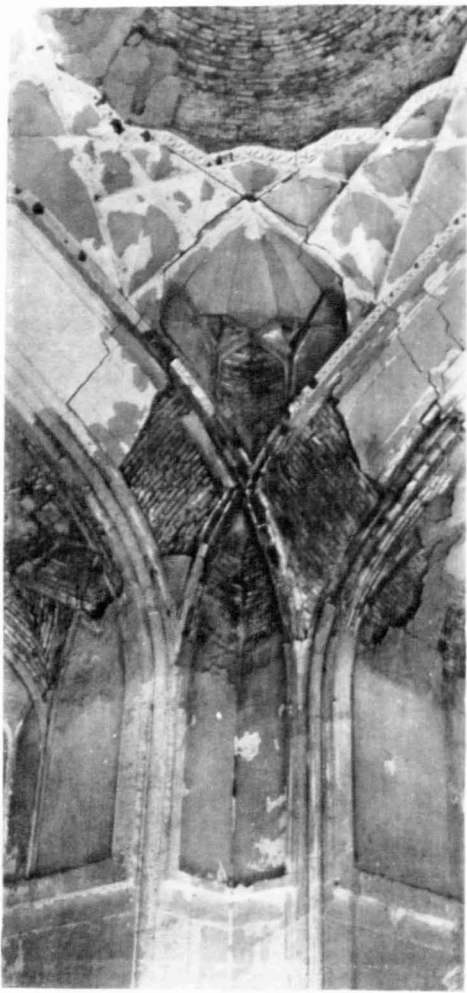
Pl. VIa. Turbat-i Jām, New Mosque: vaulting of sanctuary (photograph courtesy of The Asia Institute Archives, Shiraz).
