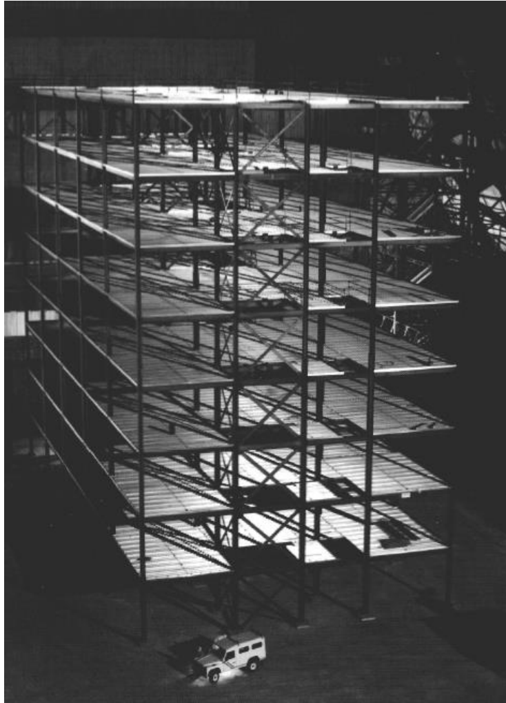
Figure 2.7. Cardington test structure (British Steel,1999)
