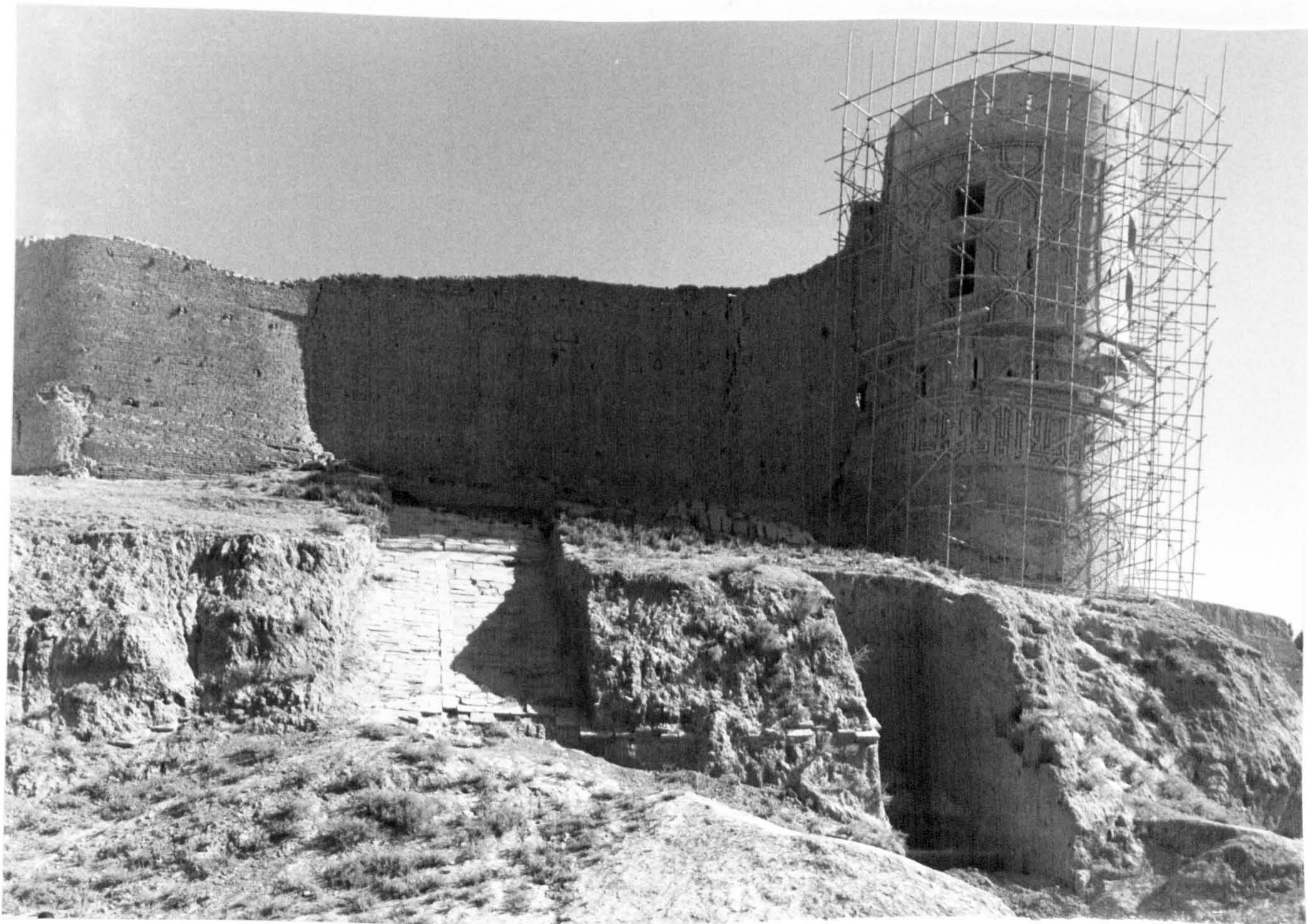
1) Herat: Citadel, NW tower: general view
