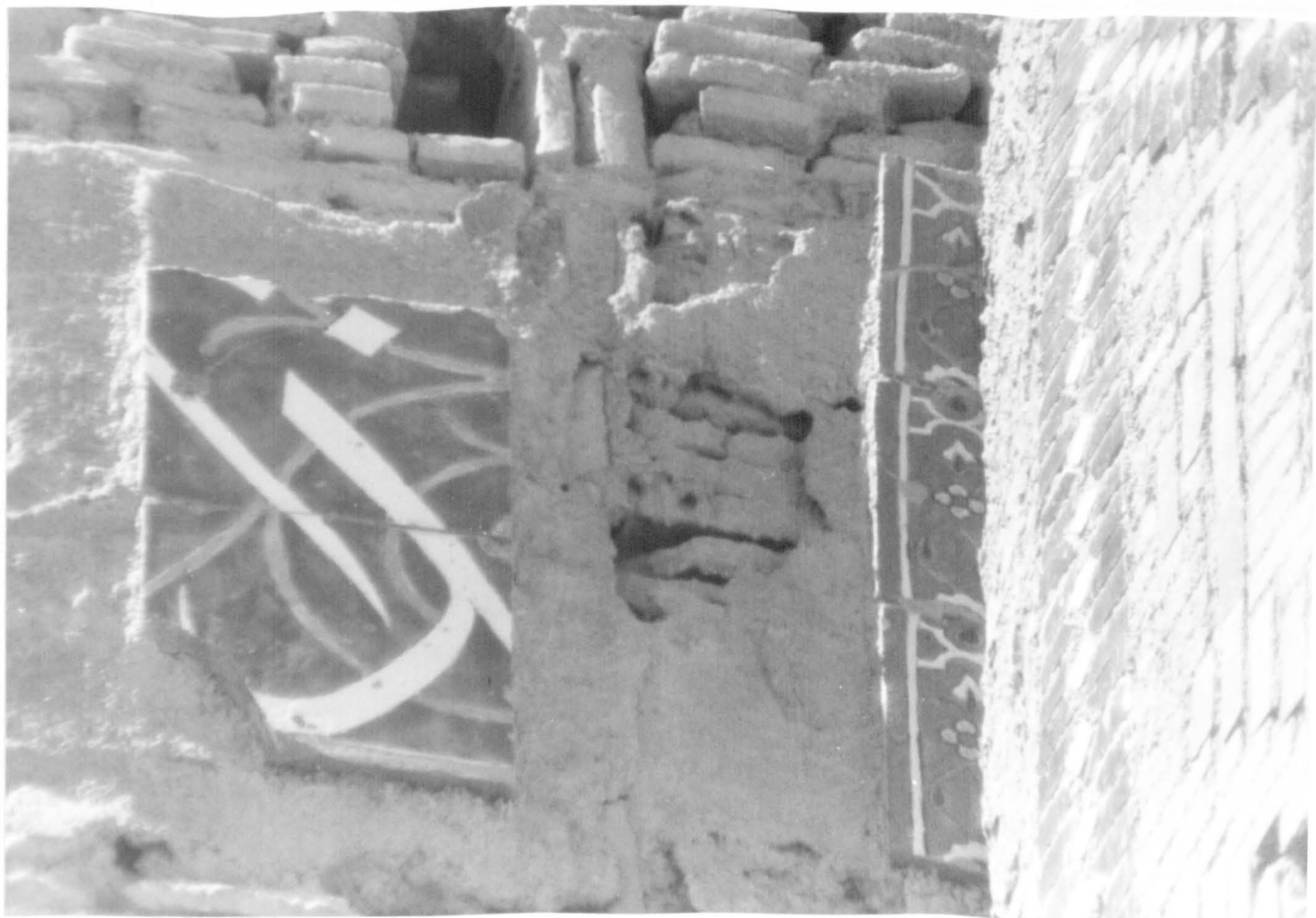
4) Herat: Citadel, wall beside NW tower: cuerda seca tiles
