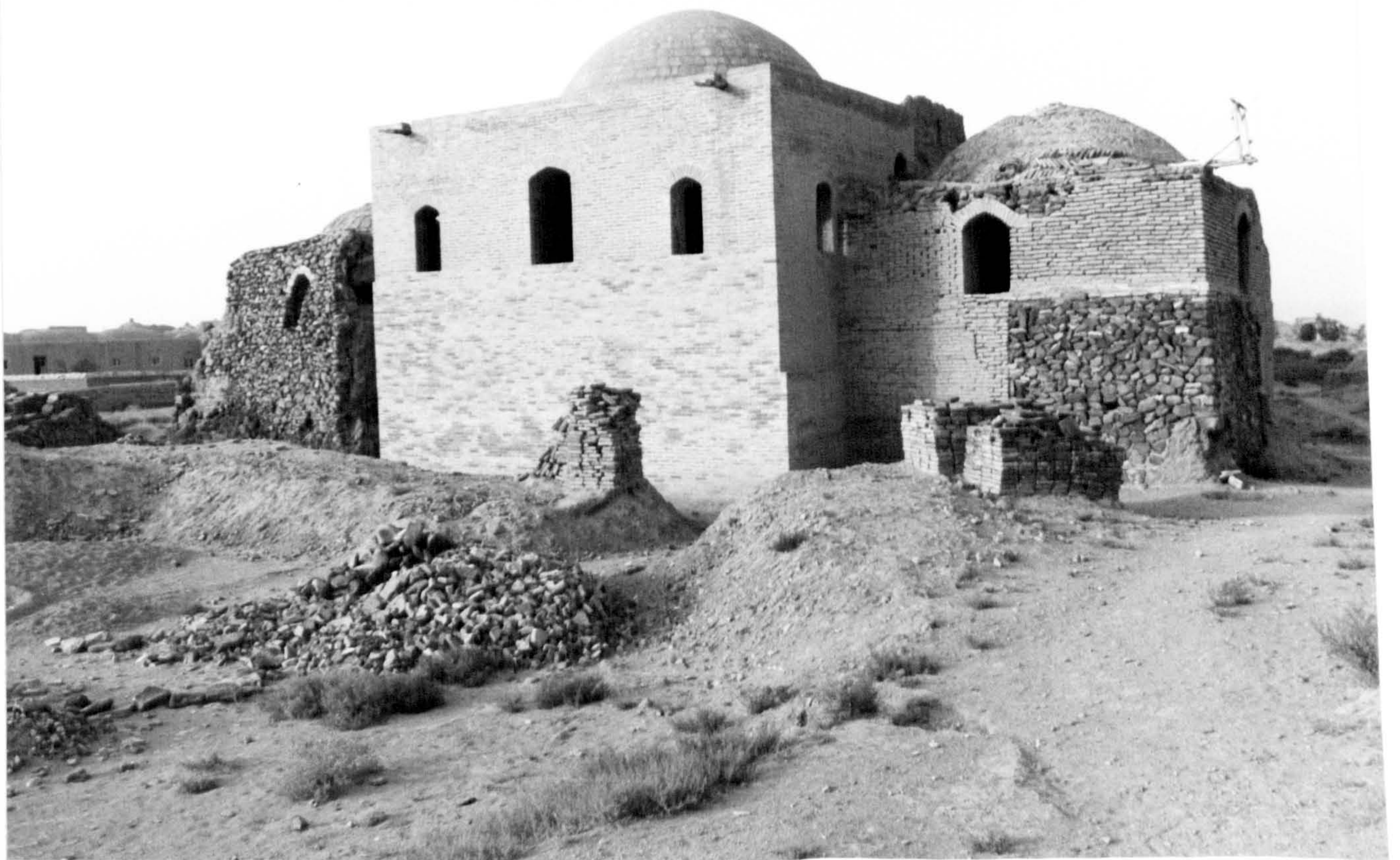
24) Hindvālān: Masjid-i Jami c , exterior: general view, from rear
