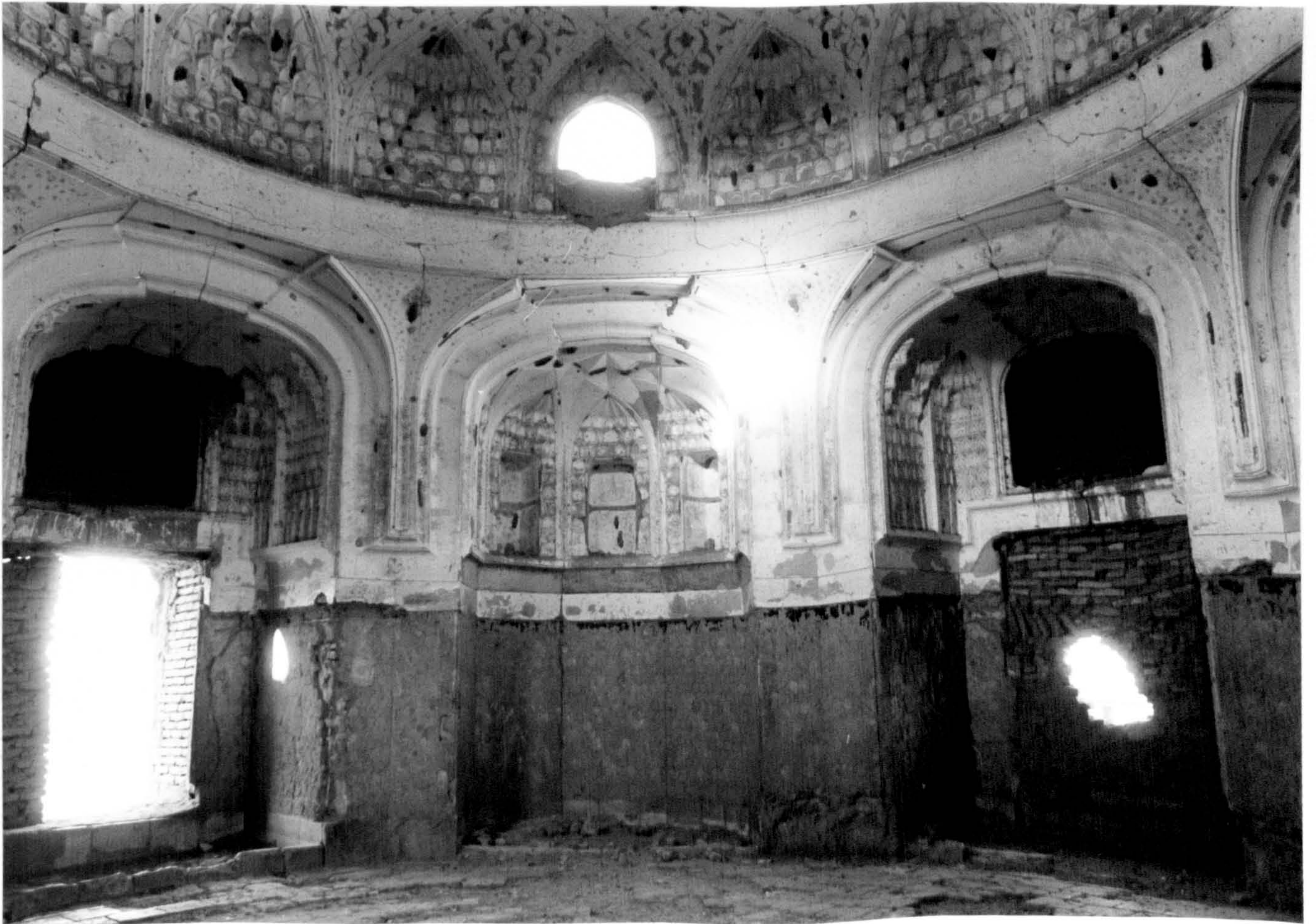
115) Kuhsān: Madrasa of Tūmān Āghā, interior: dome chamber, general view
