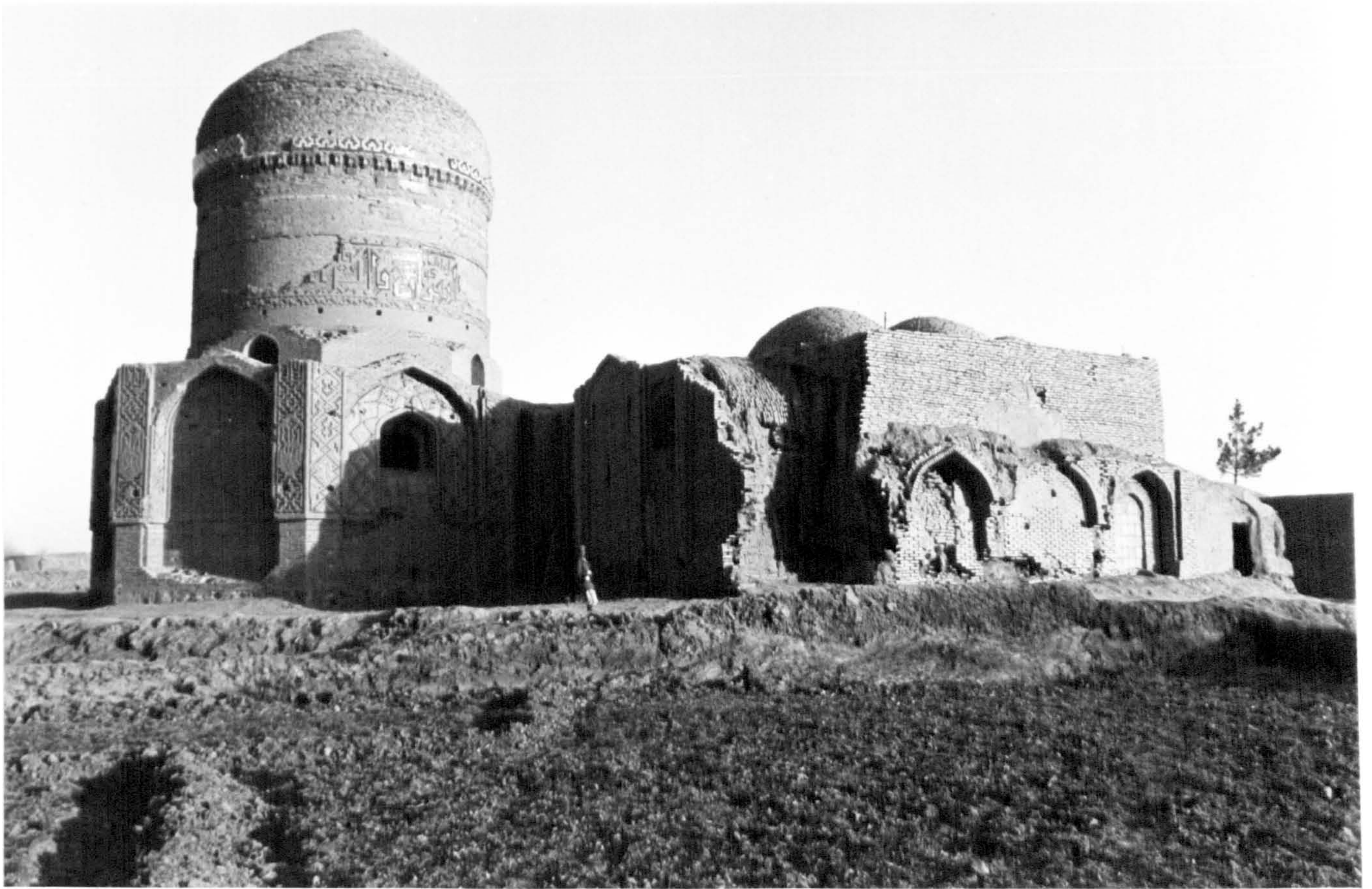
112) Kuhsān: Madrasa of Tūmān Āghā, exterior: from W
