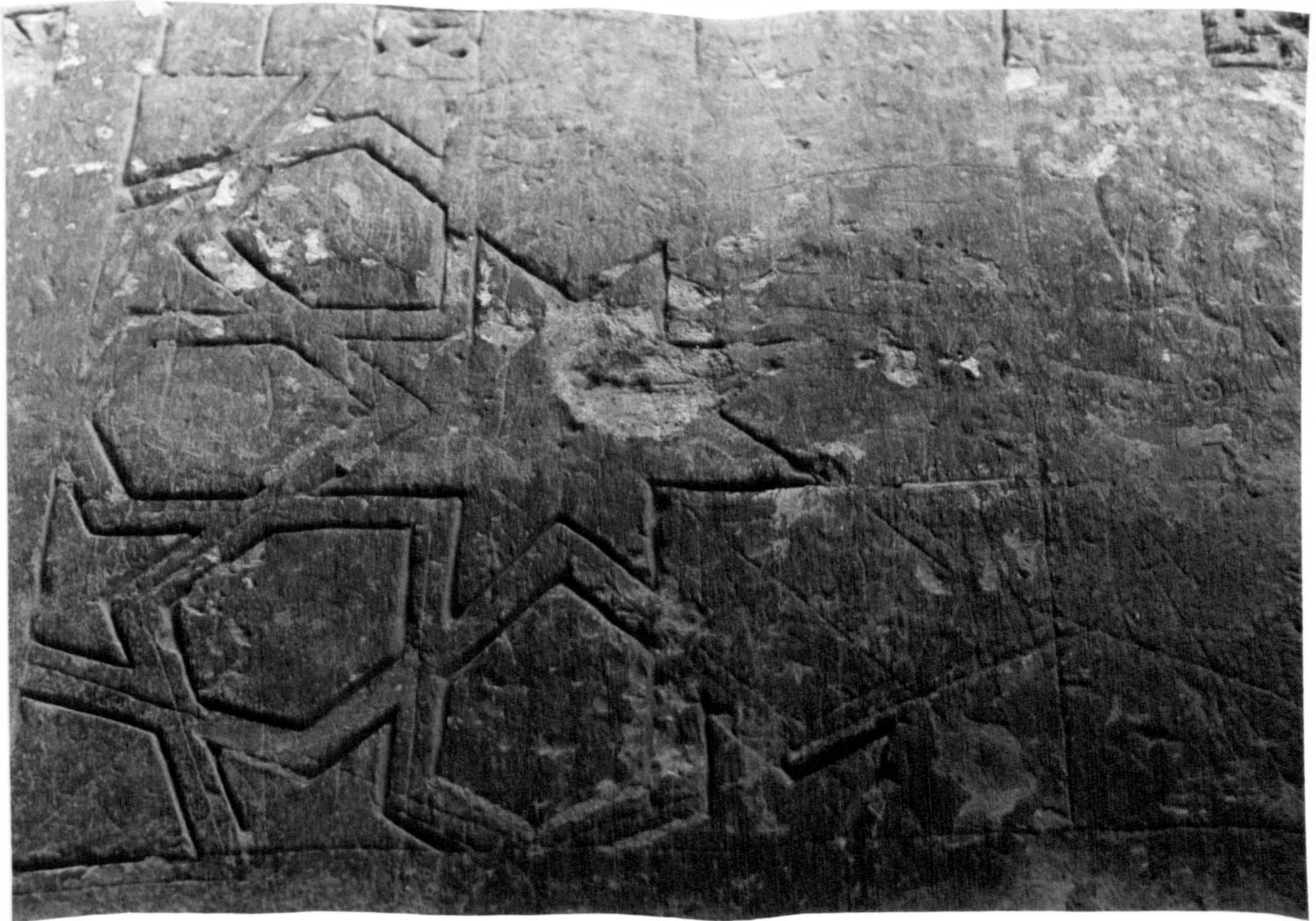
95) Mashhad: Madrasa Du Dar, courtyard facade, upper storey, S corner, setting up of stucco pattern
