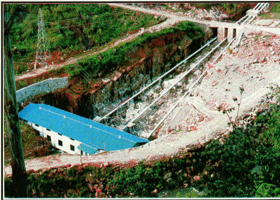
Figure 4.7: Site under construction at Dickoya, 1995
