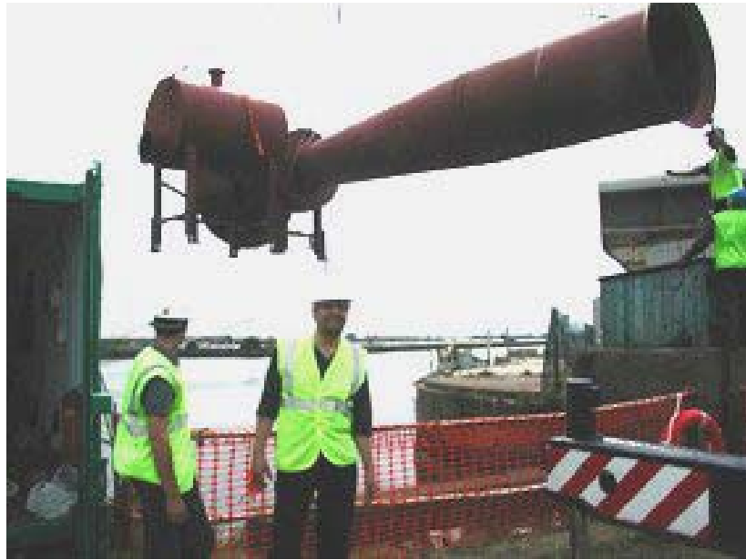
Figure 1.8: Primary circuit demonstrator of Rochester venturi being installed [32]
