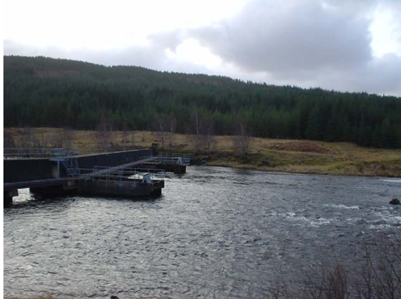
Figure 4.10: River Garry and dam
