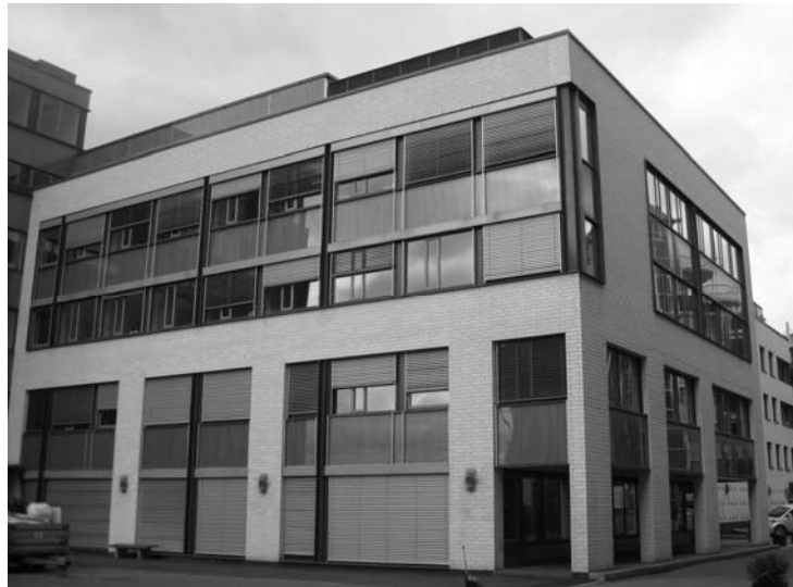
Figure 82: Building A: North facade
