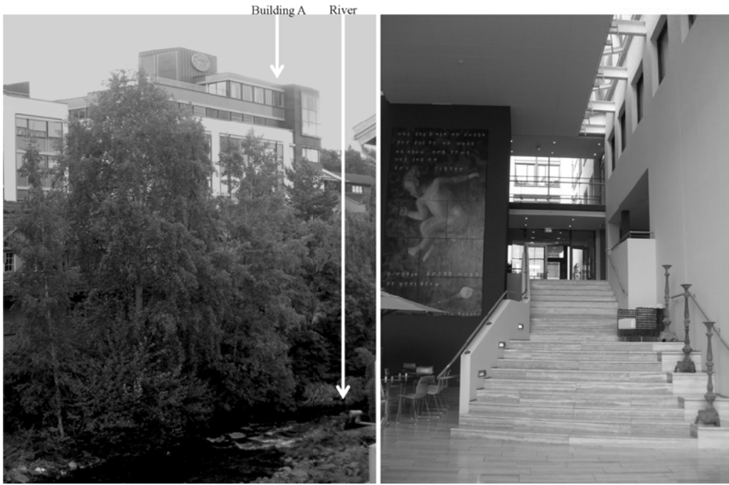
Figure 85: Building A: South façade and the main entrance
