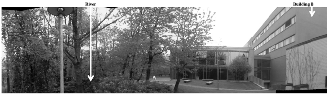
Figure 98: Building B: West façade
