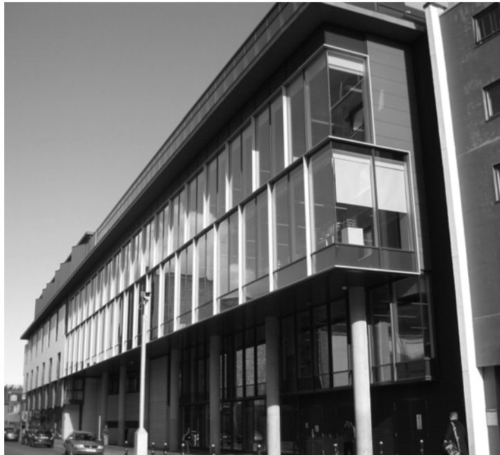
Figure 132: Building D: North façade
