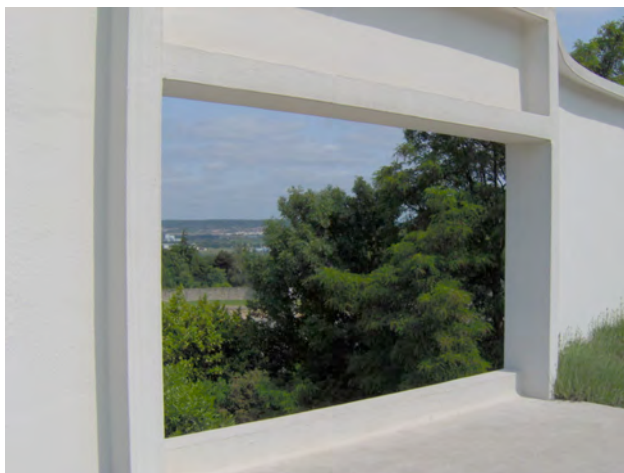
4.17 Villa Savoye, opening in roof garden wall
