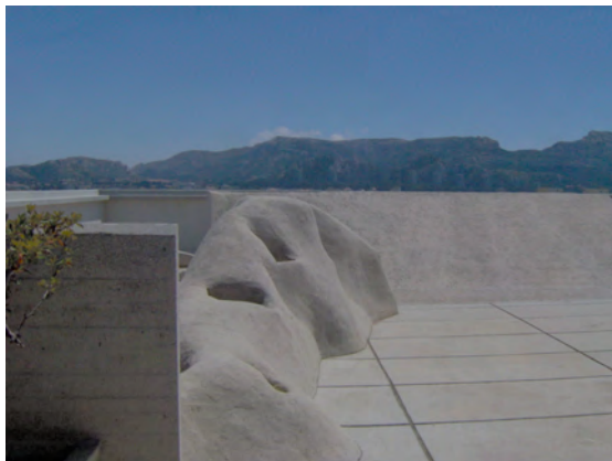
3.3 View across roof wall and concrete rocks
