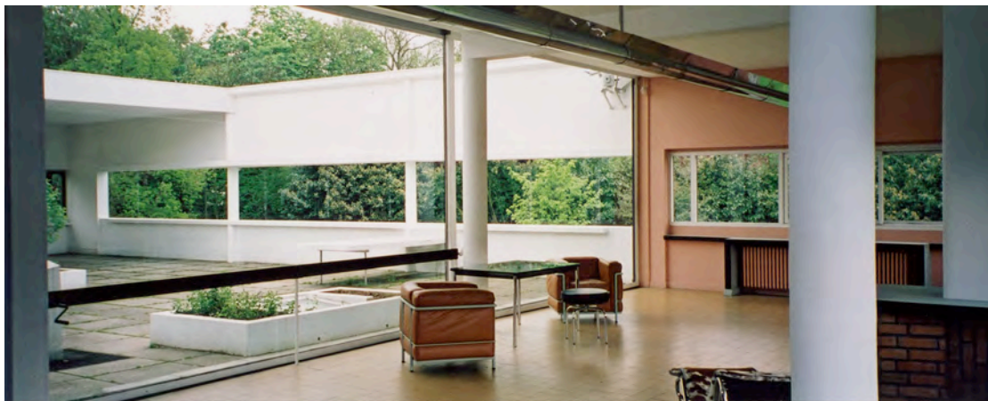
4.16 Villa Savoye, salon and terrace garden showing open and glazed strip windows
