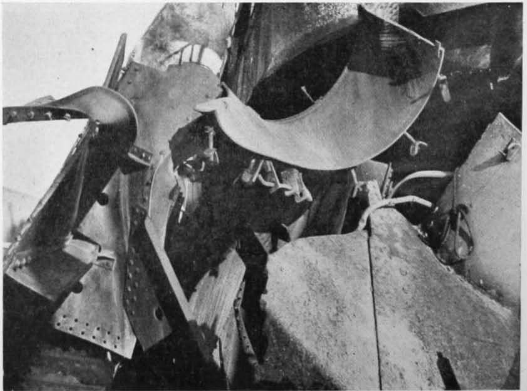
PLATE XI. Second view No. 4 wing tank—deck plates, main hatch combing, ullage chamber and plug.
