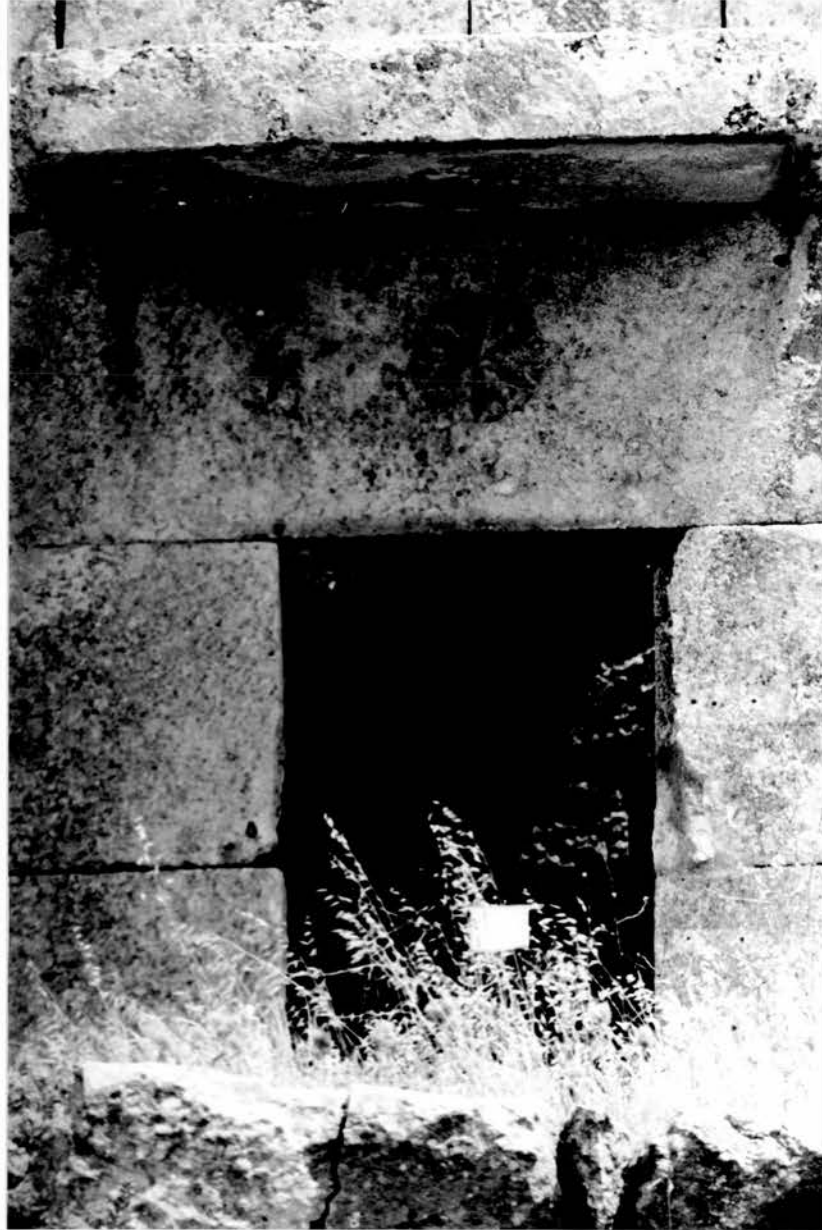
7. Window lintel, Rifādī.
