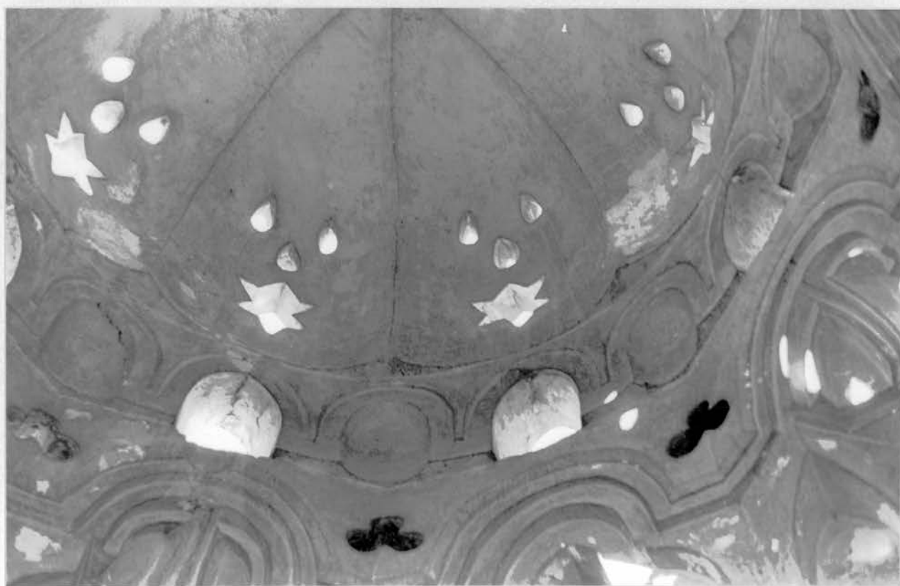
177. Interior of the dome, Fatimid mausoleum at Qūs.
