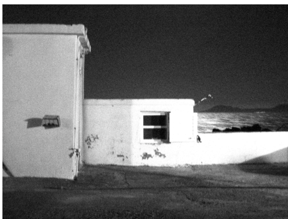
Figure 31: An extension to a small house
