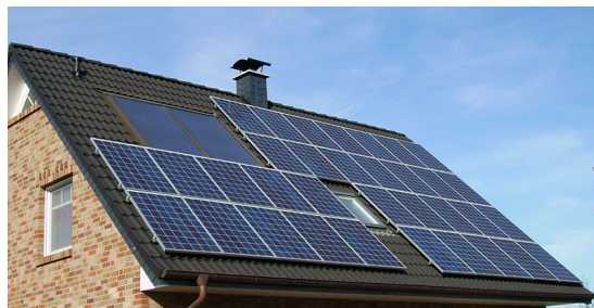
Figure 2.3: Solar panels on the roof of a house which turn light directly into electricity.
