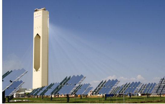
Figure 2.2: Seville's solar power tower, Spain. Light is focussed on the central tower and used to create super-heated steam.
