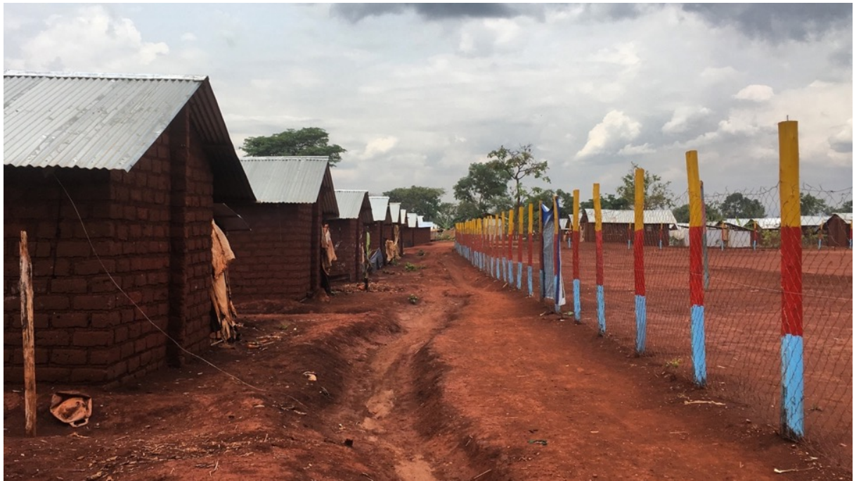
Figure 8: Houses on Burundian side of Nyarugusu camp. Credit: Boeyink 2017
