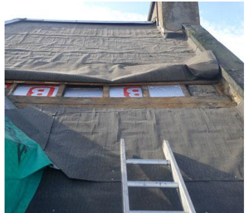
Figure 34 Rigid insulation on site (Edinburgh 2013)
