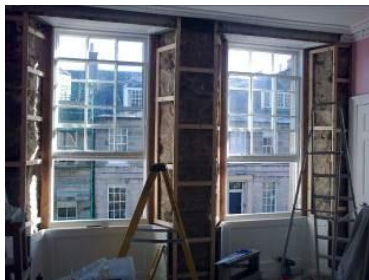
Figure 18 Framing for Insulation
