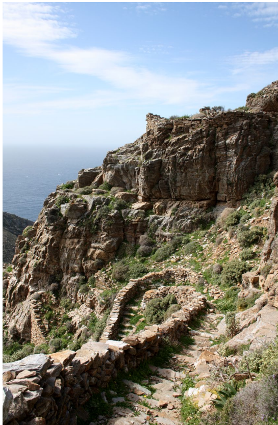
Fig. 91. The staircase to the upper level
