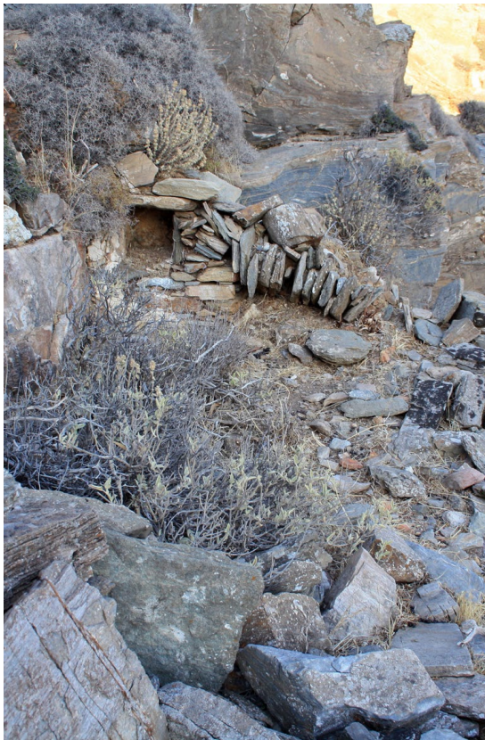
Fig. 79. The collapsed apse of ch2
