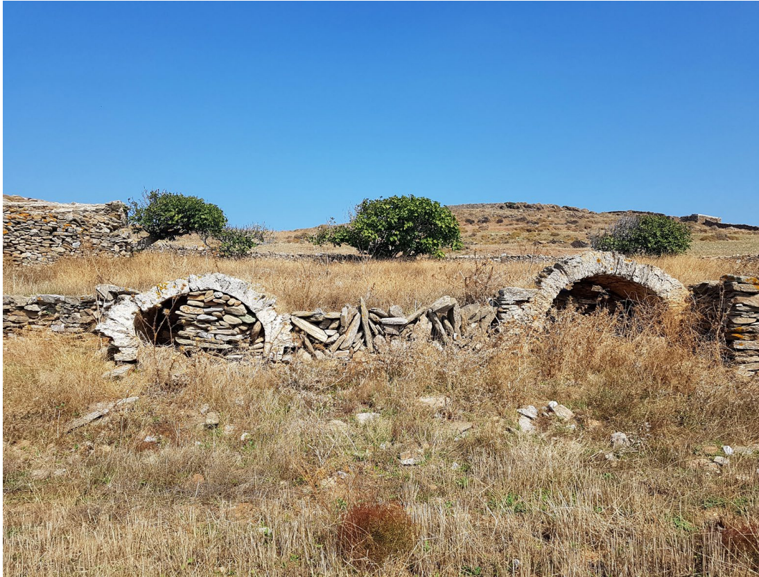
Fig. 76. The arches, view from the south
