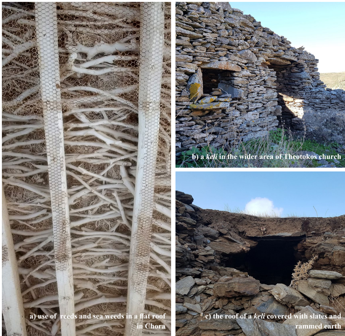
Fig. 158. Local building practices applied in the settlements and the countryside of Kythnos
