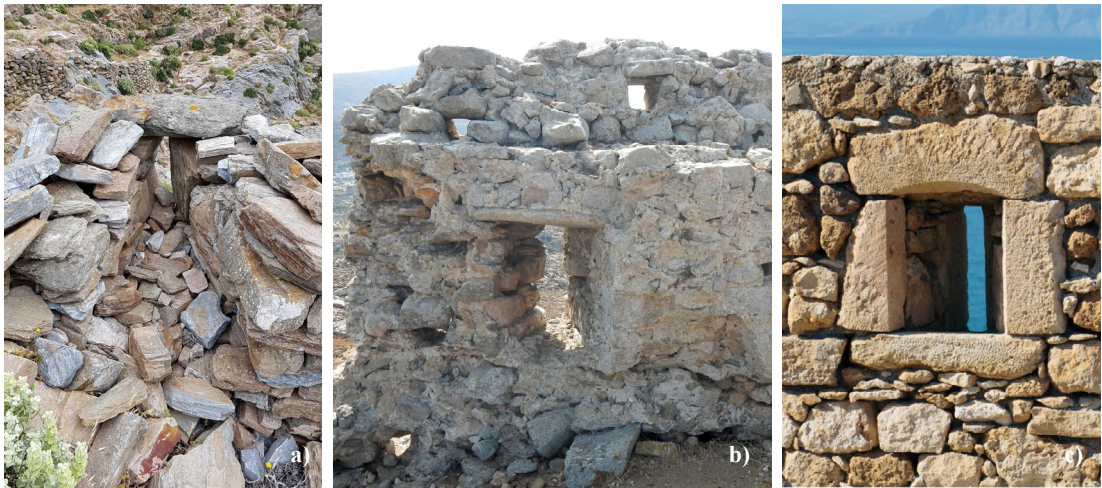
Fig. 84. Loopholes in Oria (a), the Apano Kastro in Naxos (b) and the Fortezza in Rethymno (c)
