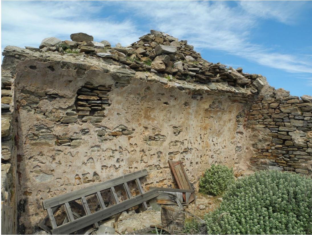
Fig. 128. Cistern 2, interior south-west view
