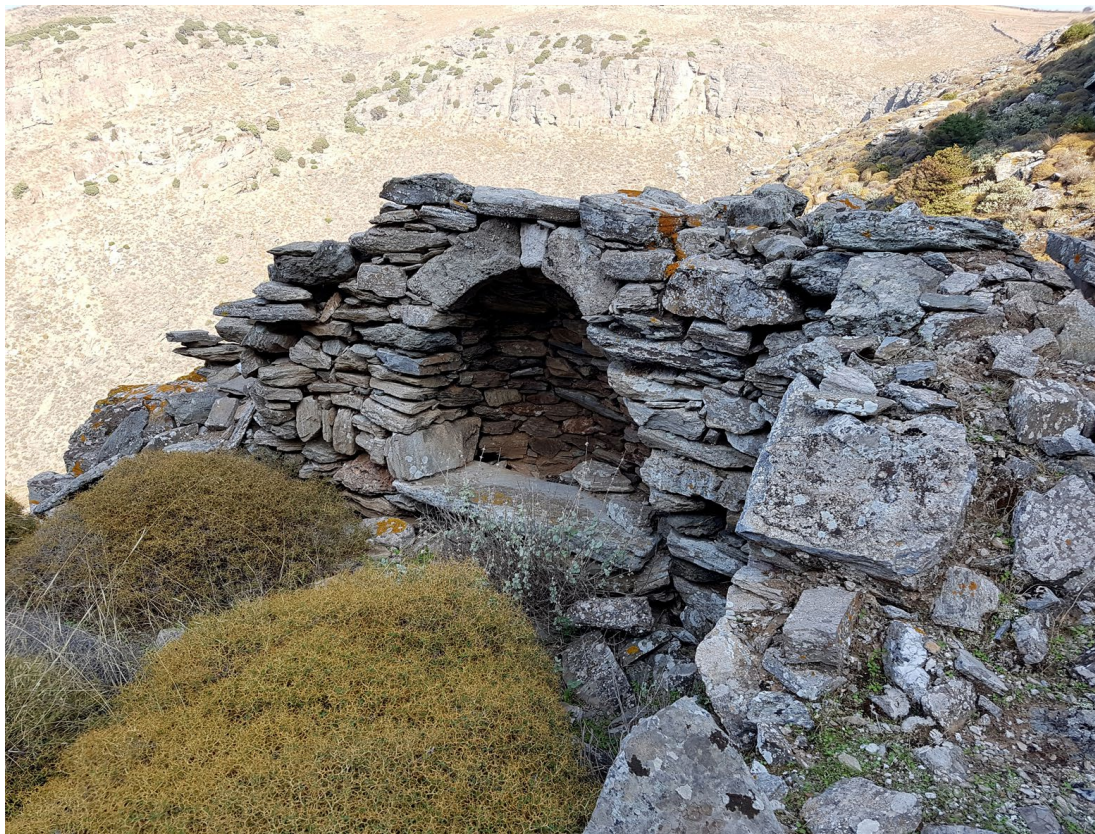
Fig. 161. The sanctuary apse of ch17
