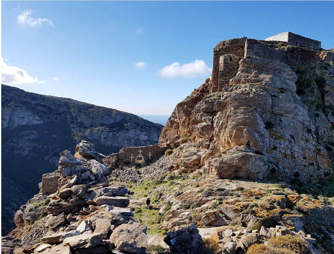
Fig. 81. The south-east gate as seen from the watchtower (9)
