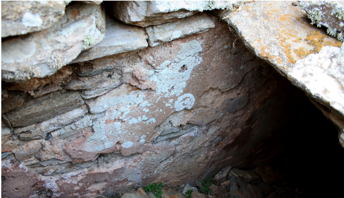
Fig. 116. Hydraulic mortar ( kourasani ) applied to the interior of c4
