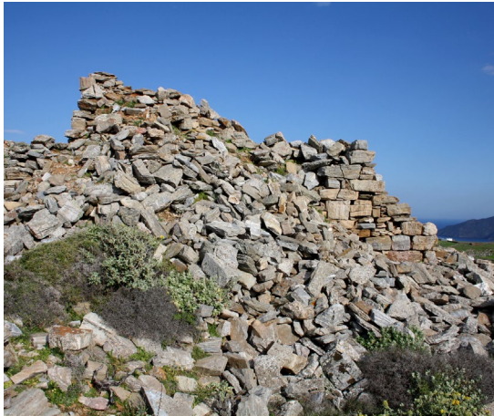
Fig. 102. Building 33 from the west
