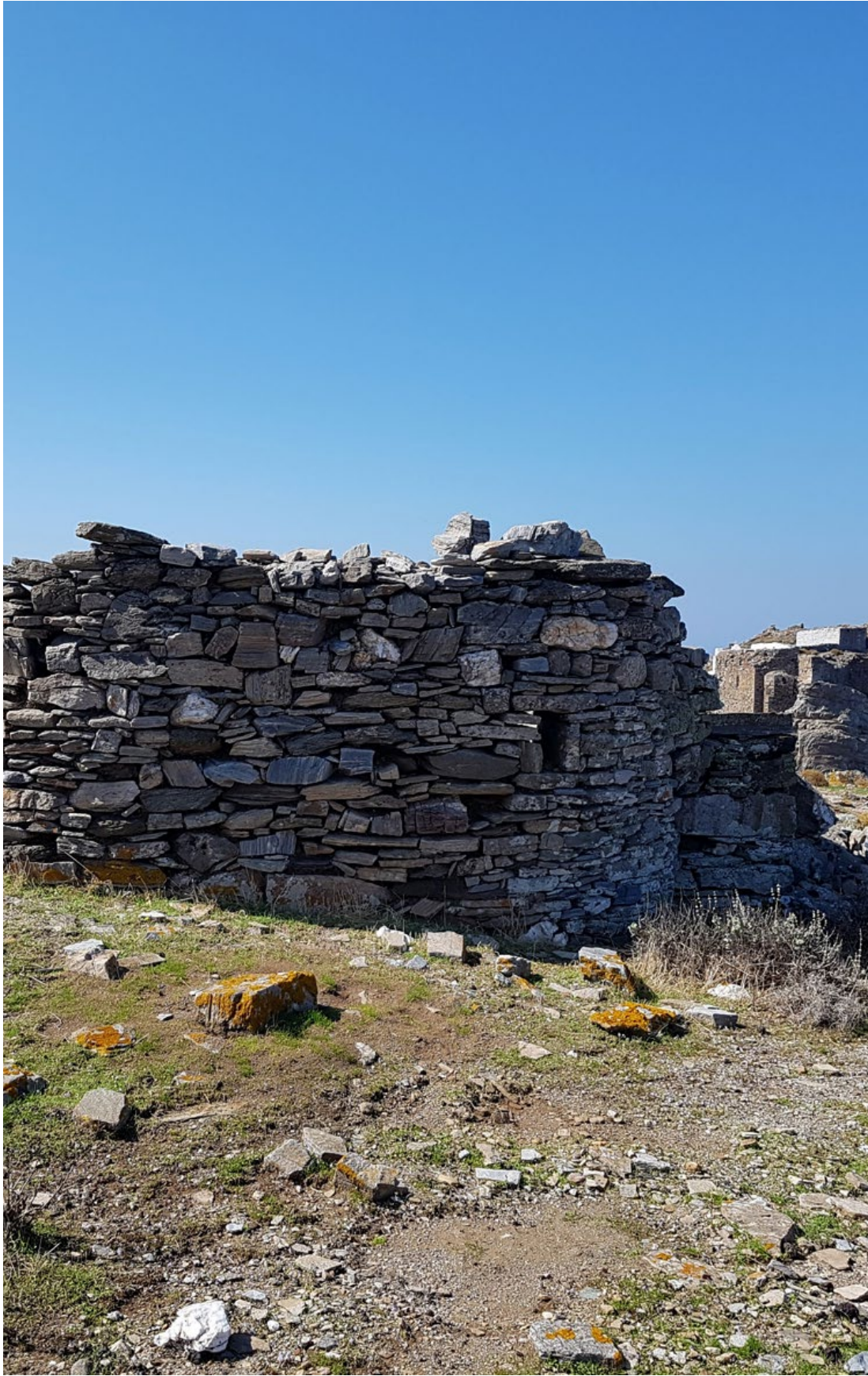
Fig. 159. The double-apsed church (ch19) of the east settlement, east elevation
