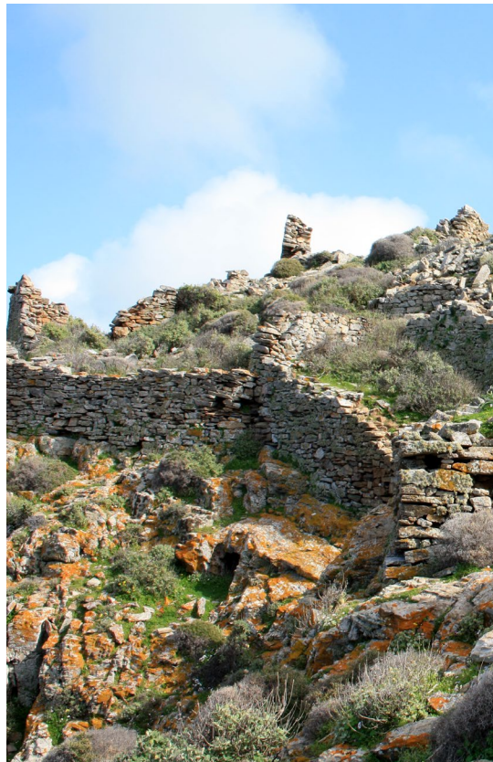
Fig. 92. The northern flank of the inner wall
