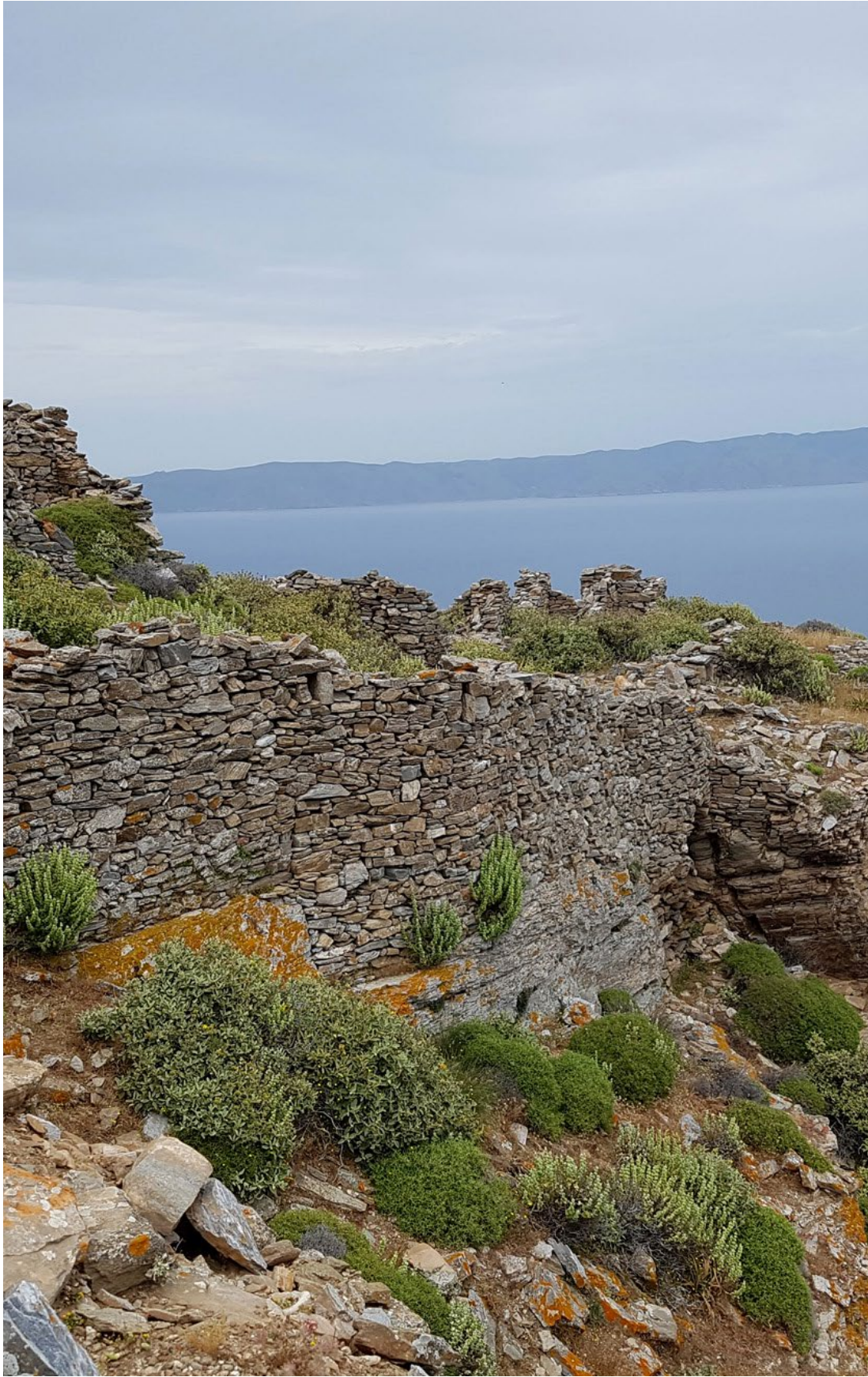
Fig. 93. The loopholes of the inner wall (northern flank)
