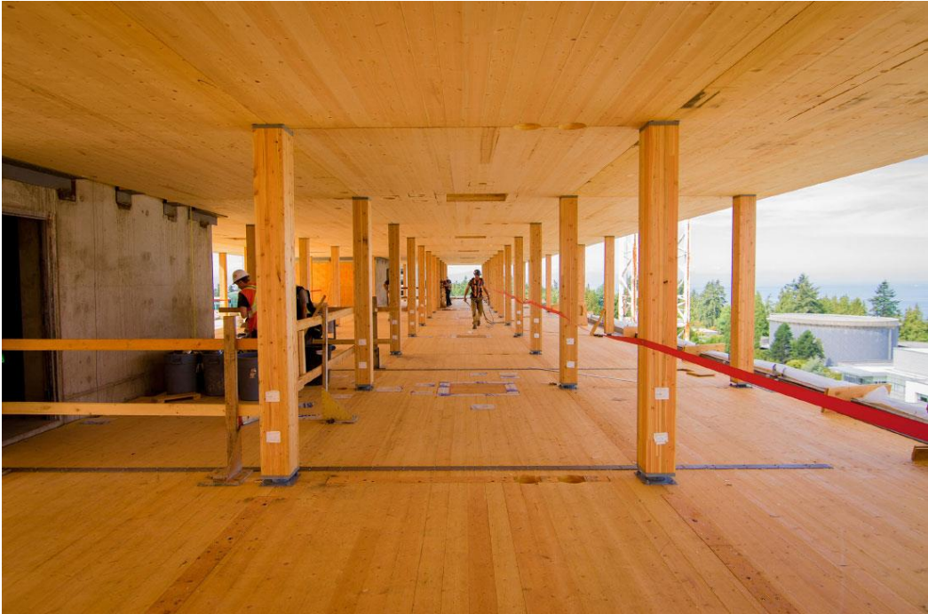
Figure 2.5. The interior of Brock Commons under construction [33].
